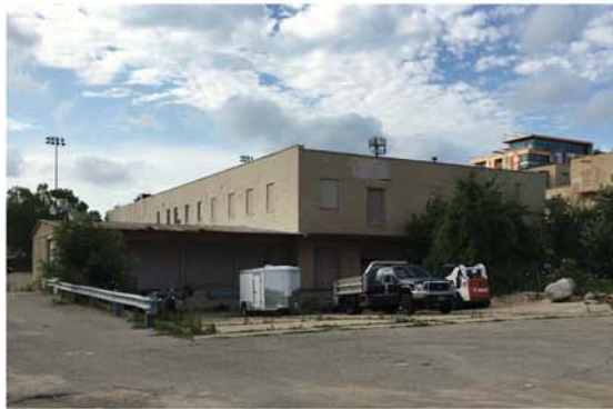
To be Demolished - 925 East Washington Ave. View from East Main Street
