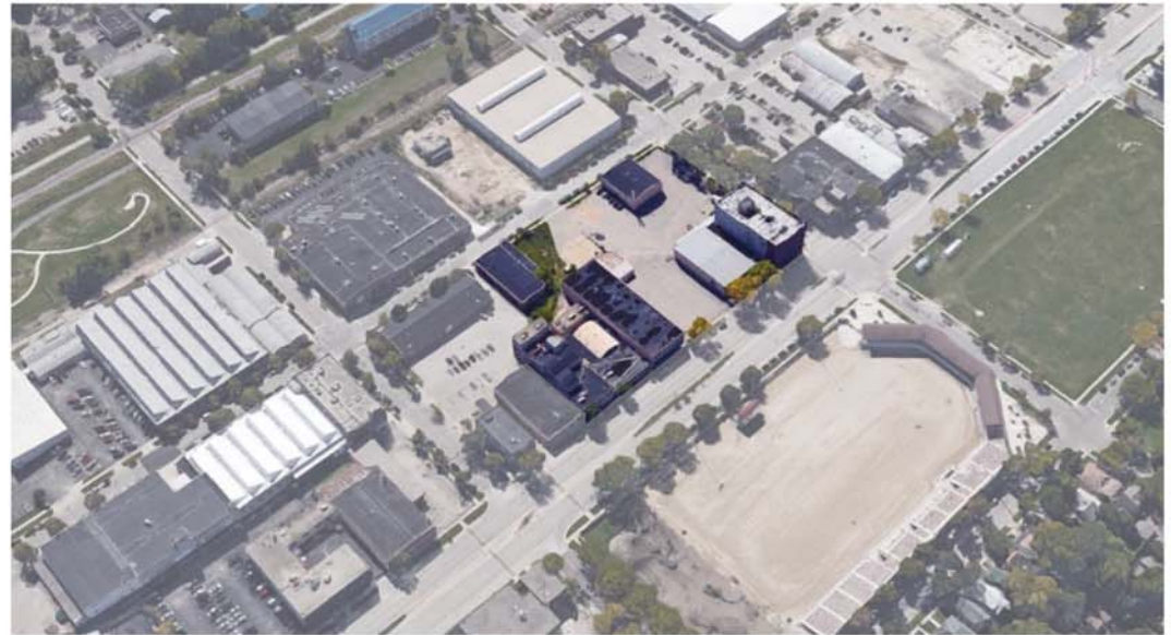
View from North
