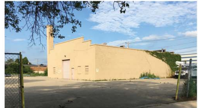
To be Demolished - 910 East Main Street, View from South Paterson Street
