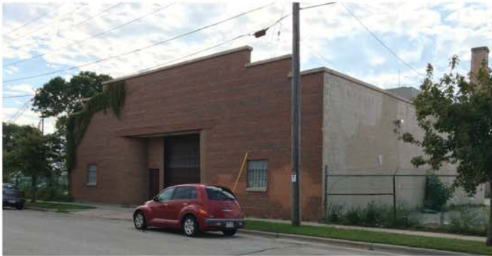
To be Demolished - 910 East Main Street
