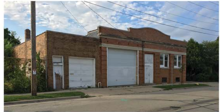
To be Demolished - 922, 924 East Main Street
