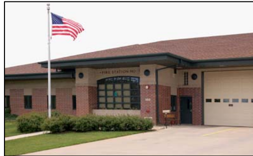
Fire Station 7 provides fire and safety protection for the area. A new ambulance would improve response time for emergencies.
