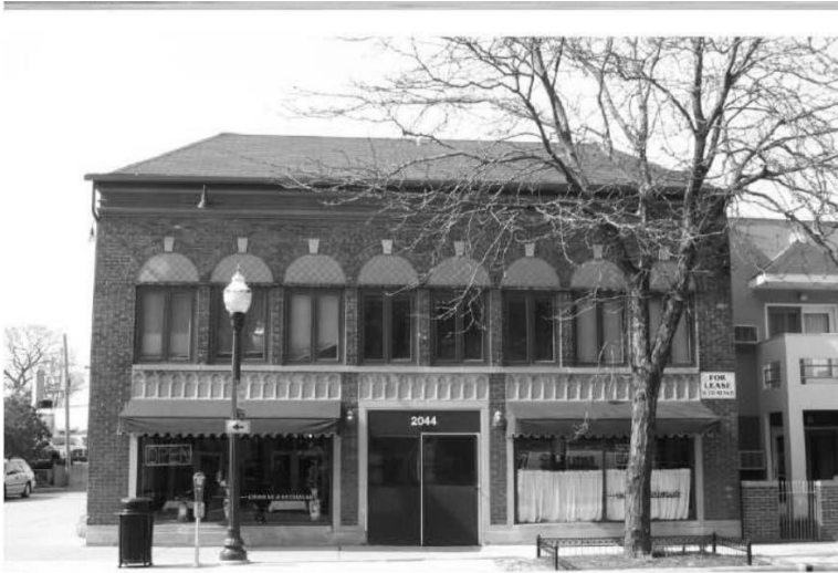
Figure K14: Typical Commercial Block Building Photo 2, MGO 28.173
