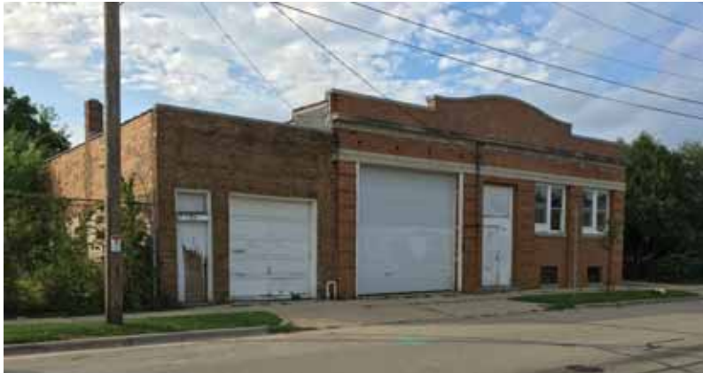
924 East Main St - To be Demolished
