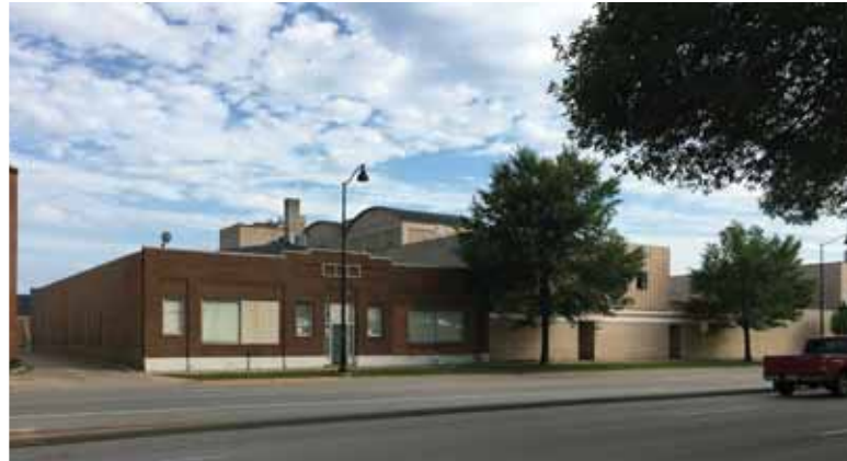
945 East Washington Ave - To be Demolished
