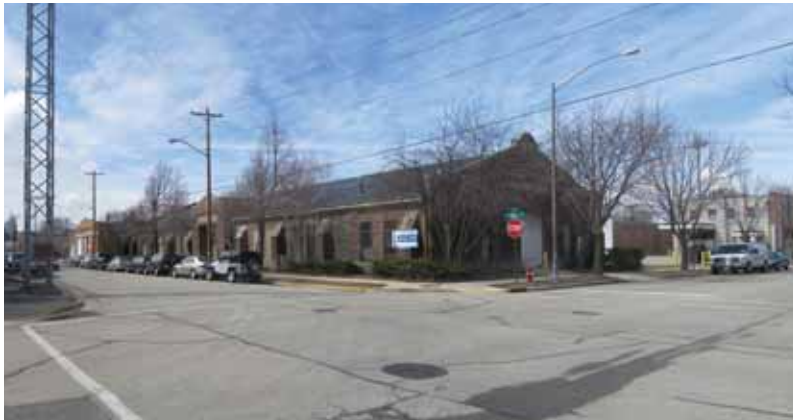
945 East Main St Telephone Building - To Remain
