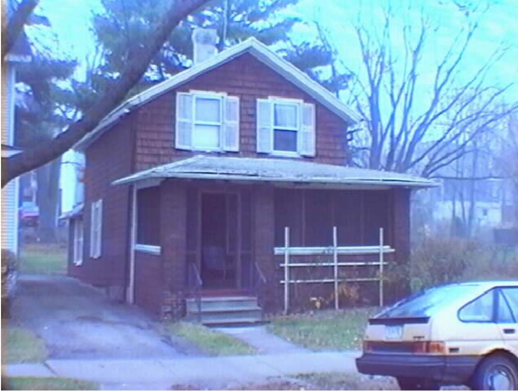
620 East Johnson Street
