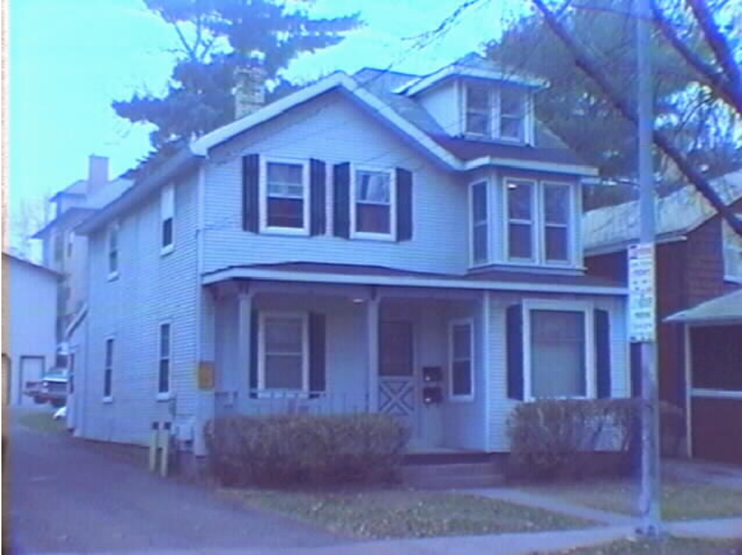
618 East Johnson Street
