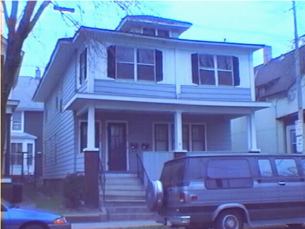
608 East Johnson Street
