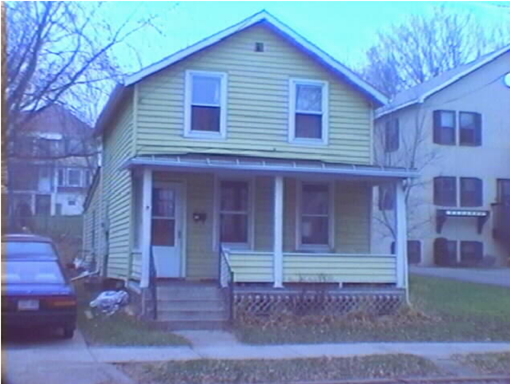
626 East Johnson Street
