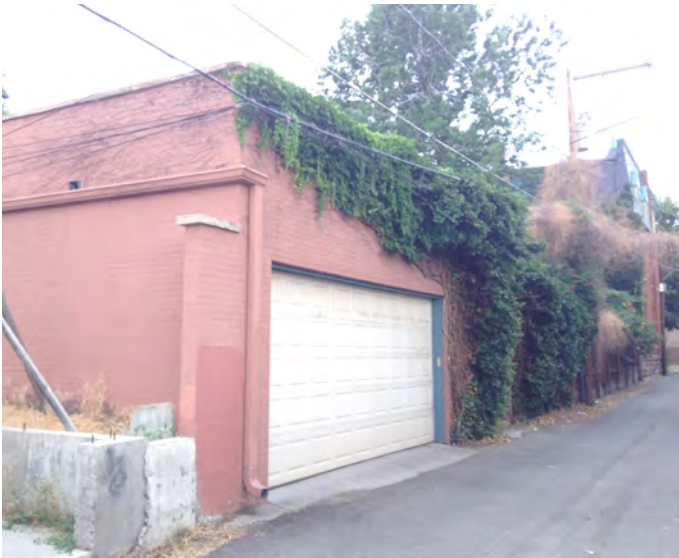
16. Carriage house structures within Clements Historic District. Accessed from the alleyway, one-story in height and of brick construction with a flat roof.
