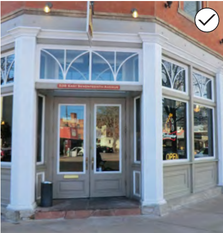
76. Orient a building's entrance to be consistent with the established historic pattern of the surrounding context/block. Typically, the primary entrance faces the street.
