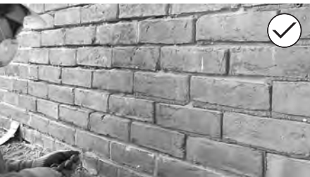
9. Re-point deteriorated masonry mortar joints.
