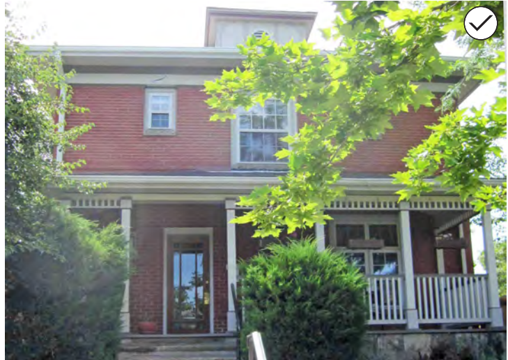
34. Maintain and enhance the energy-saving features of the original structure. The porch on this house helps to buffer temperature swings.
