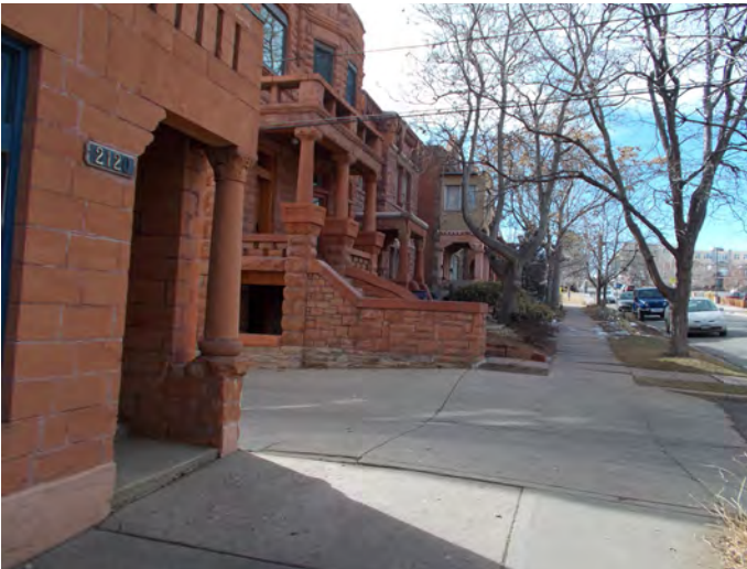
1. Streetscape of Stonemen's Row. Note the uniform setback with projecting stone stoops, the small front yard, and old growth trees in the buffer lawn.
