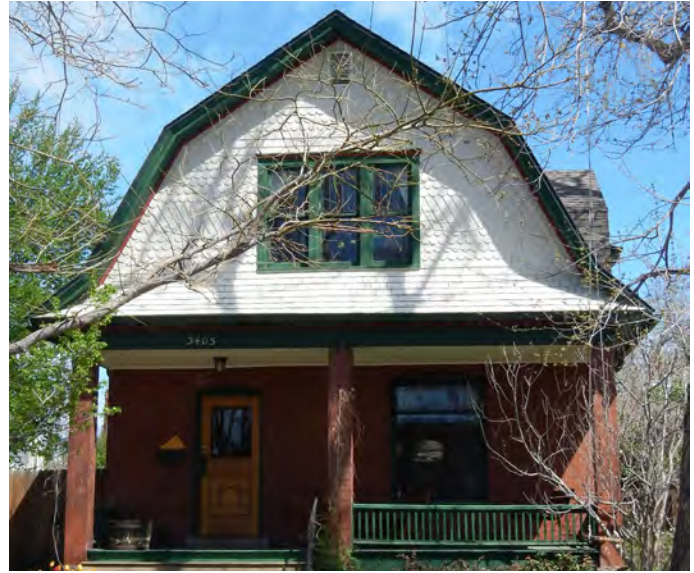
6. Queen Ann style structure with a forward facing gambrel roof. Note the masonry porch columns, the triple window bay, and fish scale shingles in the forward facing gable.
