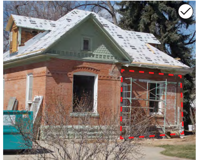
56. Minimize damage to historic structures when demolishing non-contributing additions or features. A non-historic addition was removed from the façade illustrated at left, allowing the original exterior to be repaired. A non-historic porch was carefully removed from the front of the house illustrated at right.
