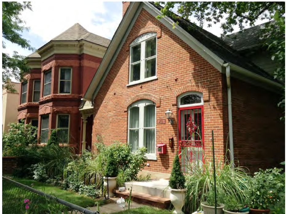
1. Streetscape within Curtis Park with eclectic architecture that characterizes the district. Note the simplified Queen Anne cottage in the foreground with orange brick façade in contrast with the elaborate, large Italianate duplex structure in the background with brick façade, stone stringcourses, window headers and sills.
