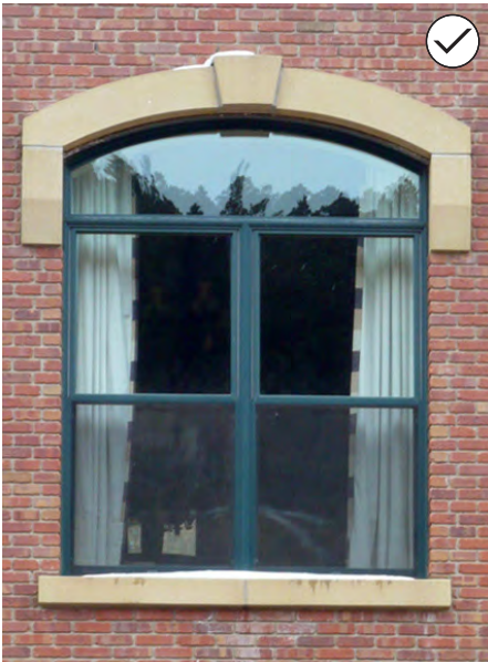
20. If windows are missing, use a replacement design that matches the style, size, and material of the original windows.
