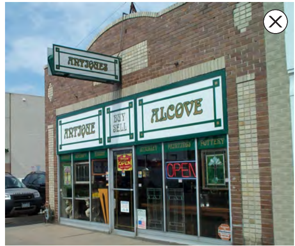
142. Do not remove, alter, cover or visually obstruct historic architectural features, such as windows, columns or decorative horizontal banding.
