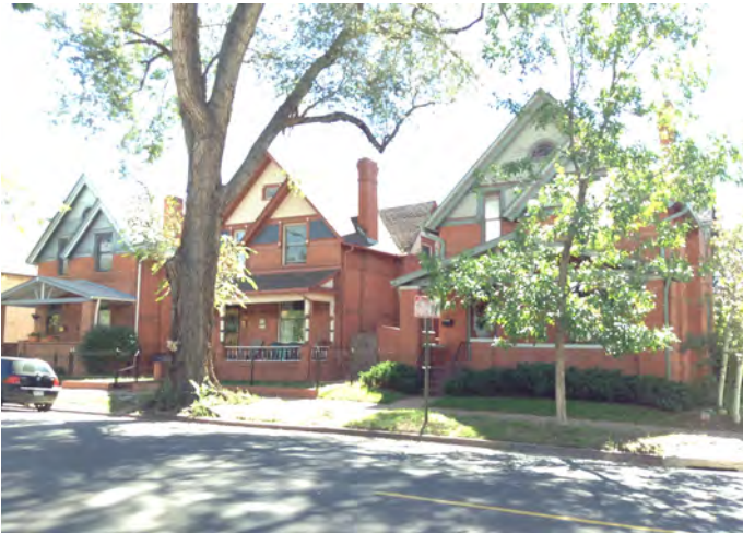
1. Street view of Queen Anne style houses within the district. Note the forward facing gables, one story porches with shed and gable roofs, the large windows, asymmetrical appearance of the front façade and overall architectural harmony of this block. Middle porch original; two flanking early 20th century addition – historic but not original.
