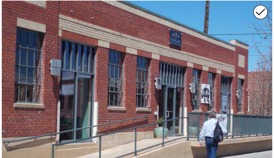
58. Select uses that are compatible with the original historic character of the building.
