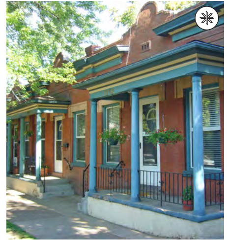
40. Maintain the overall composition of a porch when replacing missing components and decorative features (i.e., when replacing balusters, match the original proportions and spacing). If, for example, this porch originally had a wood balustrade, a wood design would be preferred. If not, a simple metal design such as this could be appropriate, in that it retains one's ability to perceive the visual prominence of the columns.
