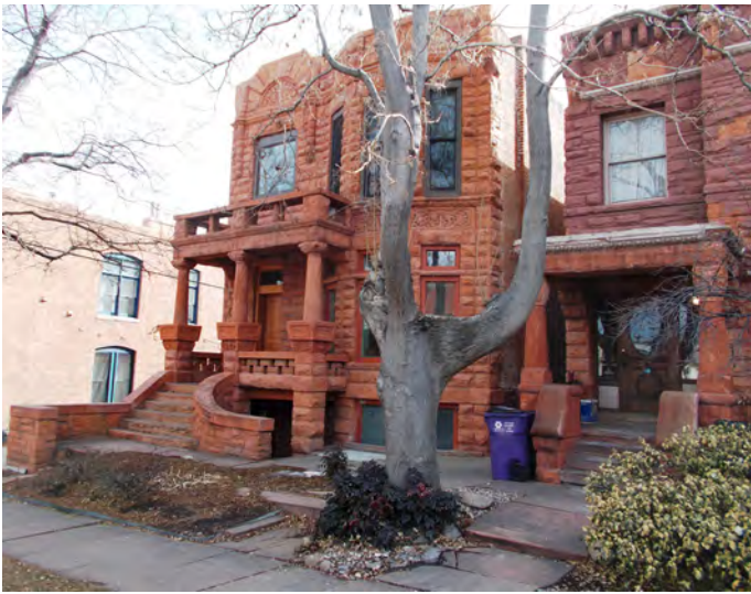
6. Streetscape of Stonemen's Row. Note the raised masonry porch forms on both these structures, with heavy Romanesque columns and detailing, the wing walls and the second-story balcony on the structure in the background and the one-story configuration of the porch in the foreground.
