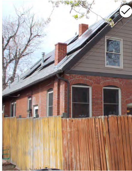
36. On a side-facing roof plane of a primary structure, minimize visual impacts by locating solar collectors on the rear 2/3 of the roof length. The collectors illustrated above do not minimize visual impacts because they are located on the front 1/3 of the roof length.
