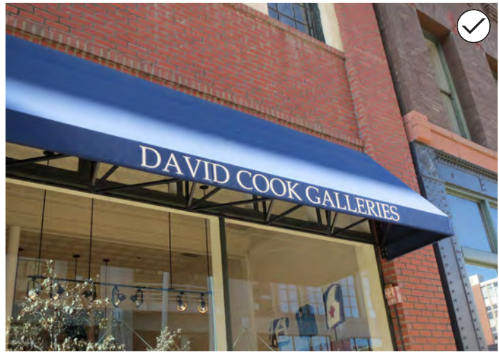
156. Use traditional triangular shaped awnings comprised of high quality canvas to frame a storefront window or door.
