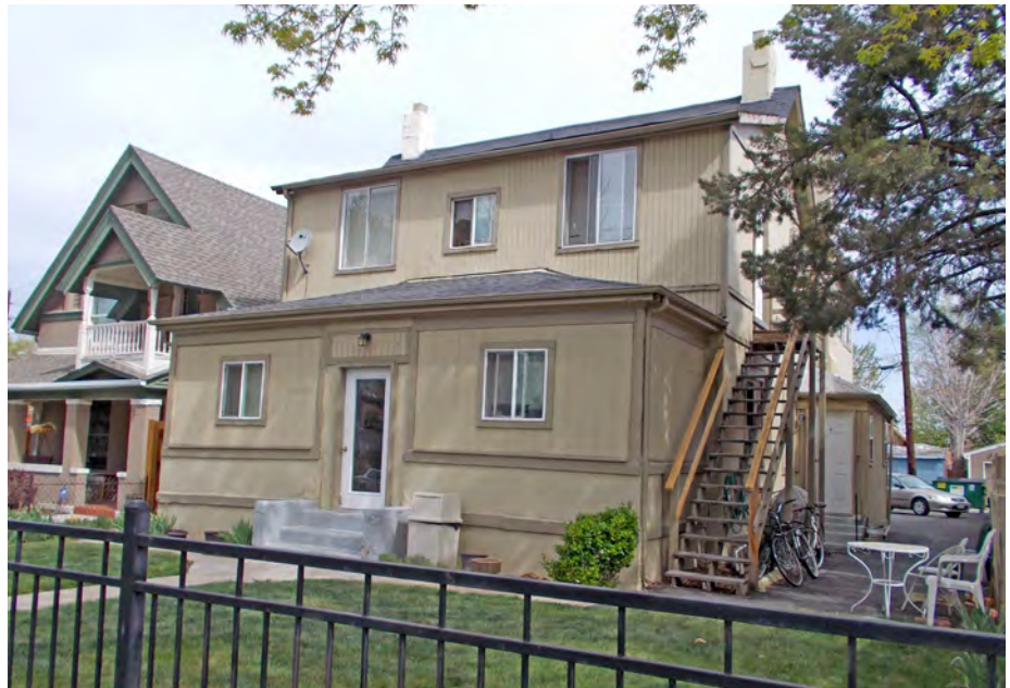
4. Non-contributing house in a historic district
