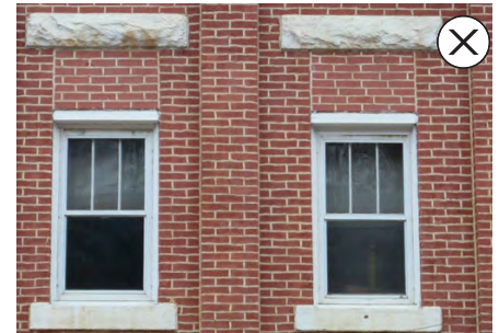
15. Do not reduce an original opening to accommodate a smaller window or door, or increase it to accommodate a larger one.
