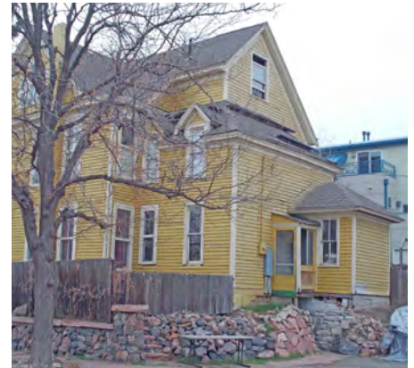
2. Contributing addition to a historic structure.
