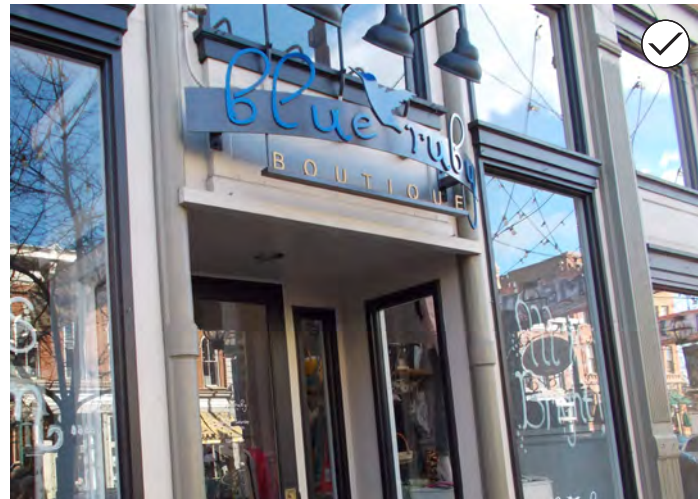
152. A slightly arched sign can still be considered a wall sign if it extends off the wall plane by 2 feet or less. This wall sign does not obstruct architectural details of the building.
