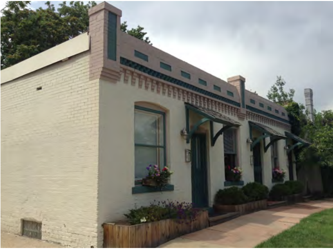
10. One-story multi-family Italianate dwelling facing onto a side street. Note the building mass aligns with the sidewalk, the decorative cornice, the segmental arched window and covered stoop entries.
