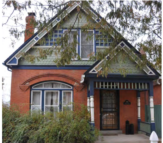
4. Queen Anne cottage. Note the decorative fish scale shingles and barge boards in the forward facing gable, the spindle columns and fretwork on the projecting front porch, the arched windows on the first floor with decorative jack arch and corbels.
