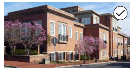
80. Use vertical and horizontal articulation techniques to reduce the apparent scale of a larger building mass.
