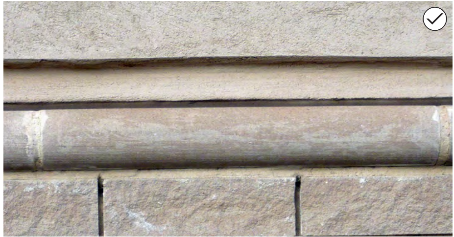
82. New materials that convey characteristics similar to historic materials may be considered if they have a similar appearance, size and shape to traditional materials, such as the cast stone illustrated above, which is detailed to convey a sense of authenticity.
