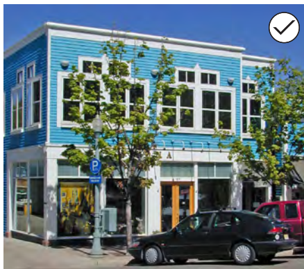
107. Design the mass of a new commercial or mixed-use building to reflect the scale of a surrounding residential district.
