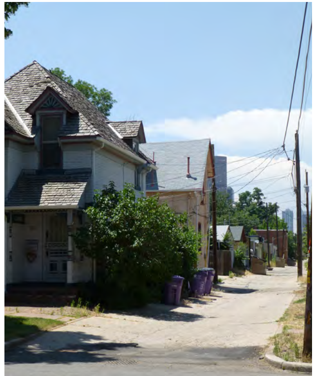
13. An alley streetscape within the district. Note the primary structure fronting onto the numbered streets with relatively small side yard setback next to the alley, the two-story carriage house behind the primary structure on the numbered street, the smaller one-story carriage houses in the background, and the service nature of this alley streetscape that allows the district to be free of power lines on the primary and secondary streets.
