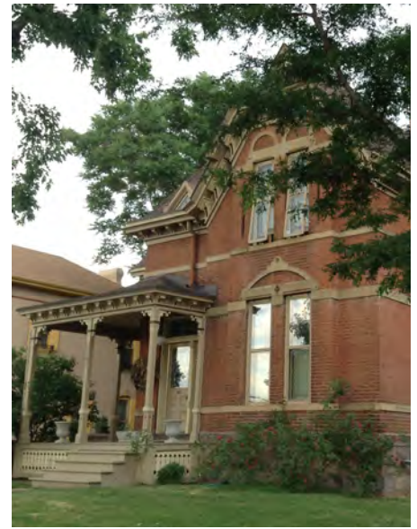
15. Elaborate Italianate style single family residence on Glenarm St. Note the stone foundation and brick walls, the projecting offset front porch and entry, the tall, narrow wood windows with elaborate headers and sills, and the heavy decorative cornice.
