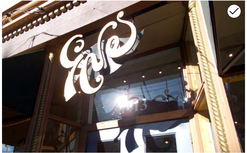
158. An arcade sign may be mounted parallel to the building front inside an entry arcade.
