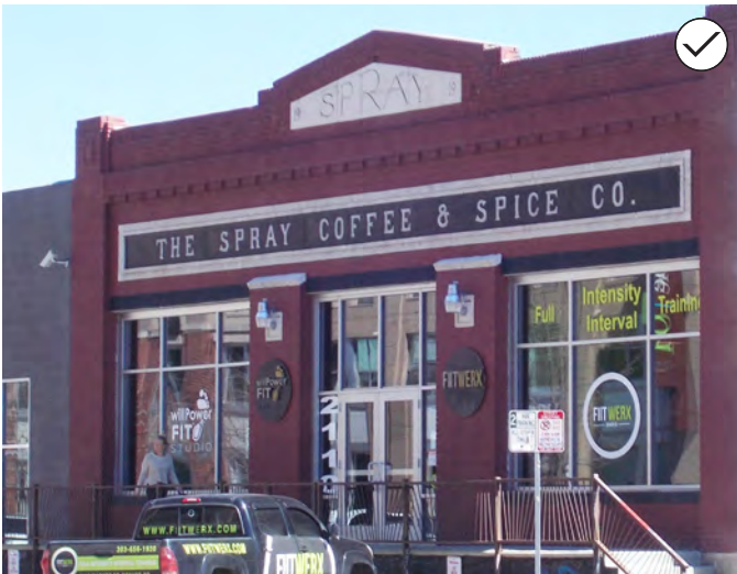
151. When using an existing sign band, provide space between the sign and the sign band edge. Keep sign flush with painted or pin mounted letters.
