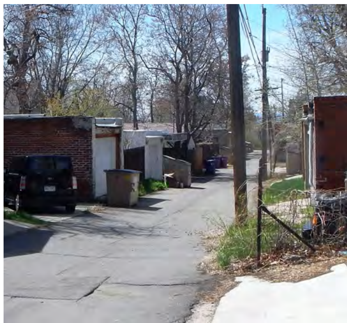
8. Typical alley way within Wolff Place. Note the low masonry one-story structures with single bay entries. The accessory structures on this alley feature flat roofs with parapets.
