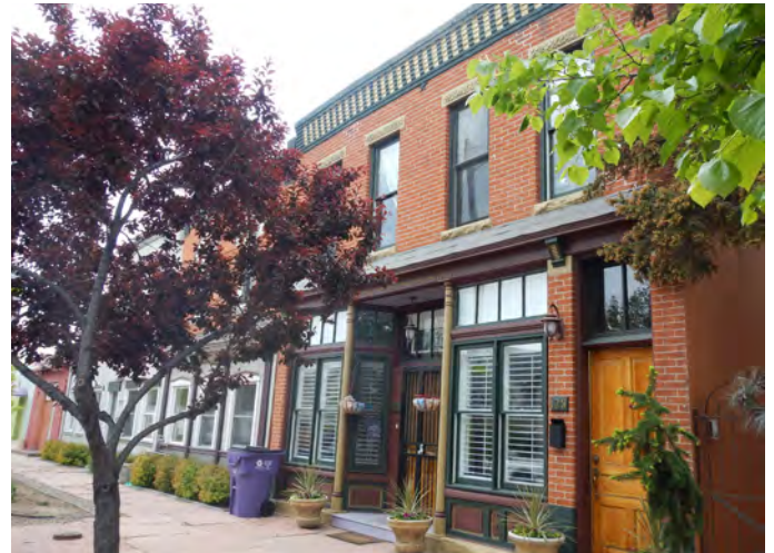
4. Historic commercial development within Baker. Note the two story massing, the recessed central entry with offset side entry, the storefront windows with transoms above and the decorative cornice.
