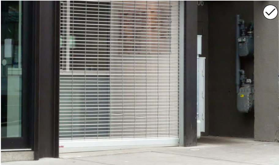
61. Use operable and transparent security screens on ground floor storefronts, when necessary.
