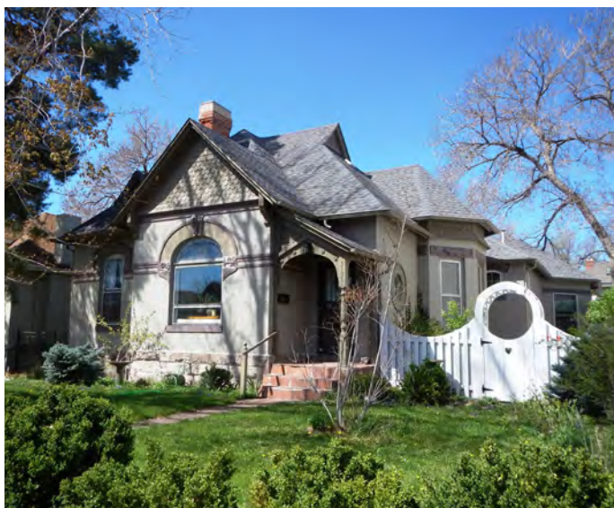
3. Queen Anne style cottage. Note the complex roof form, the fish scale shingles, the stone foundation, the decorative banding, the arched window with semi-circle brick arch above, and the spindle column on the covered stoop entry.
