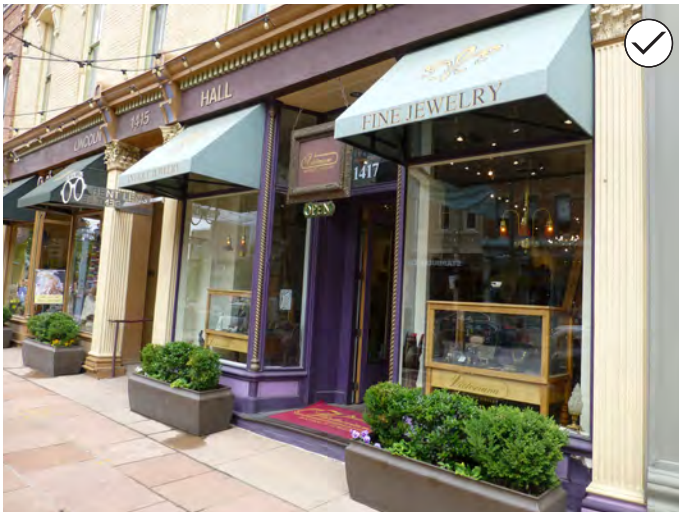
139. Coordinate sign locations, types and sizes to create consistency among multiple tenants in one building, such as the multiple retail tenants in this building.
