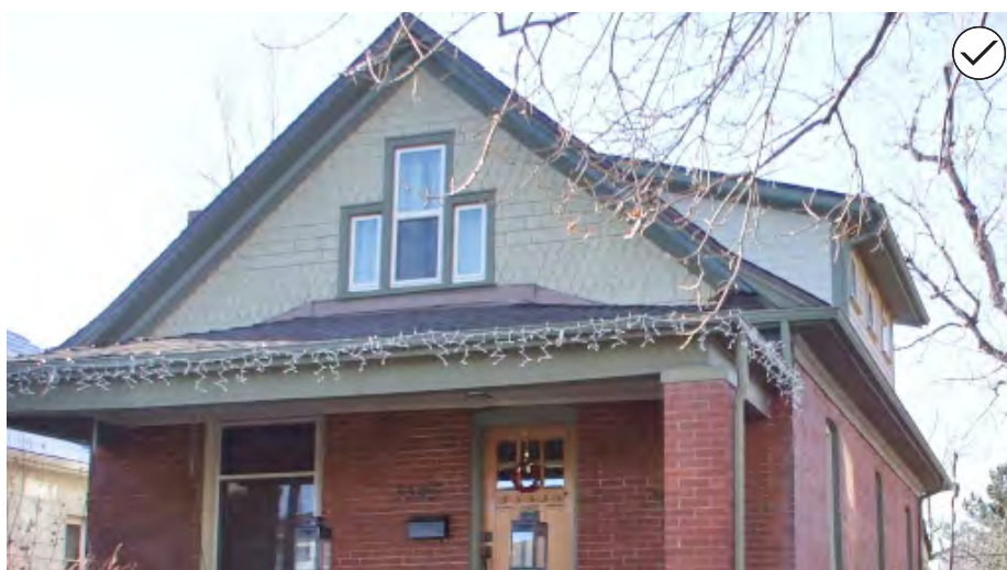
27. Design a dormer to be subordinate to the overall roof mass and in scale with those on similar historic structures.
