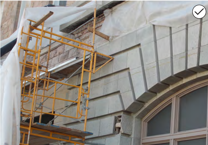
56. Minimize damage to historic structures when demolishing non-contributing additions or features. A non-historic addition was removed from the façade illustrated at left, allowing the original exterior to be repaired. A non-historic porch was carefully removed from the front of the house illustrated at right.
