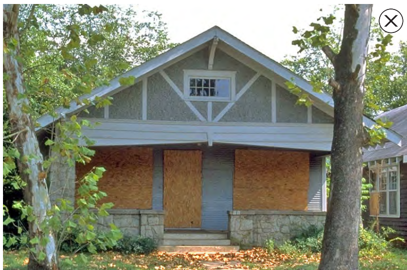
55. When closing off a window or door opening, paint the boards or panels to match the building color (left). Avoid mounting boards or panels on the exterior (right).
