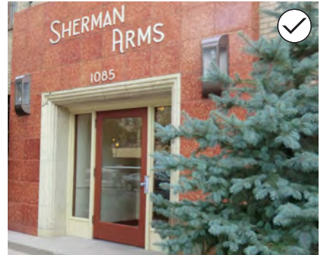
5. Preserve the character-defining features of a historic building, such as the moldings around this door and sidelight assembly.
