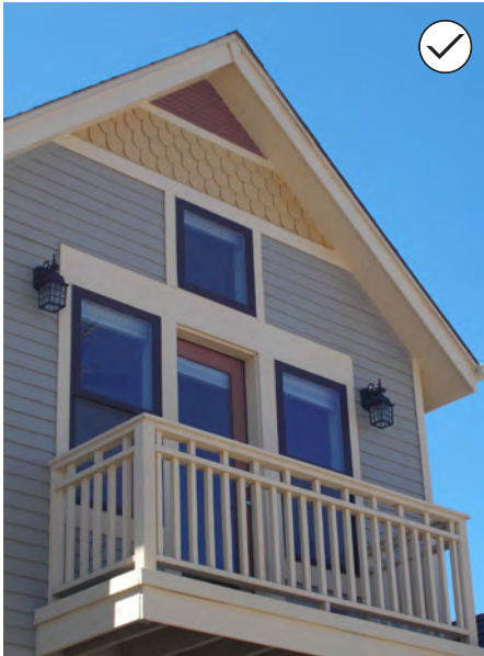
81. New materials that convey characteristics similar to historic materials may be considered, such as the smooth-finish (non-wood grain) fiber cement board illustrated above.
