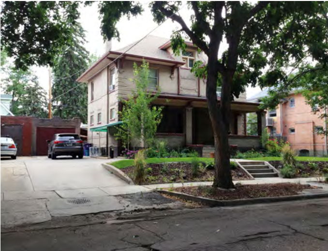
5. A historic curb cut onto East Park Place leads to a shared driveway with one-story accessory structures in the back ground.
