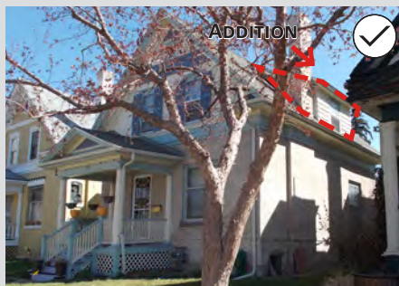
65. An appropriate side shed dormer addition, located behind the chimney. See "Dormer Location" on page 35 for more information.
