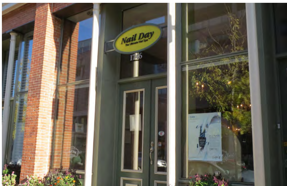
132. This signage was installed to limit impacts to character defining features of the building, such as the cast iron columns.
