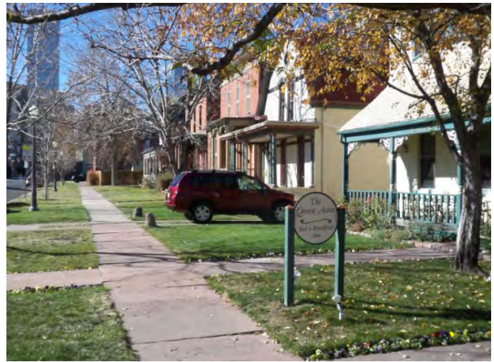
17. Sidewalk and walkways on Glenarm Pl. Note the at-grade historic sandstone walkways and sidewalks. The sidewalk is about 4-6 ft. in width and the walkways are about 3-4 ft. in width and lead in a straight path to the entryway, note the open front yards with no fencing.
