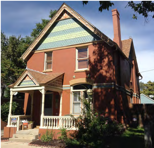
6. Typical Queen Anne development within the district. Note the forward facing gable with fish scale shingles and decorative sunburst and barge board, the projecting front porch with cross gable roof with a matching fish scale shingles and sunburst motif, the arched ground floor window.
