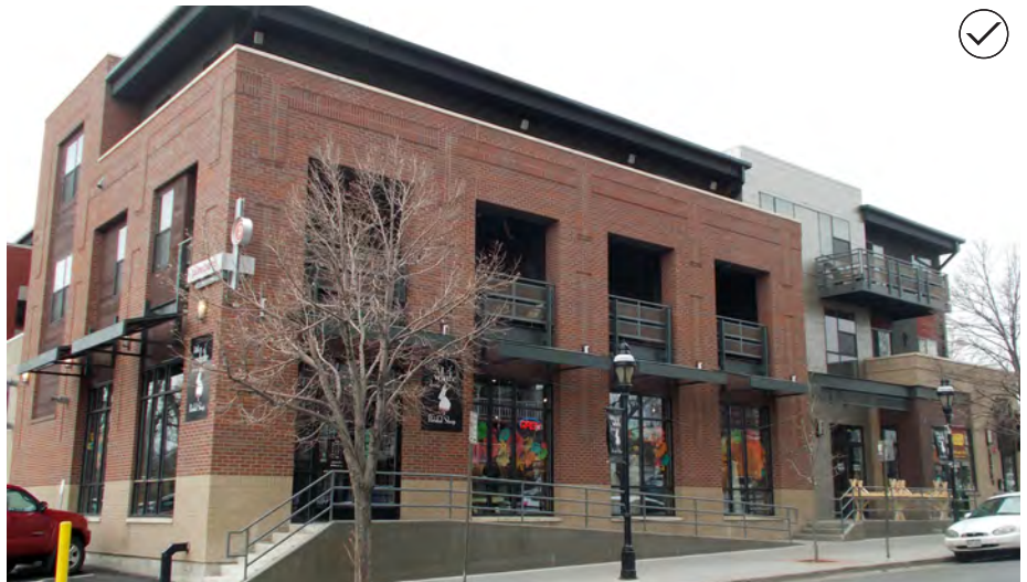
106. Divide the mass of a larger building into subordinate modules to reduce its perceived scale.
