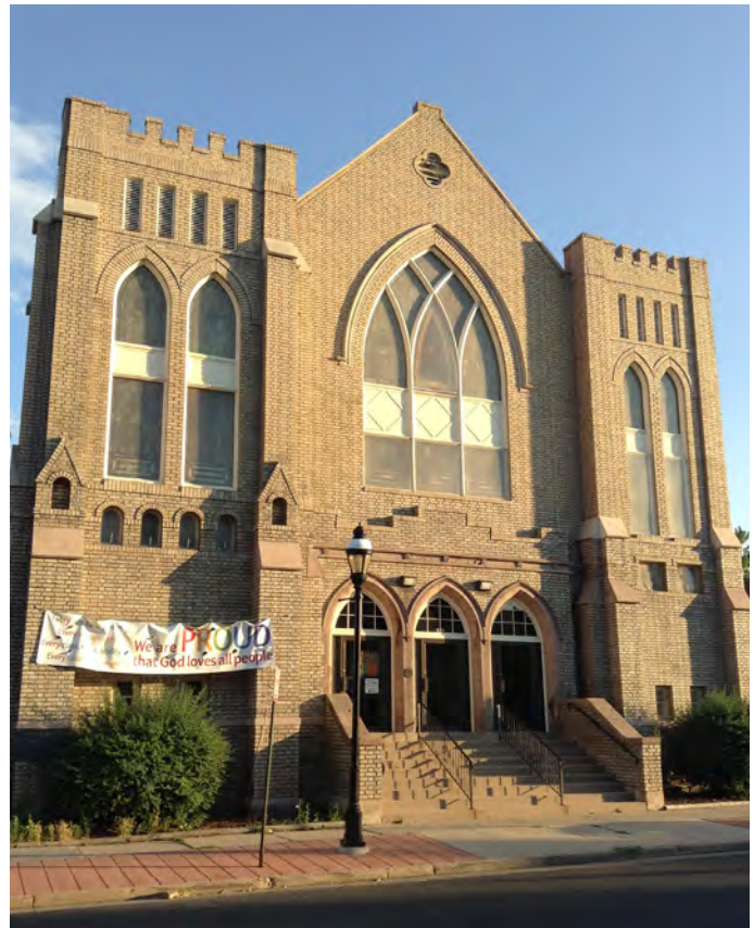
6. Gothic Revival Church. Note the arched windows with tracery, the crenellated side towers and the "castle-like" appearance of this structure.
