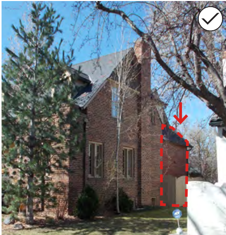
72. Place a one-story addition to the rear of the existing structure, if possible. The addition illustrated above is subordinate to the main structure and uses similar materials but is slightly differentiated.
