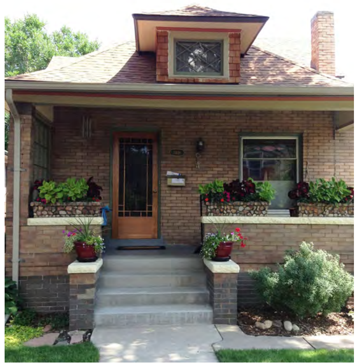
6. Craftsman Bungalow. Note the dormer window in the hipped roof, the masonry porch foundation and piers, the differentiation in brick from the foundation to the primary wall, and the offset entryway.
