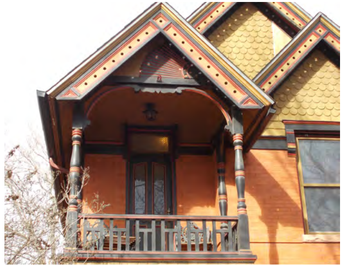
7. Second-story porch detail of a Queen Anne style building. Note the spindle columns, decorative balustrade, ornate barge boards, and the decorative fish scale shingles and sunburst motif in the forward facing eave. Also note the wood panel door with large decorative lights and transom.
