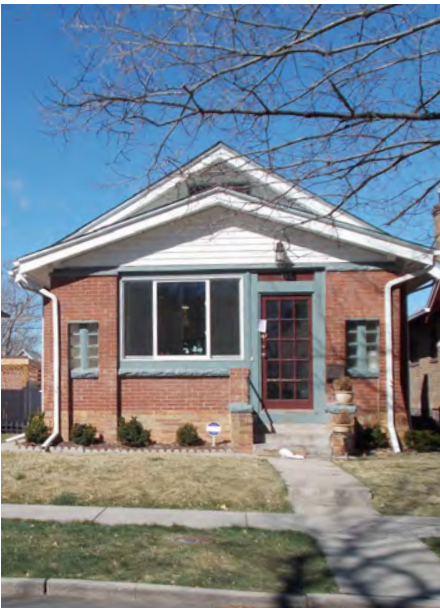
3. Non-contributing porch infill/enclosure in a historic district
