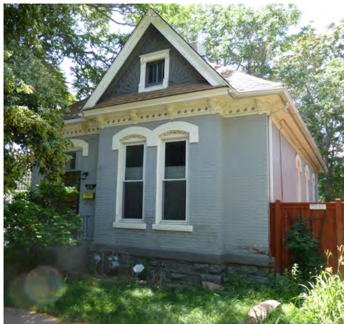
9. One-story Queen Anne Cottage within the district. Note the raised stone foundation, the paired window bays with arched brick headers, the decorative cornice and brackets and the forward facing gable with a sunburst motif.
