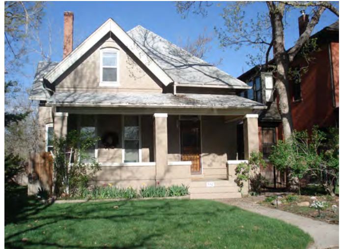
7. Queen Anne Cottage within the district. Note the simplicity of design with a primary pyramidal roof and a forward facing gable with barge boards.
