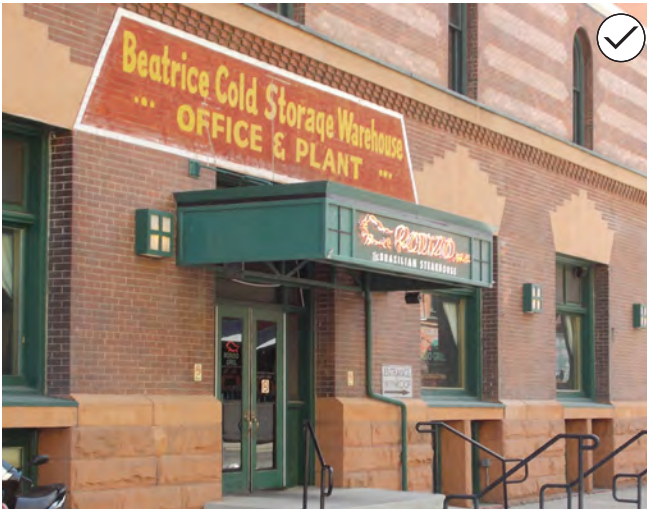
155. Use a canopy sign on a warehouse or industrial building where one would be traditionally found.
