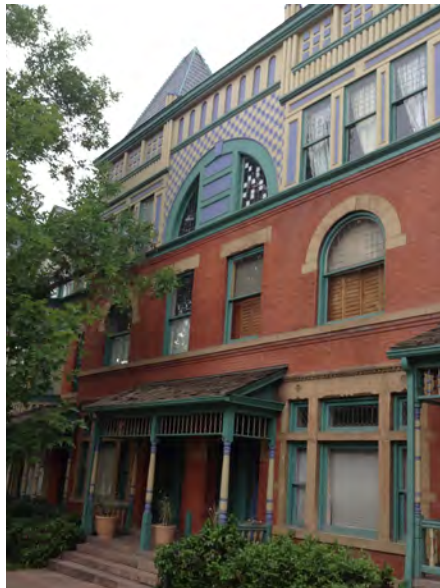
14. Queen Anne rowhouse on 21st Street. Note the historic sandstone sidewalk, brick construction with stone foundation, steeply pitched slate roof, and the one story porches with fretwork and spindle columns.
