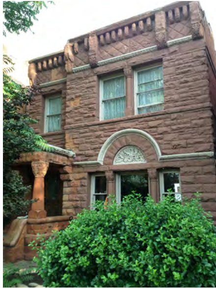
4. Romanesque style building on Stonemen's Row. Note the masonry façade, the Romanesque style column capitals, the semi-circle arch motif over a Palladian-esque window motif, and the heavy cornice.
