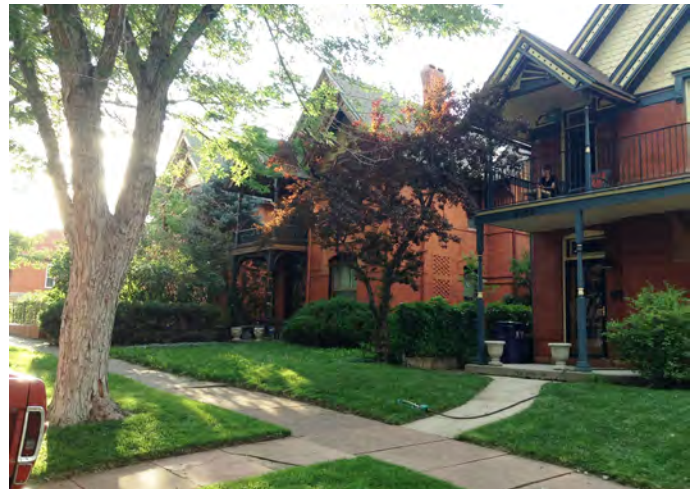
2. Streetscape on the north side of the district with Queen Anne Style buildings. Note the uniform setback and the large front yard, when compared to the front yards on Stonemen's row.
