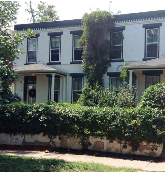
5. Italianate duplex on Alcott St. Note the decorative cornice on the parapet concealing the flat roof, the tall narrow double-hung windows with decorative headers and sills, and doors with transoms above.
