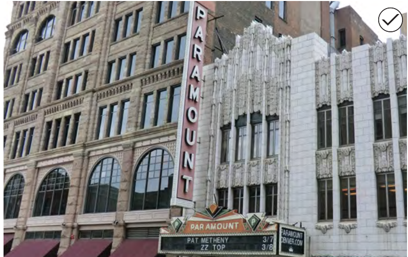
51. Preserve the overall rhythm and arrangement of windows on a historic commercial building façade.
