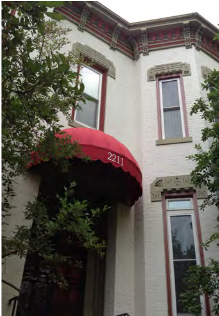
13. Italianate style rowhouse on Glenarm Pl. Note the heavy roof cornice, elaborate window headers, and tall narrow windows.
