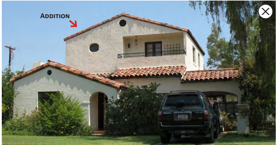
73. Design a rooftop addition to minimize impacts on the residential structure and context of the historic district. The rooftop addition illustrated above is incompatible because it overwhelms the original structure and has a high visual impact.
