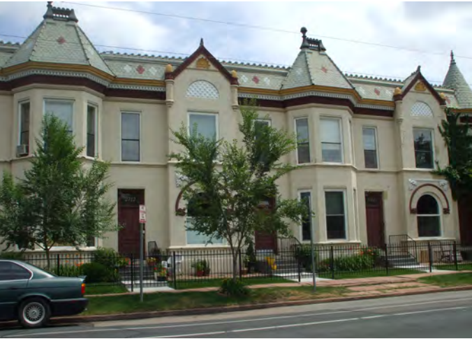
4. Multifamily Victorian eclectic dwelling fronting onto a primary street. Note the repeating projecting towers, the arched windows on the first floor with decorative headers, the transoms above the single entry door, and the decorative pattern roof.
