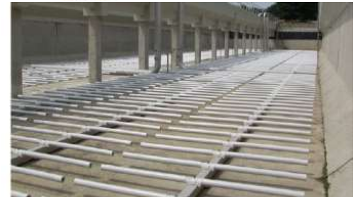
Figure 5-3. Example of Tube Membrane Diffusers. (OTT Magnum FLEXSIL)
