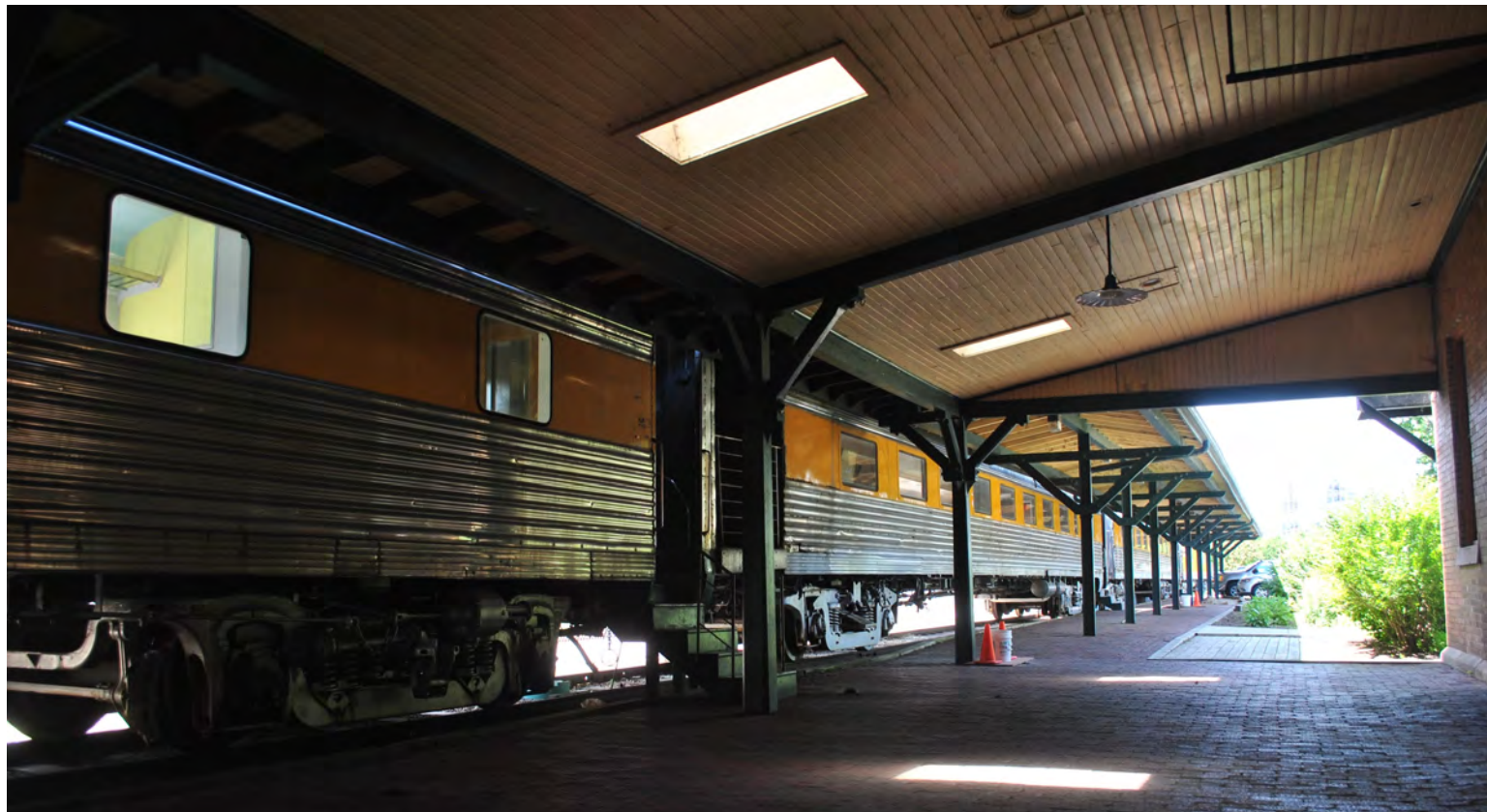
View from the Platform Showing the 1903 & Mid-Century Canopies
