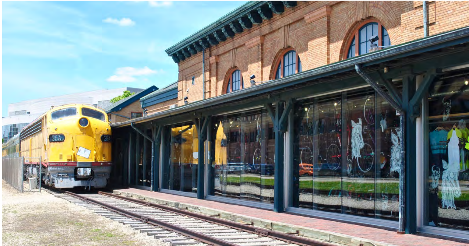
Locomotive with Enclosed Canopy Behind
