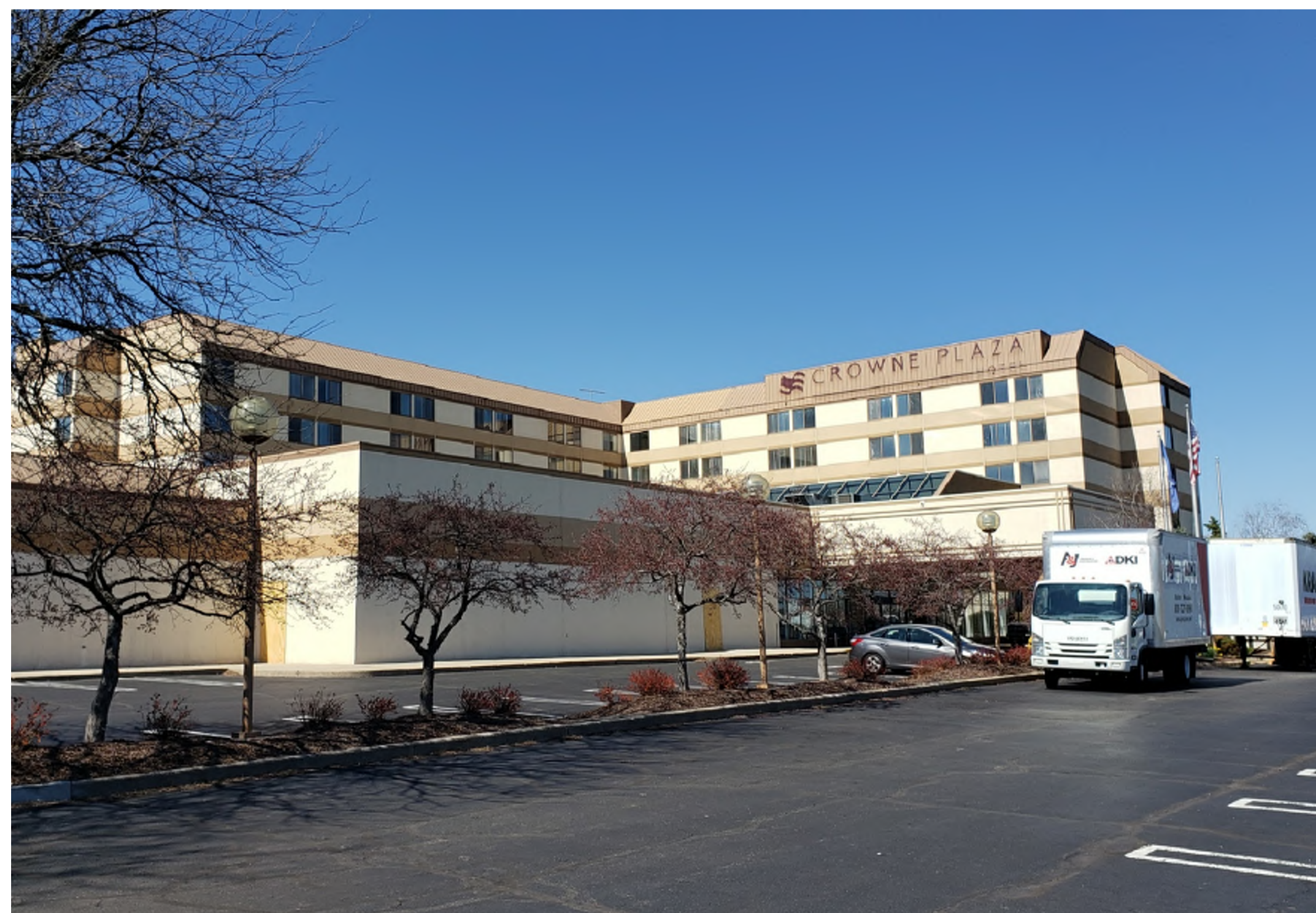
4402 East Washington Avenue - Exterior No. 3
