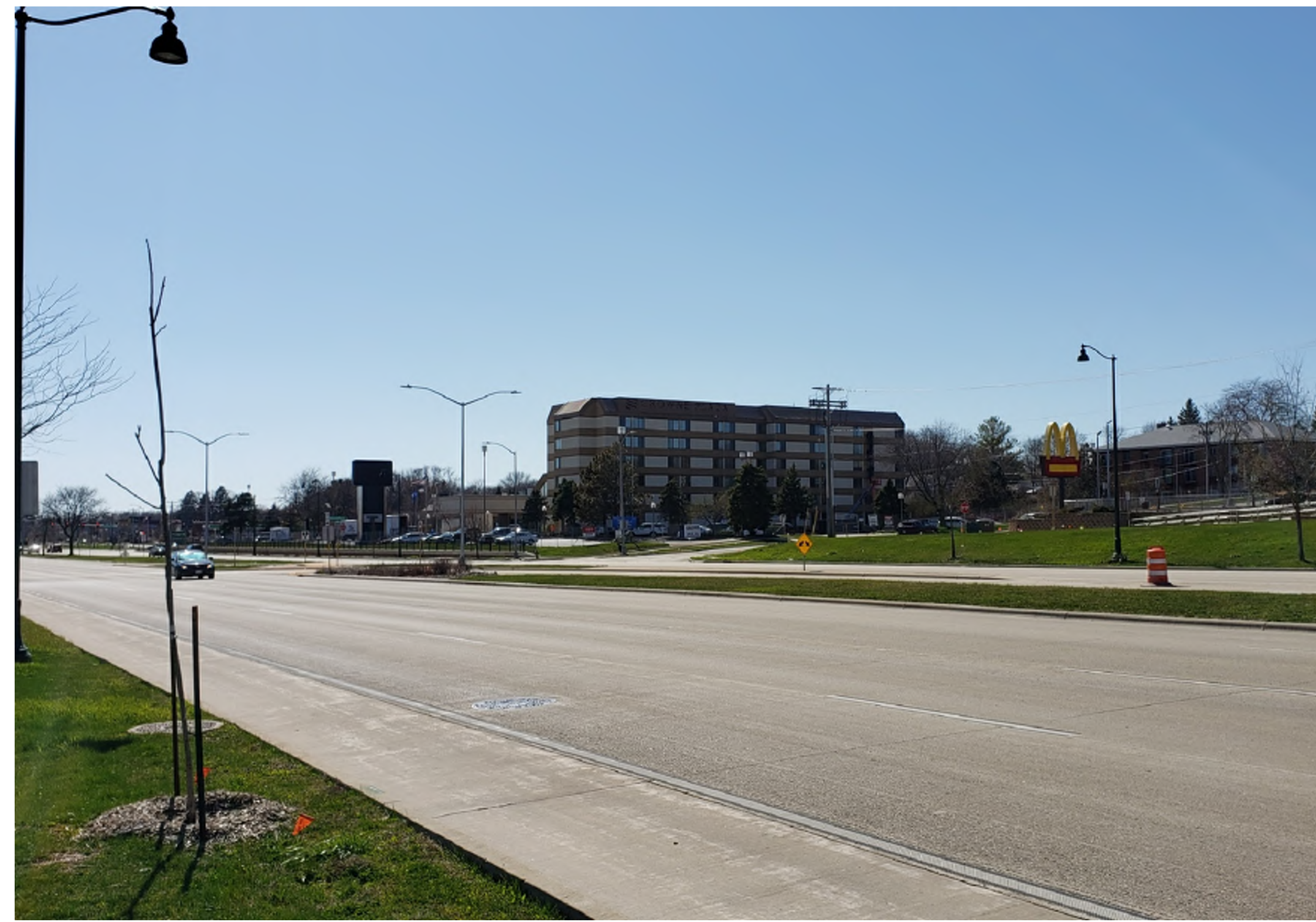
4402 East Washington Avenue - Exterior No. 8
