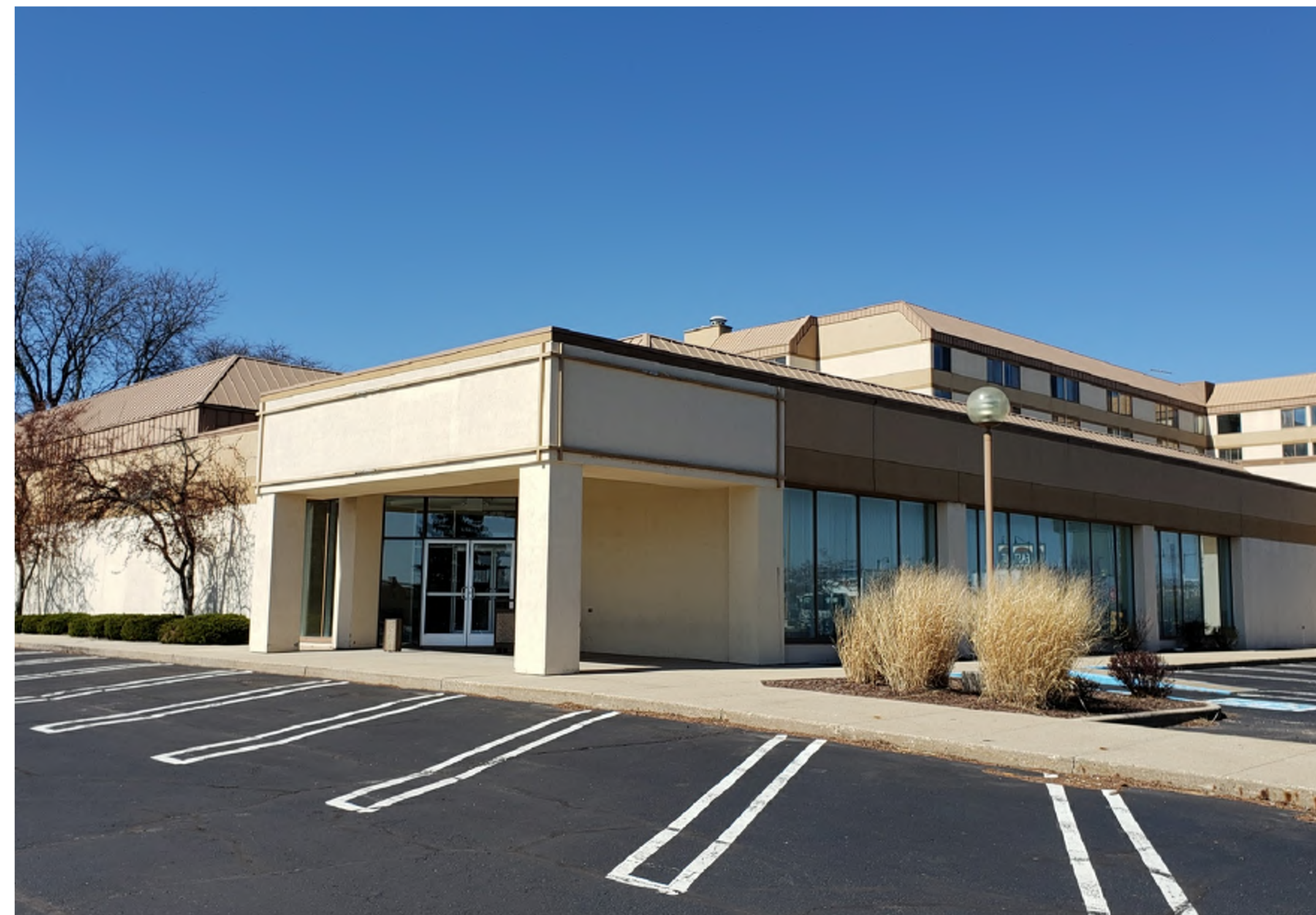
4402 East Washington Avenue - Exterior No. 5
