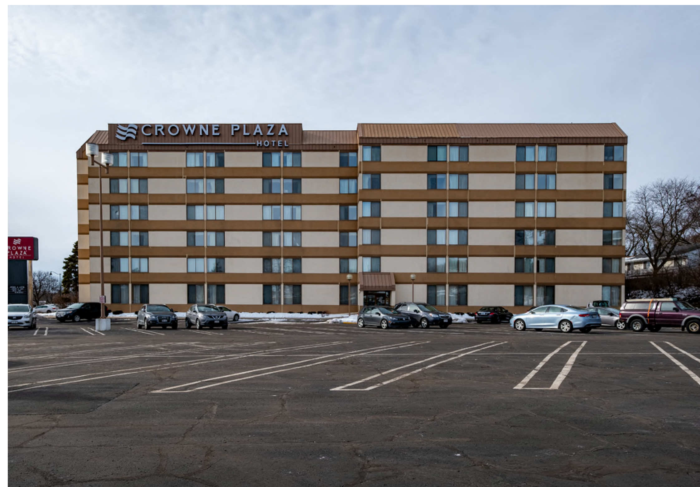
4402 East Washington Avenue - Exterior No. 2
