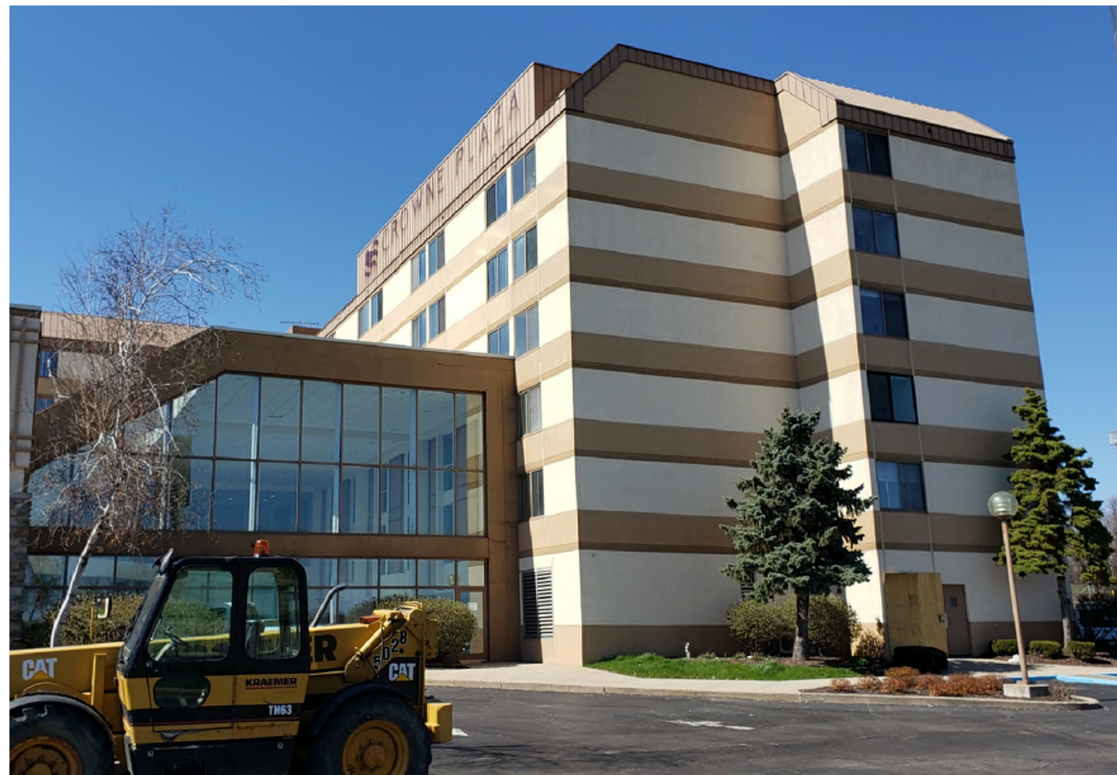
4402 East Washington Avenue - Exterior No. 6
