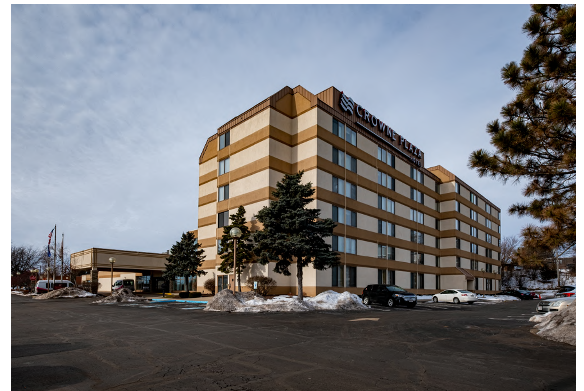
4402 East Washington Avenue - Exterior No. 1
