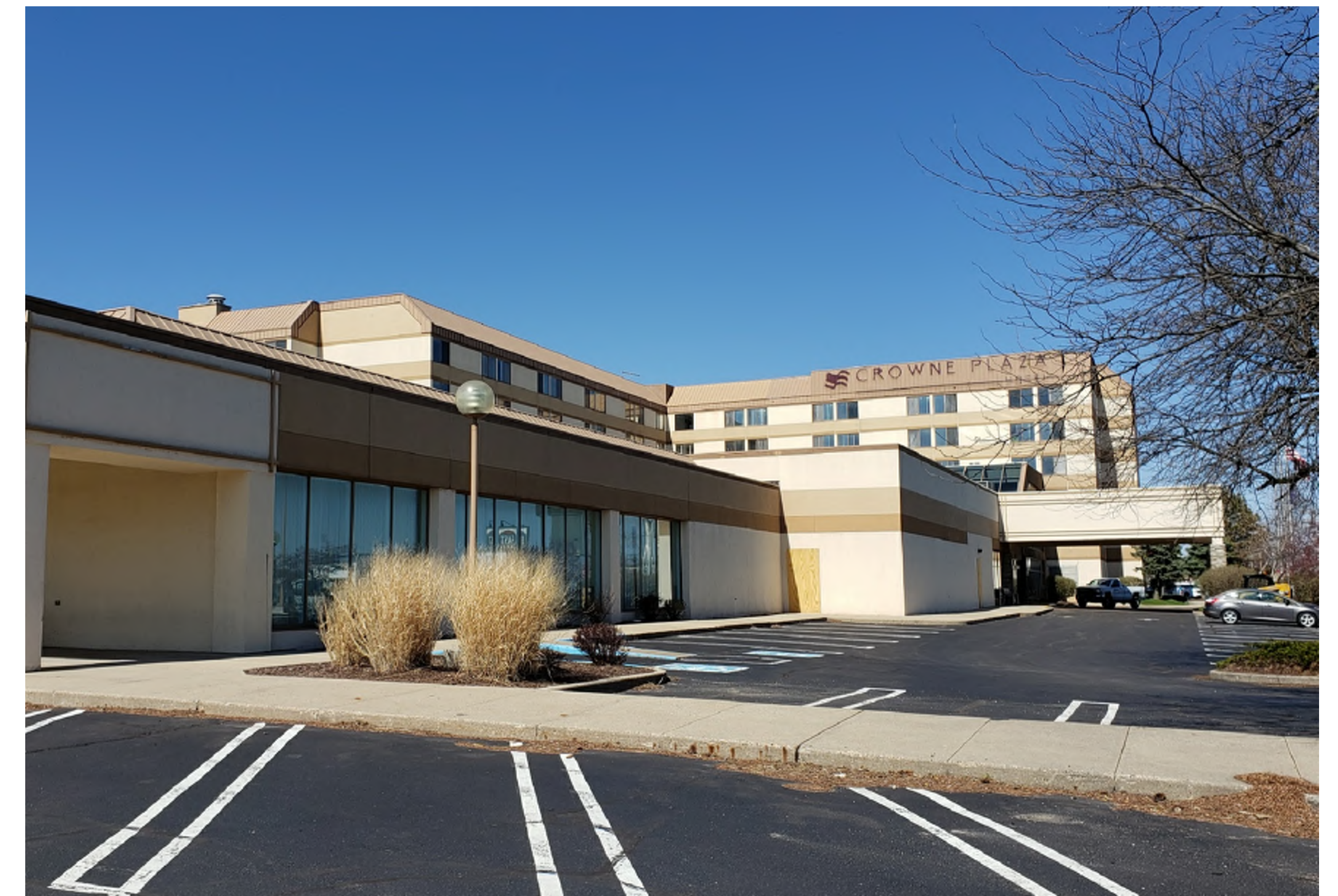
4402 East Washington Avenue - Exterior No. 4
