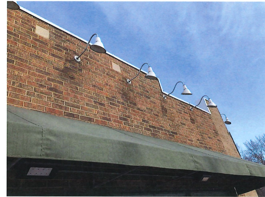
Existing Canopy -Reuse Existing, New to Matched Existing
