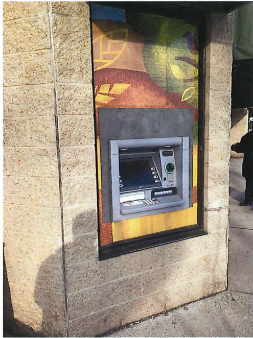
Existing Integral Color CMU -Reuse Existing
