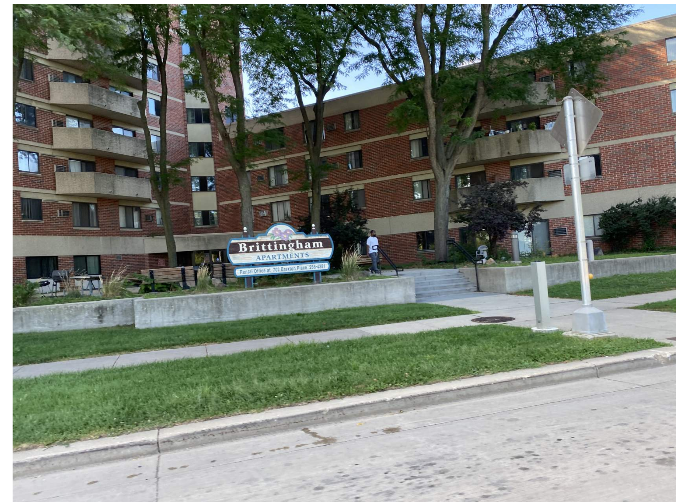
EXTERIOR - ENTRY ON W WASHINGTON
