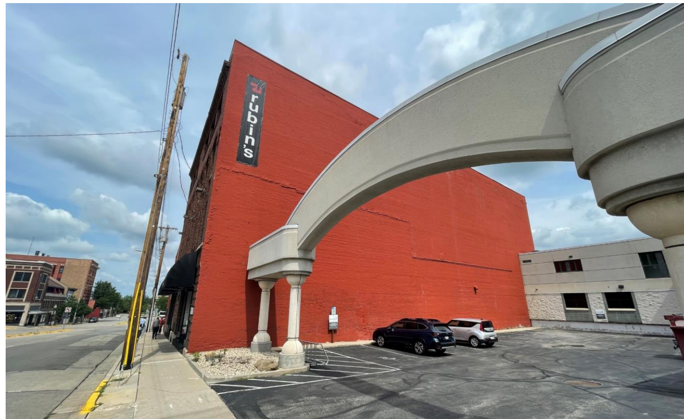
Image No. 3 Looking East
