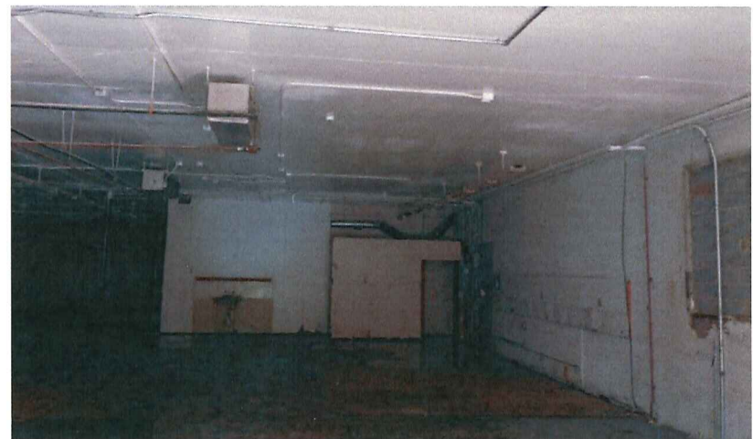
Existing Building Photos 2087 Atwood Ave, Madison, WI September 16, 2015
