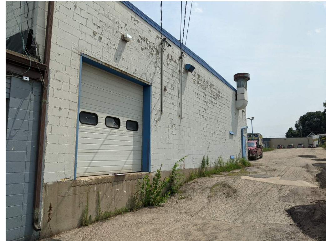
REAR FAÇADE (WEST)
