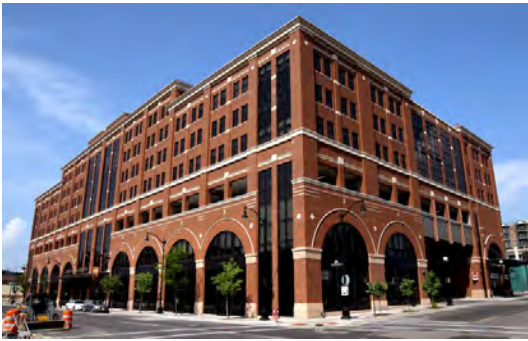
Grand River Station transit center, La Crosse, WI
