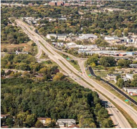
Stoughton Road and Highway 30 interchange
