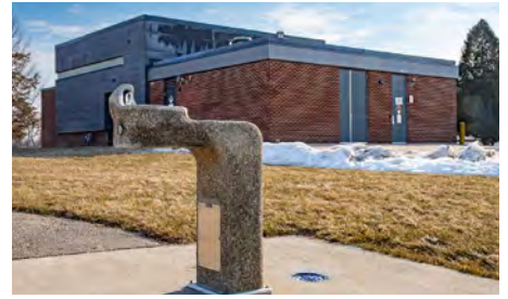
Madison Water Utility's Well 15
