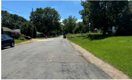
Missing sidewalks near Hawthorne Elementary School
