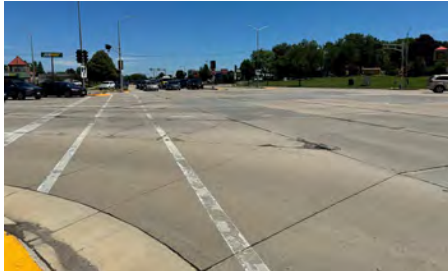
Pedestrian crossing of Highway 51 at East Washington Avenue
