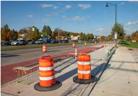
East Washington Avenue - construction of BRT station
