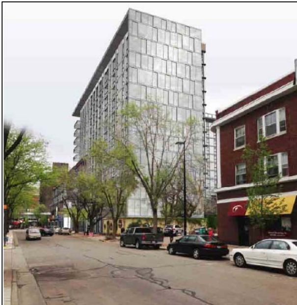
Original (Shear Wall Looking North from Frances St.)
