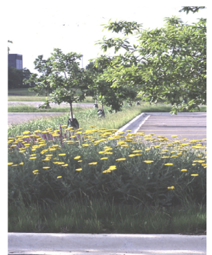
Fig. 2-4: Parking lot with bioswale to filter and absorb runoff. Shade trees reduce heat gain. Tellabs HQ, Naperville, IL.
