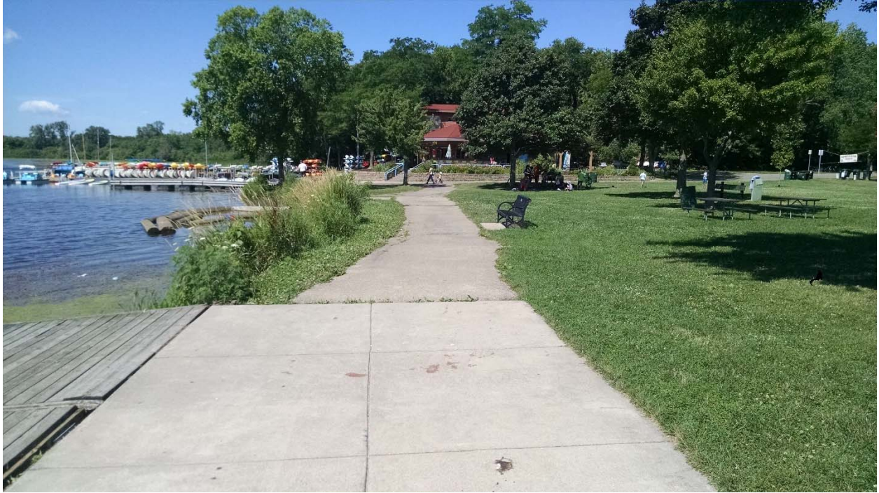
The asphalt path on site will be removed and replaced. The alignment will change slightly.
