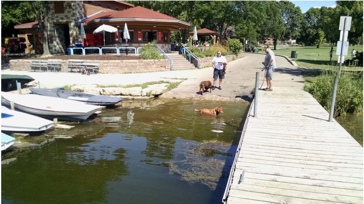
The existing boat launch will not be disturbed or altered. A graded, articulated block canoe launch will be constructed immediately east of the dock.
