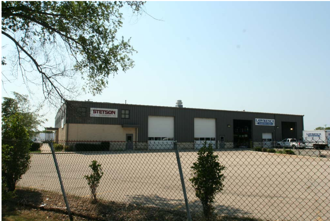
L 4015 TERMINAL DR. - STETSON BUILDING PRODUCTS
