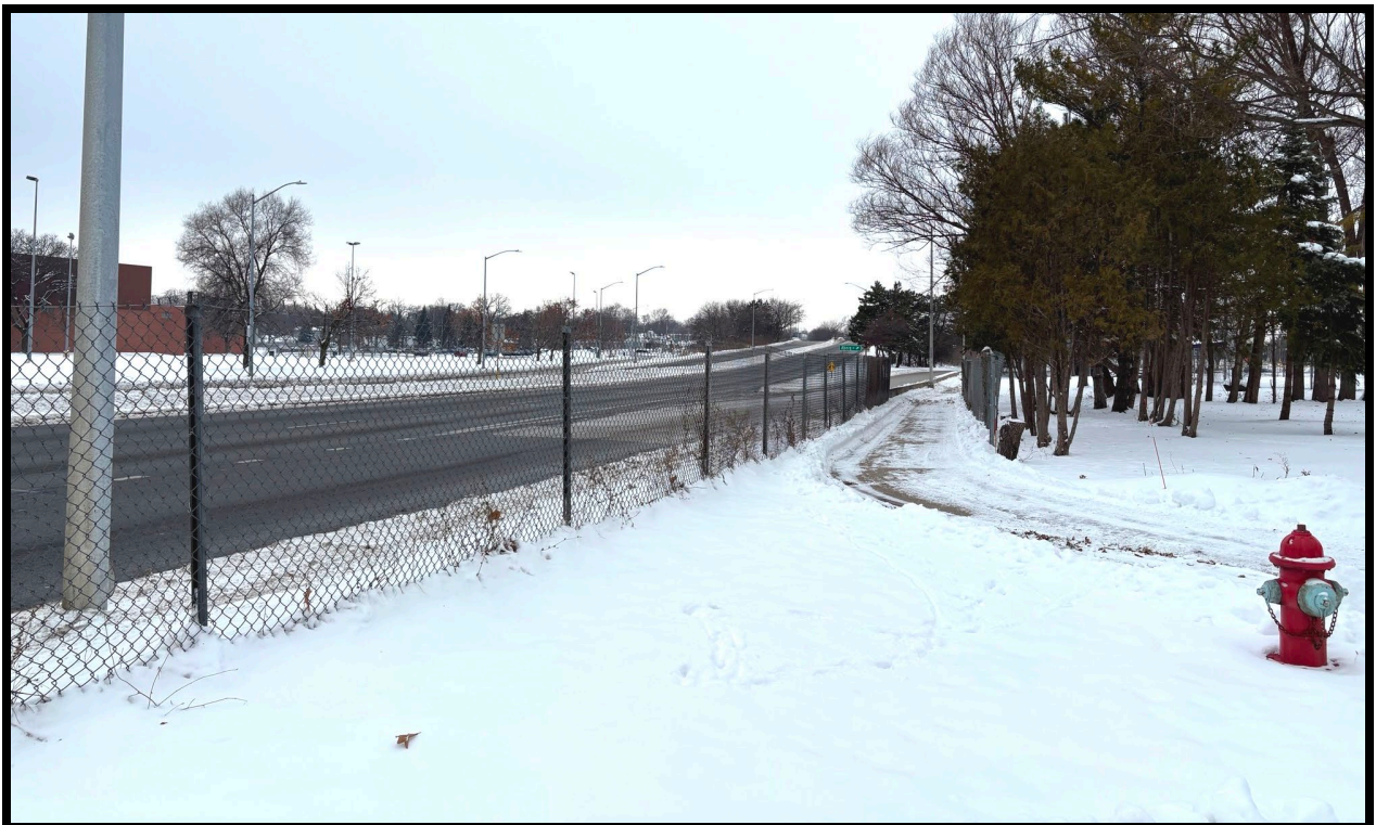
View of the Subject's Frontage along the Packers Avenue/Aberg Avenue Interchange Looking North – Subject on Right
