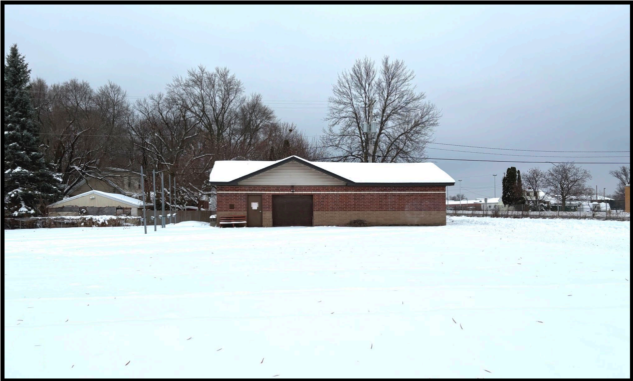
View from Roth Street Looking South towards the Maintenance Shop/Garage on the Subject Property
