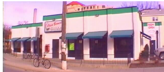
454 unknown date of construction
