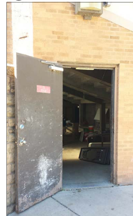
03 EXISTING SERVICE DOOR to LOWER LEVEL
