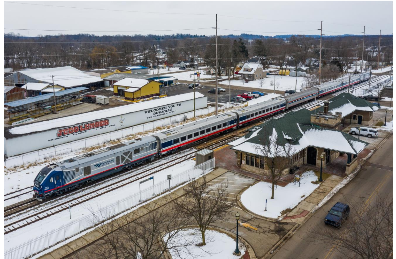
Amtrak Station in Pontiac, MI - Photo: Siemens Mobility
