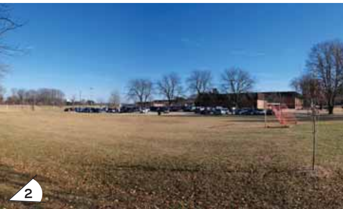
2 View of West side of the school
