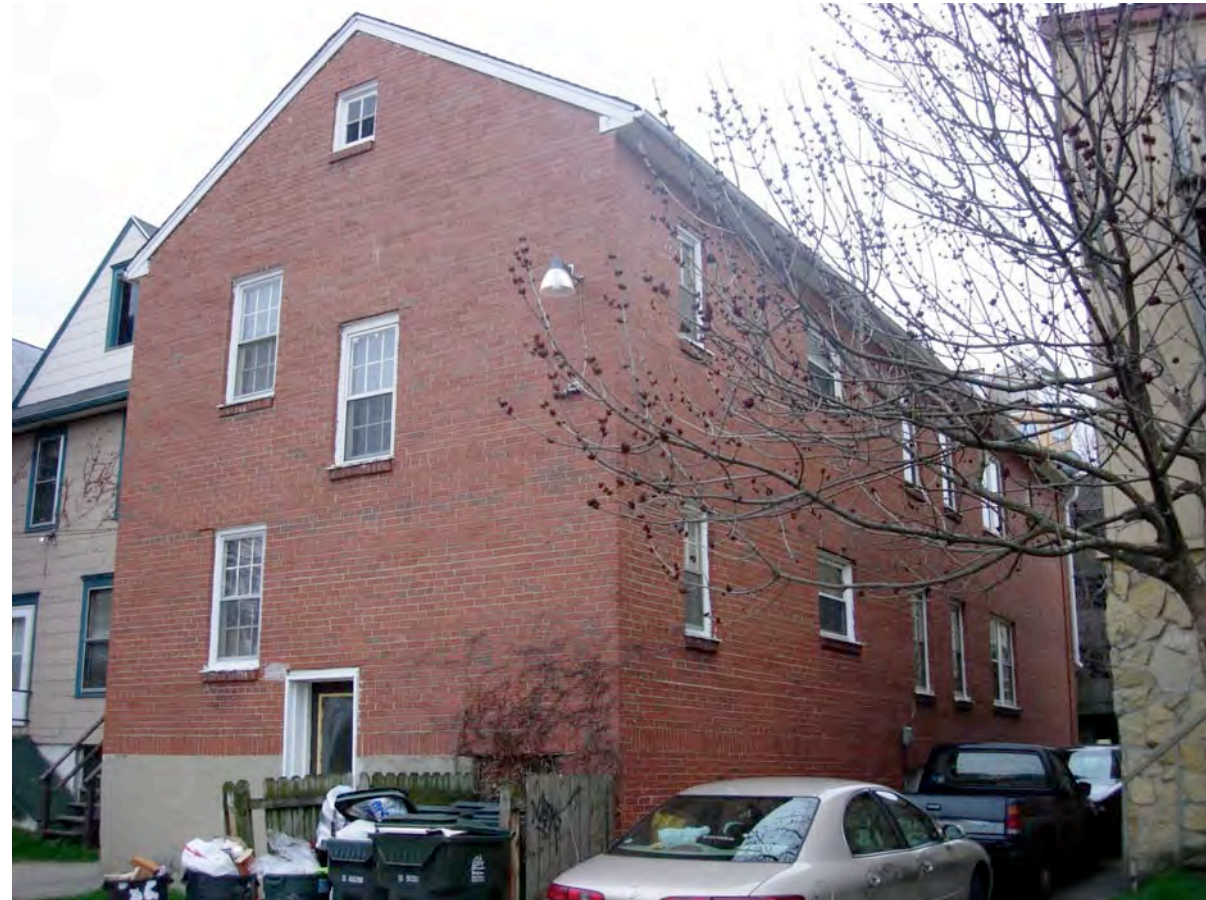
View from North East
