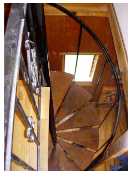
Stair Down to Second Floor
