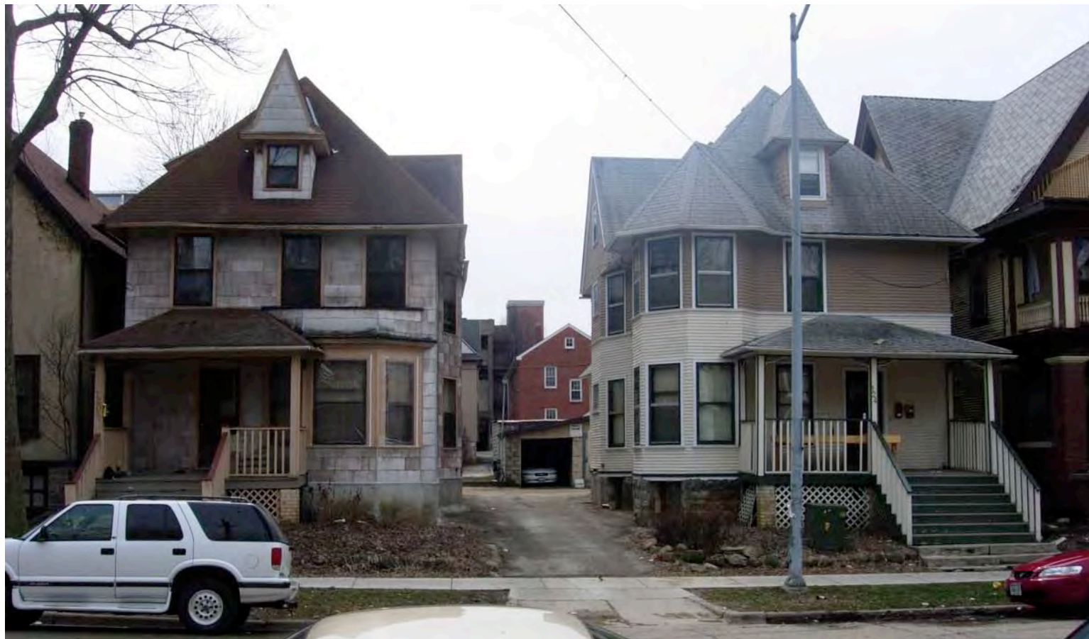
View West between 120 & 124 North Hancock
