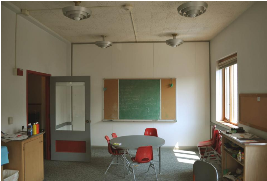
2 nd floor, Education Building, typical classroom.
