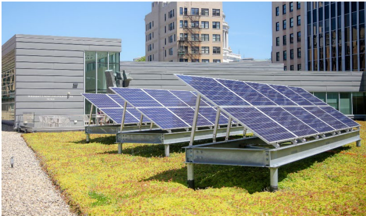
Solar Installations & Green Roofs
