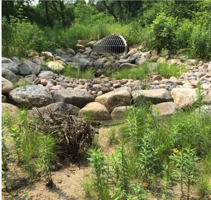
Improved Stormwater Management
