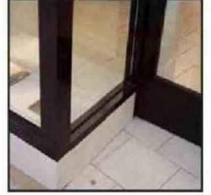
EWS-2 ALUMINUM STOREFRONT SYSTEM FINISH: ANODIZED BLACK
