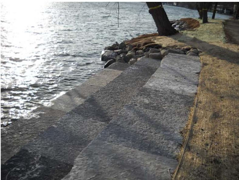
This photo to the left shows a previously installed, cut limestone step canoe launch. This particular installation is at B. B. Clarke Park, and was installed in 2011.
