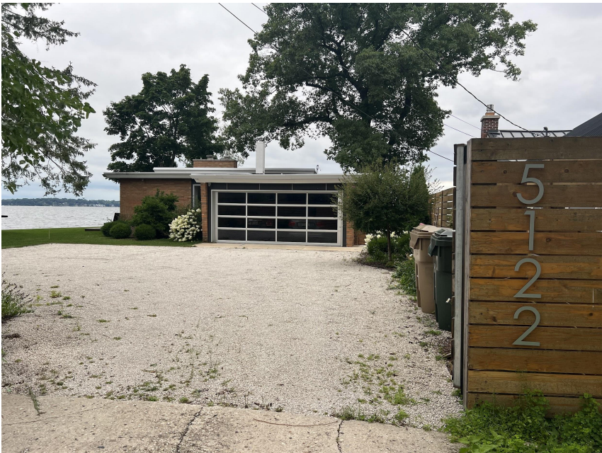
View from the driveway entrance (the "front yard") facing the garage which will be demolished and rebuilt as a part of the overall addition project.
