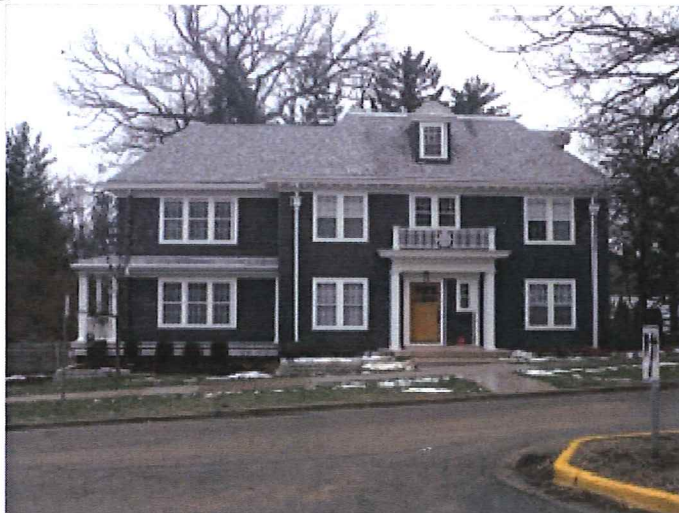
LARGE 2-STORY ADDITION, NEARLY FLUSH WITH FRONT FACADE, BUILT RECENTLY (LAST 2 OR 3 YEARS)
