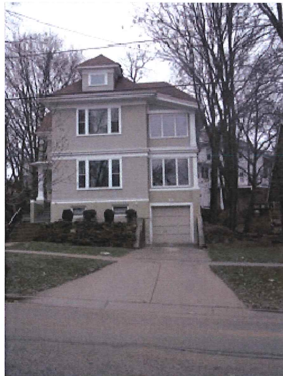
GARAGE WITH 2 UPPER FLOORS, NEARLY FLUSH WITH FRONT FACADE, APPROX. 3' TO PROPERTY LINE
