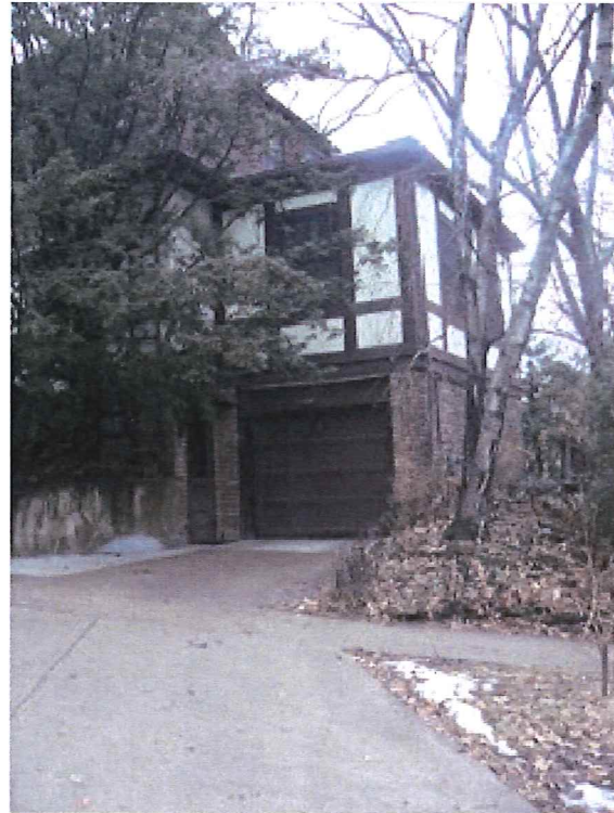
ORIGINAL CONSTRUCTION OF GARAGE AND UPPER FLOOR, APPROX. 3' TO PROPERTY LINE
