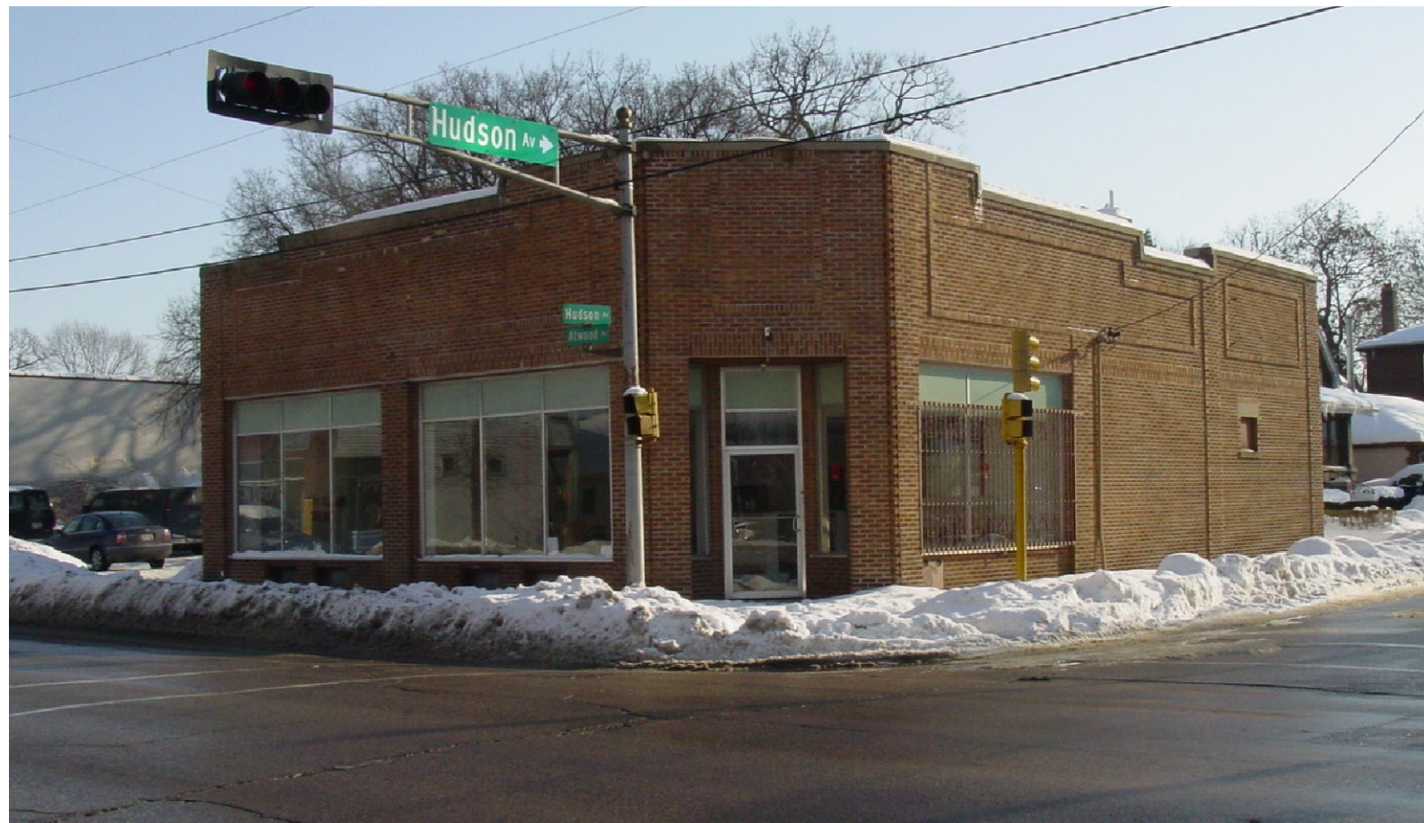
2. EXISTING BUILDING PHOTO NTS
