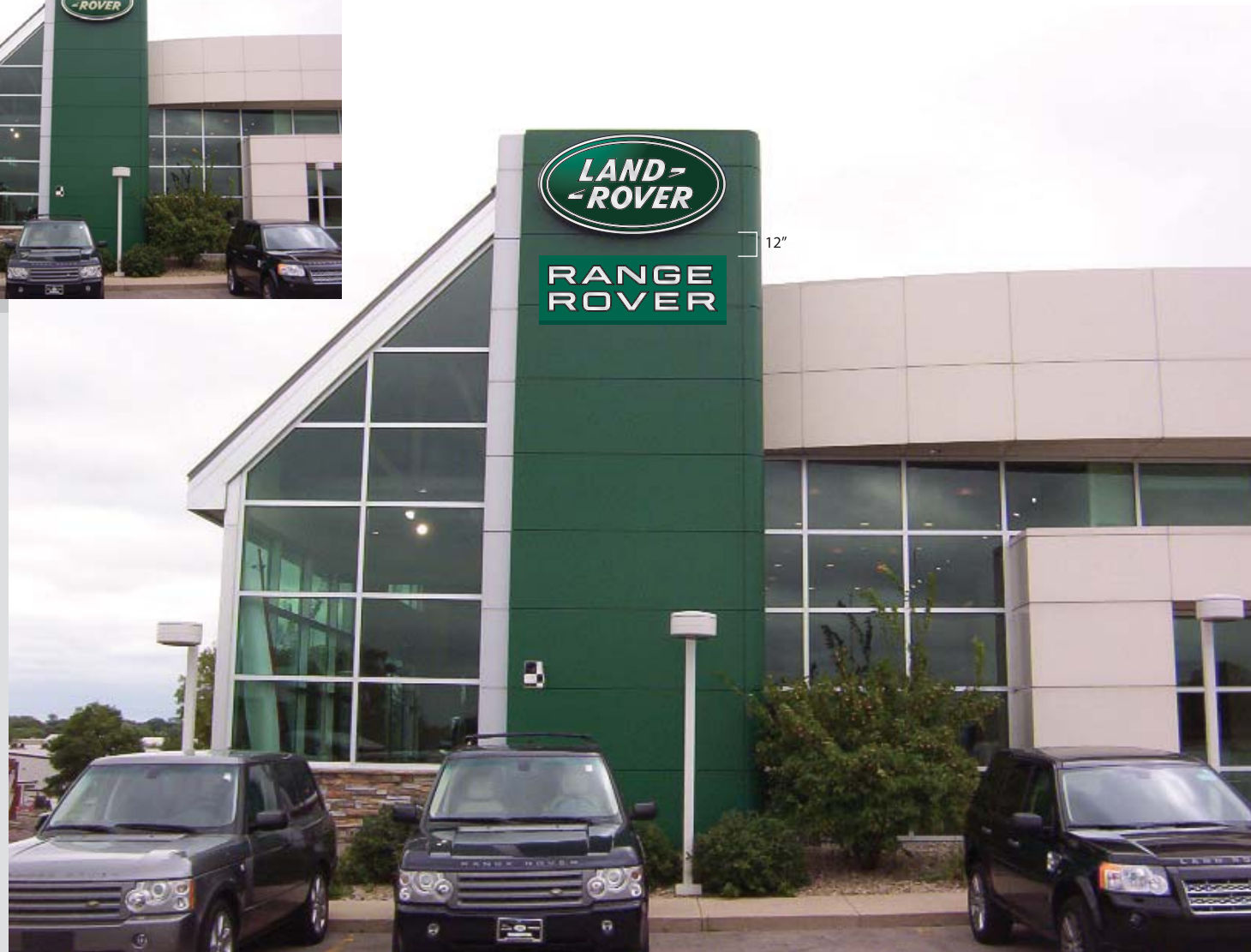
LR face replacement, new RR
