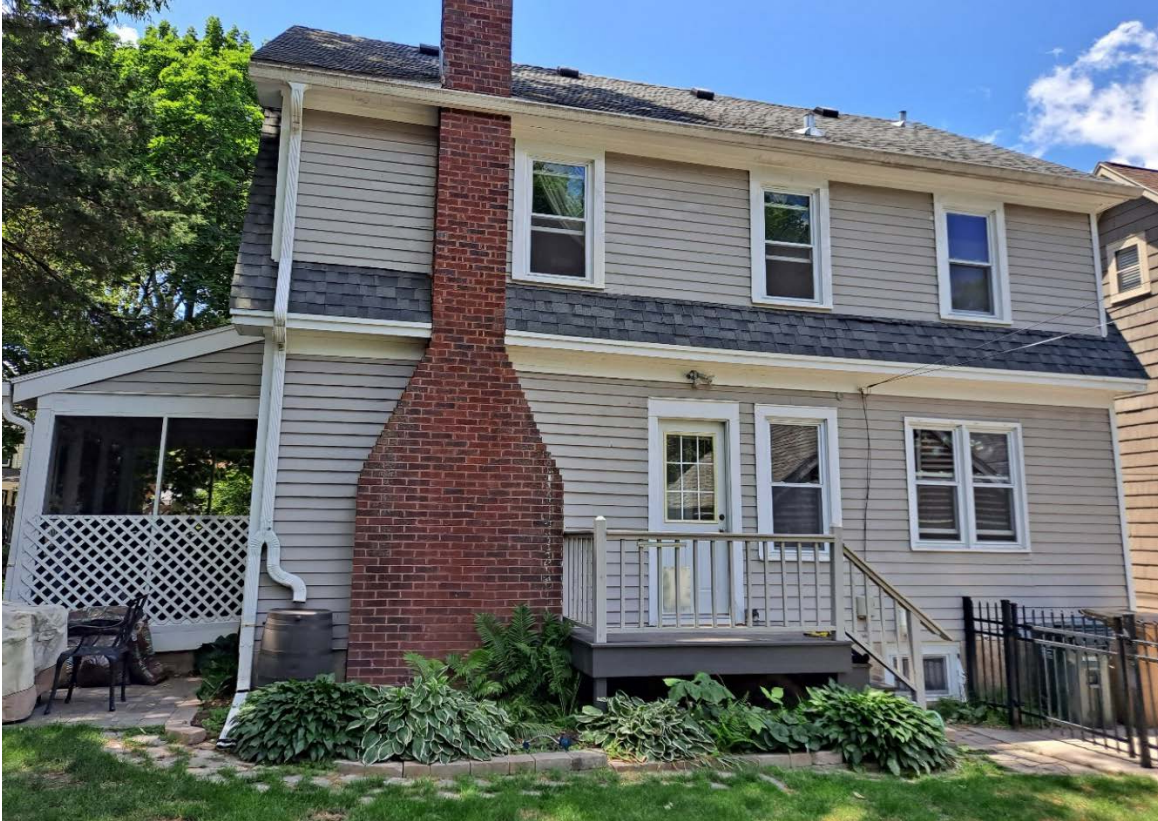
House - Existing Rear Elevation
