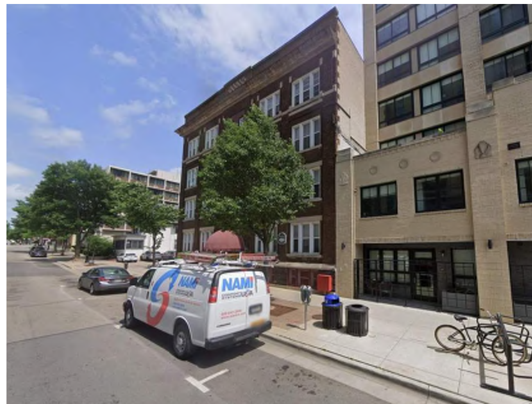
GILMAN SOUTHWEST END LOOKING EAST
