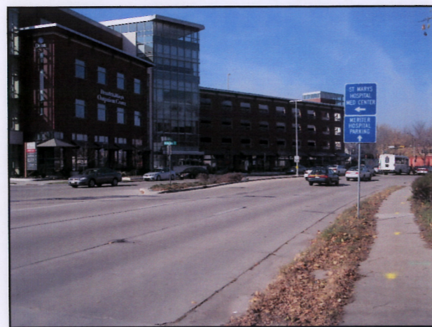
SOUTH CORNER OF LOT LOOKING NORTHWEST
