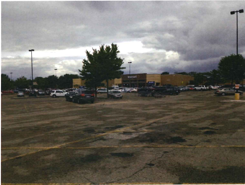
Front of Existing Store from Parking Lot Near Intersection of Commercial/Nakoosa
