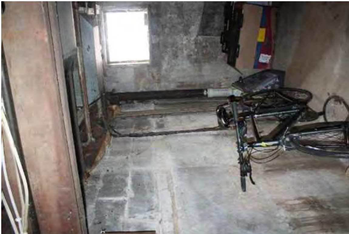
Photo 324: 410 1/2 East Washington Avenue, Interior, basement
