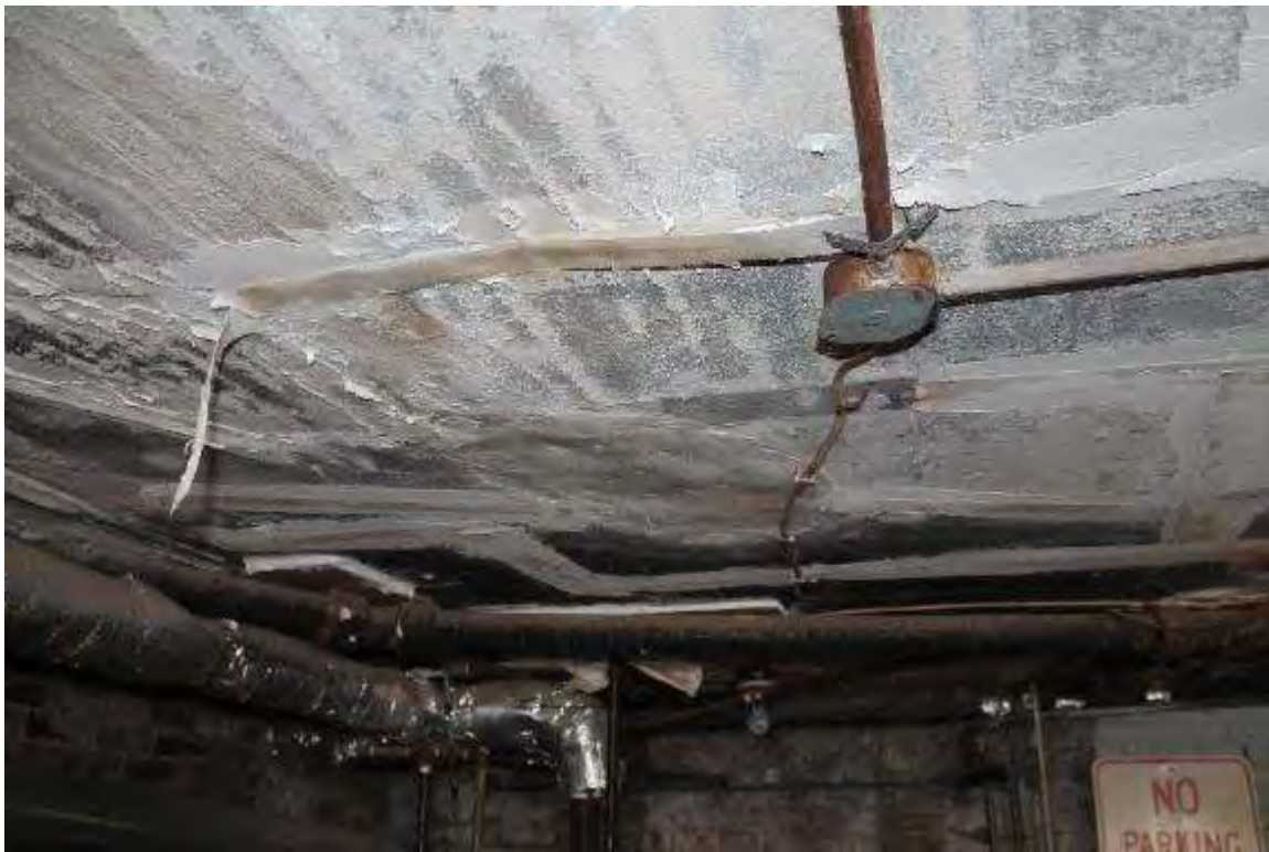
Photo 50: 9 North Hancock Street, Interior, basement
