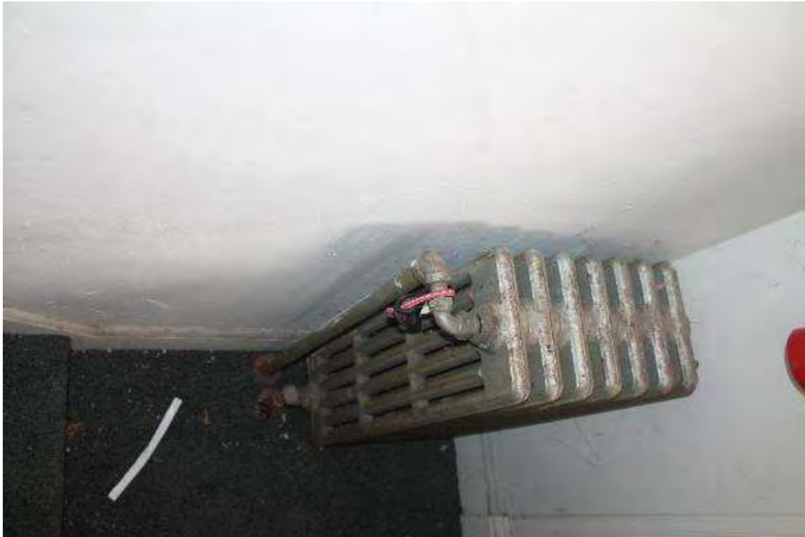
Photo 112: 12 North Franklin Street, Interior, first floor entryway
