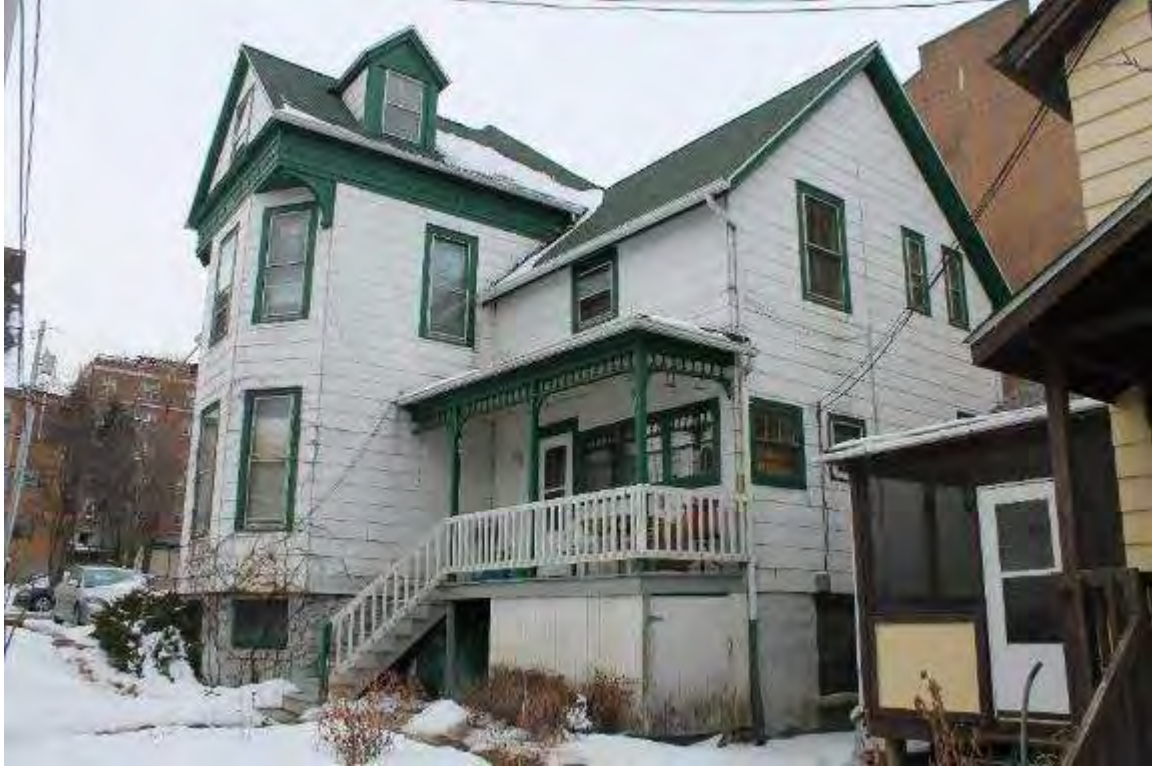
Photo 5: 9 North Hancock Street, Exterior, facing west
