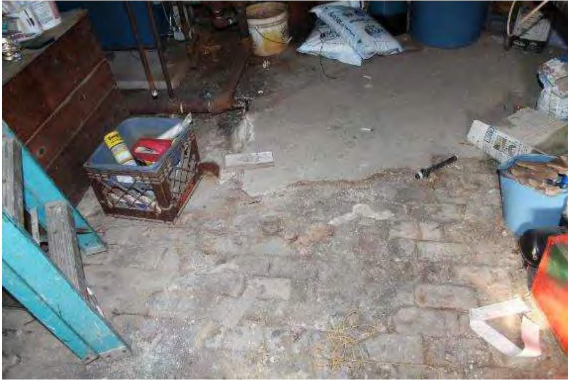
Photo 49: 9 North Hancock Street, Interior, basement
