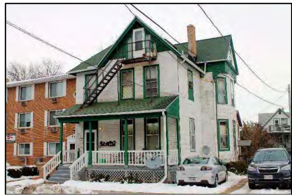
9 North Hancock Street
