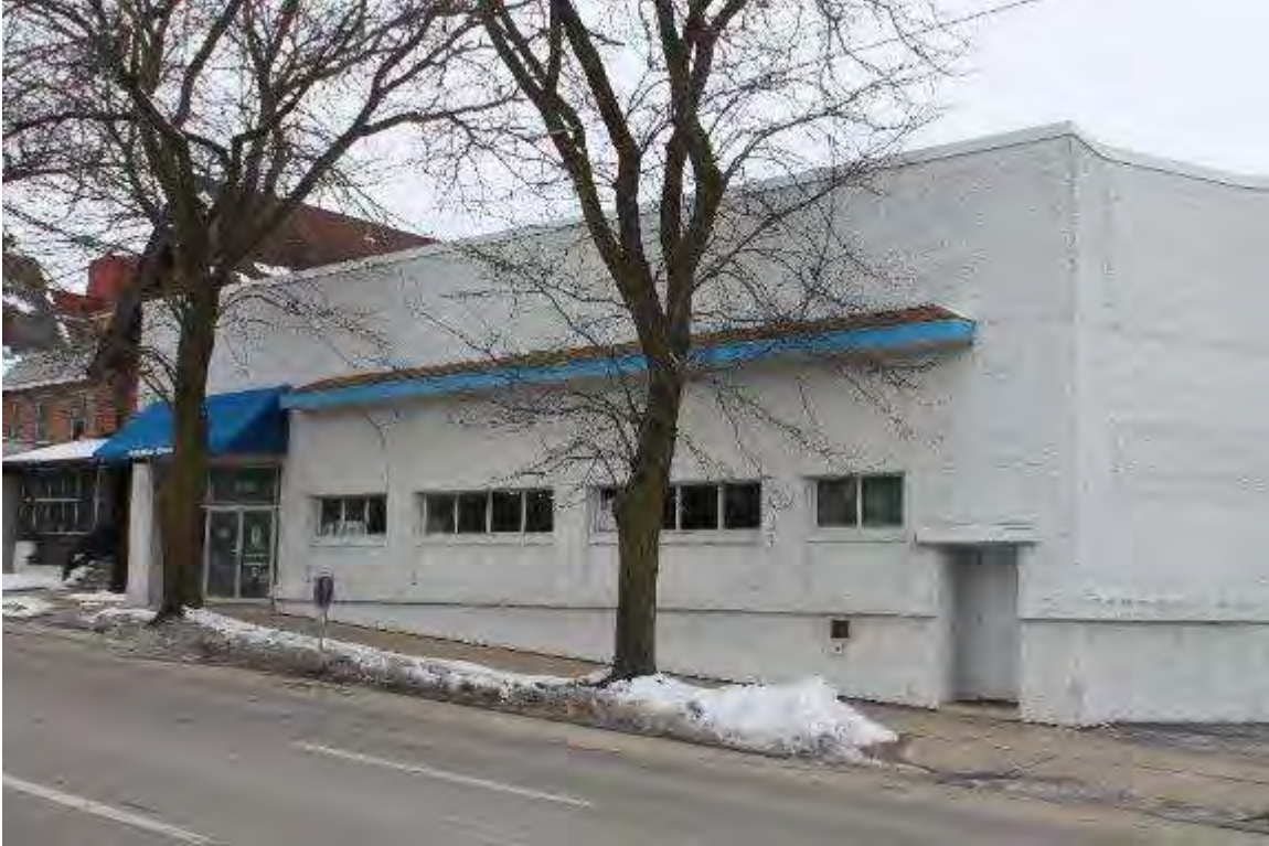
Photo 335: 412-414 East Washington Avenue, Exterior, facing west
