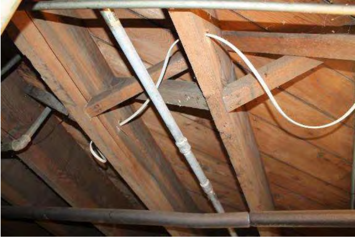
Photo 293: 410 East Washington Avenue, Interior, basement
