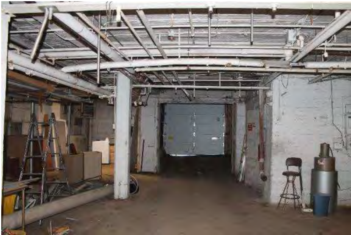
Photo 362: 412-414 East Washington Avenue, Interior, lower level storage space
