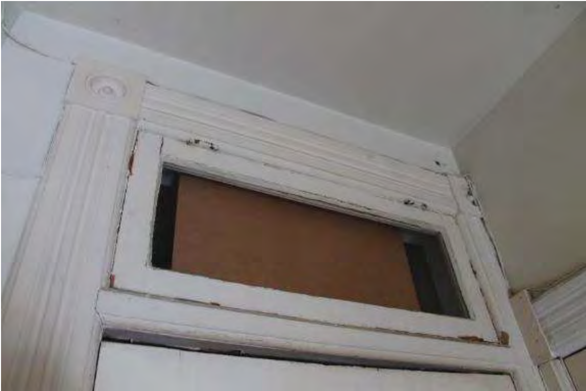
Photo 34: 9 North Hancock Street, Interior, second floor hallway
