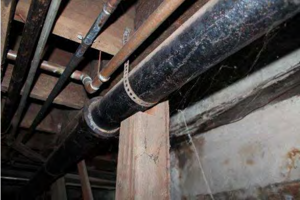
Photo 223: 402-408 East Washington Avenue, Interior, basement
