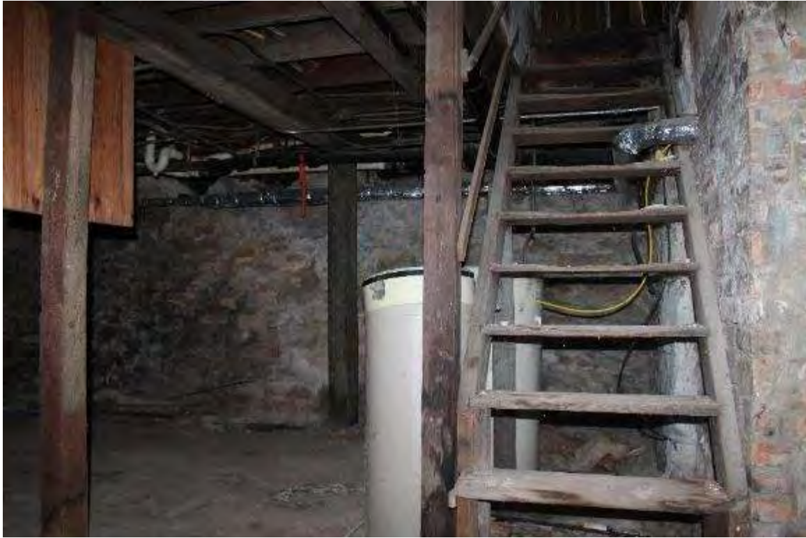
Photo 220: 402-408 East Washington Avenue, Interior, basement
