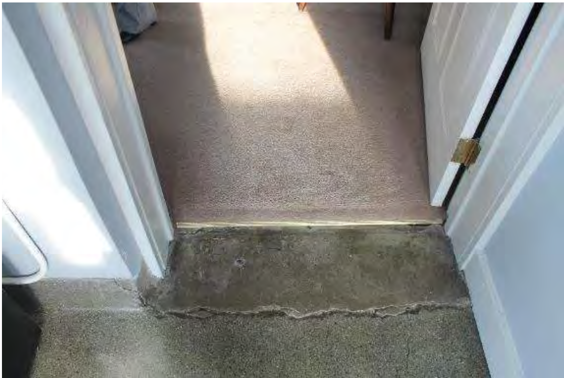
Photo 166: 402-408 East Washington Avenue, Interior, first floor commercial unit 1
