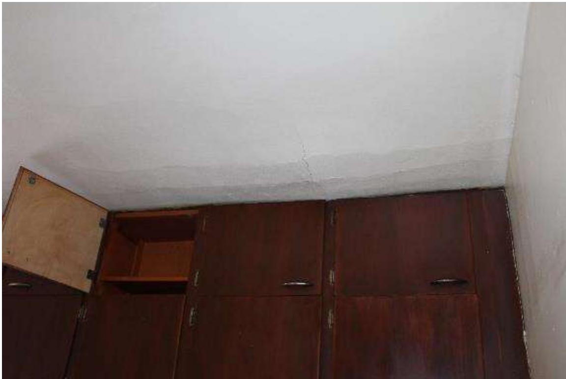
Photo 202: 402-408 East Washington Avenue, Interior, second floor unit 3
