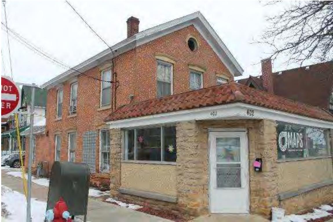
Photo 135: 402-408 East Washington Avenue, Exterior, facing north
