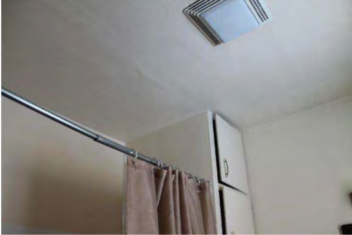
Photo 215: 402-408 East Washington Avenue, Interior, second floor unit 4
