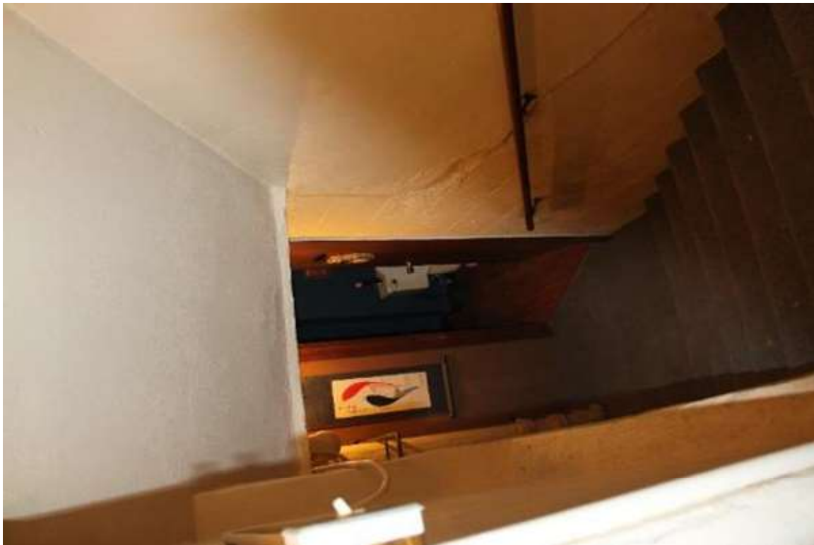
Photo 174: 402-408 East Washington Avenue, Interior, first floor commercial unit 2
