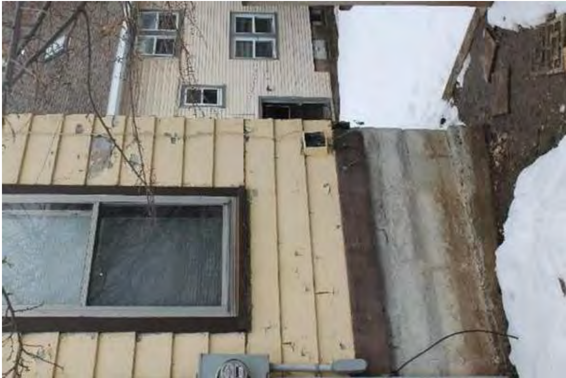
Photo 298: 410 1/2 East Washington Avenue, Exterior, facing north
