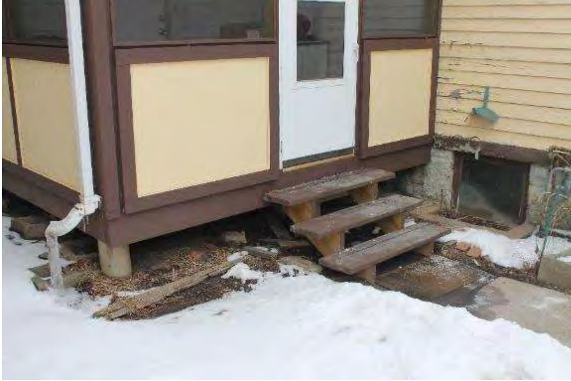
Photo 305: 410 1/2 East Washington Avenue, Exterior, facing north
