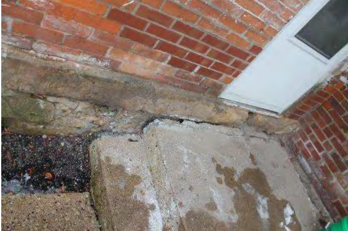
Photo 153: 402-408 East Washington Avenue, Exterior, facing west
