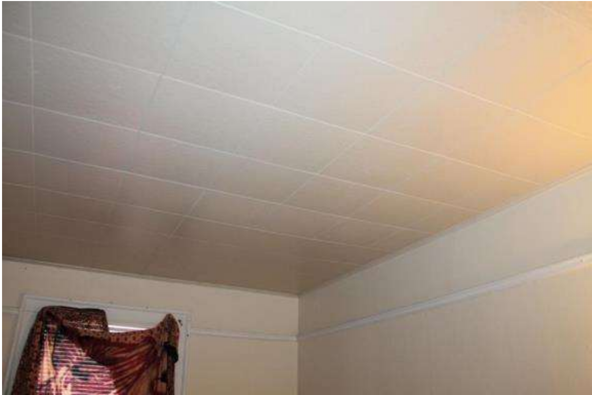
Photo 88: 8-10 North Franklin Street, Interior, second floor unit 2
