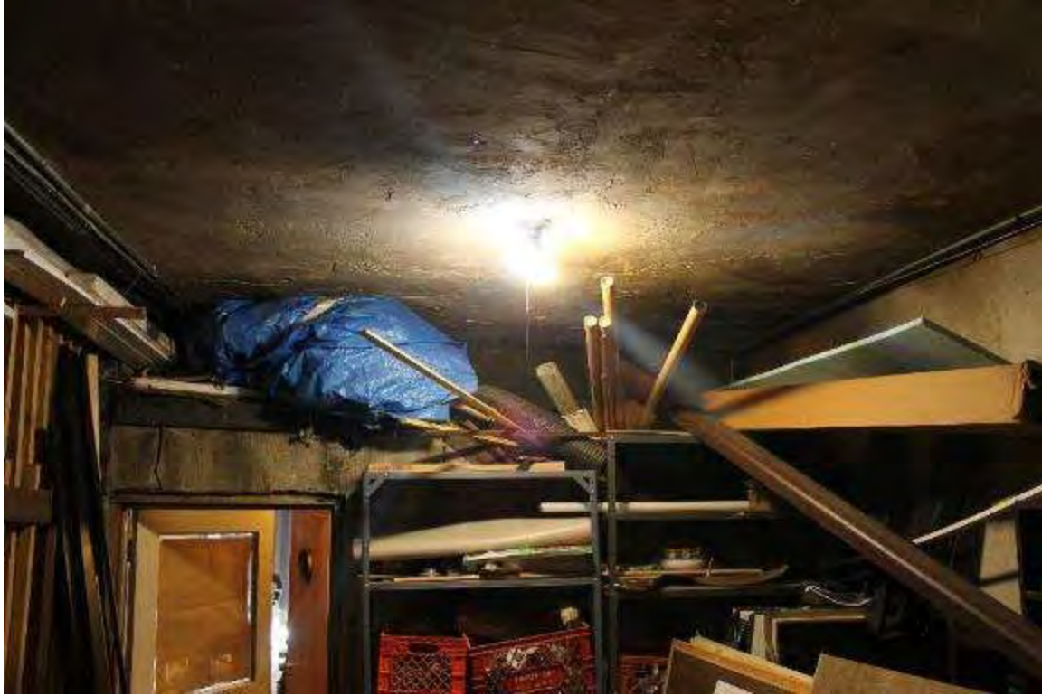
Photo 173: 402-408 East Washington Avenue, Interior, first floor commercial unit 2 garage
