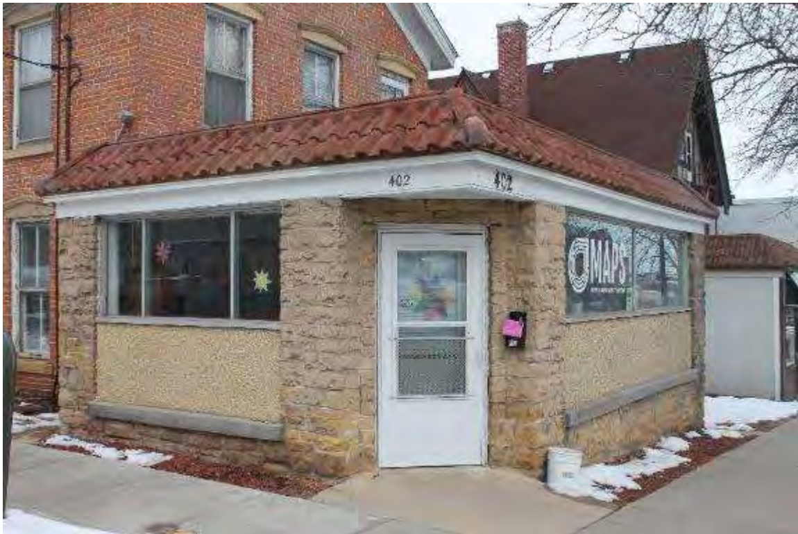
Photo 136: 402-408 East Washington Avenue, Exterior, facing north
