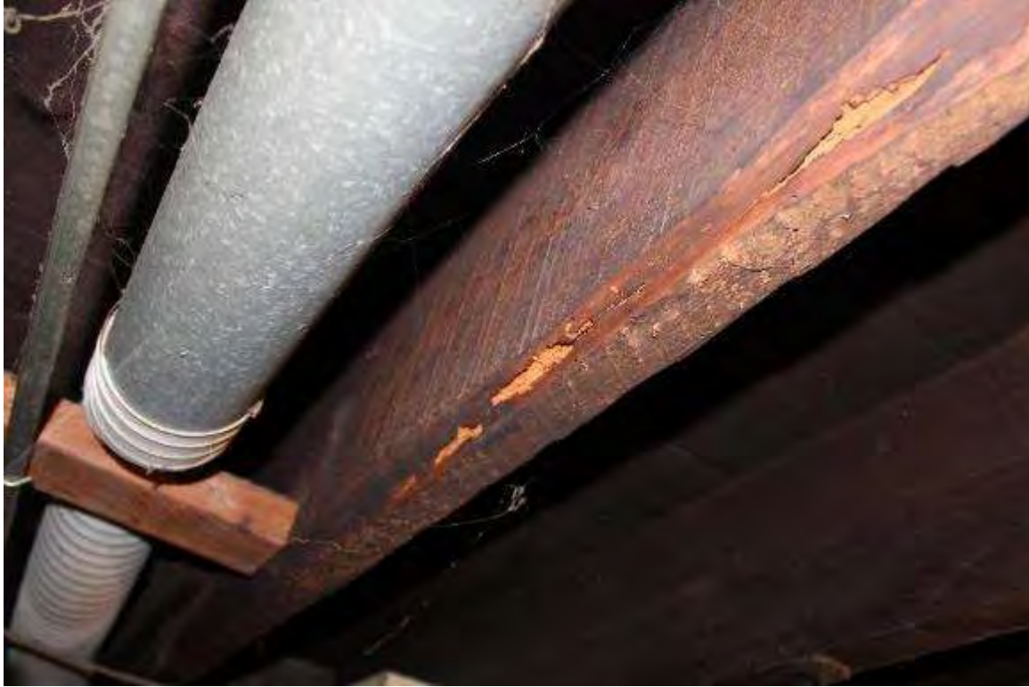
Photo 225: 402-408 East Washington Avenue, Interior, basement
