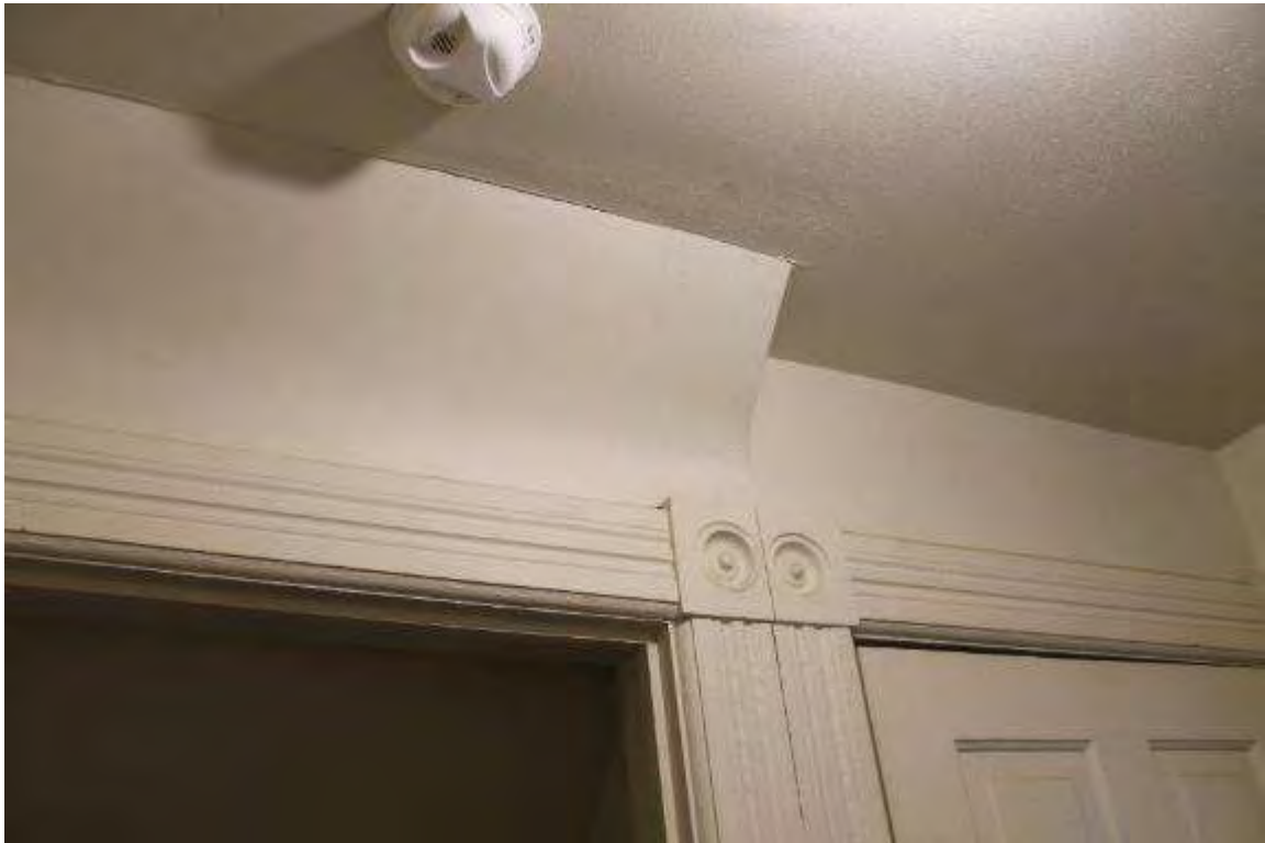
Photo 28: 9 North Hancock Street, Interior, first floor unit 1
