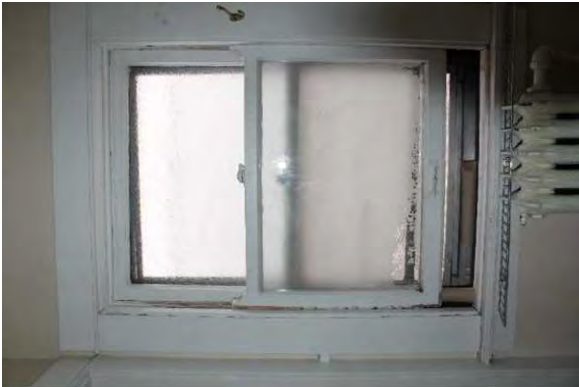
Photo 256: 410 East Washington Avenue, Interior, second floor toilet
