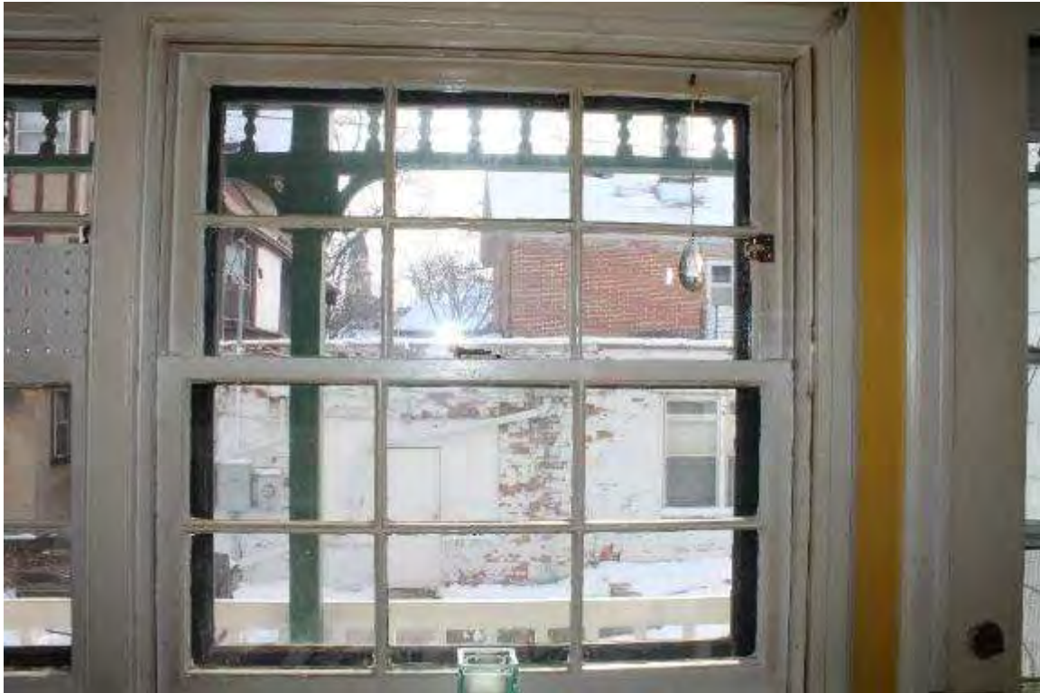
Photo 24: 9 North Hancock Street, Interior, first floor unit 1
