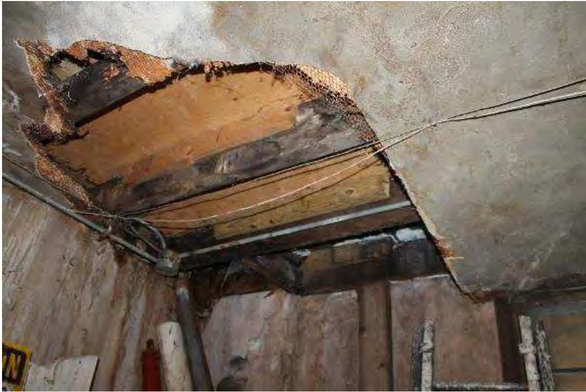
Photo 172: 402-408 East Washington Avenue, Interior, first floor commercial unit 2 garage
