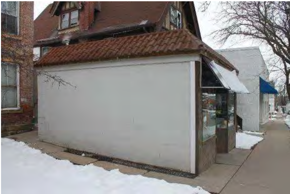
Photo 160: 402-408 East Washington Avenue, Exterior, facing northeast
