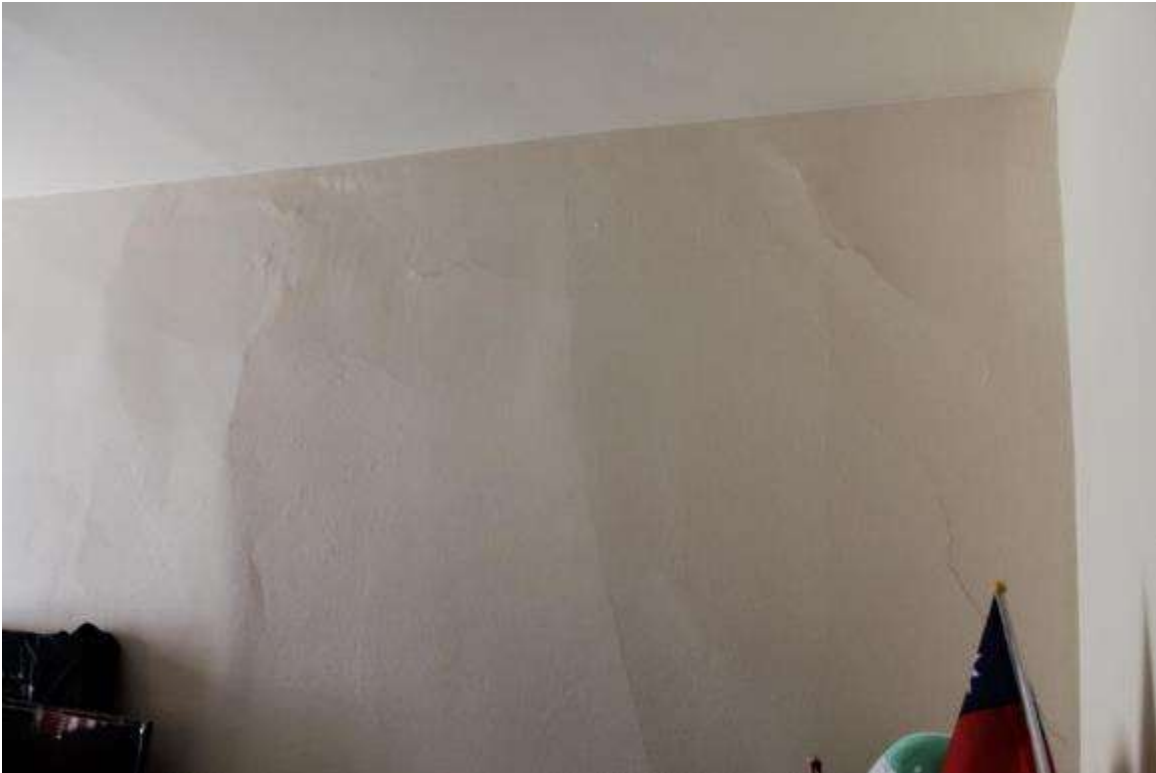
Photo 206: 402-408 East Washington Avenue, Interior, second floor unit 3
