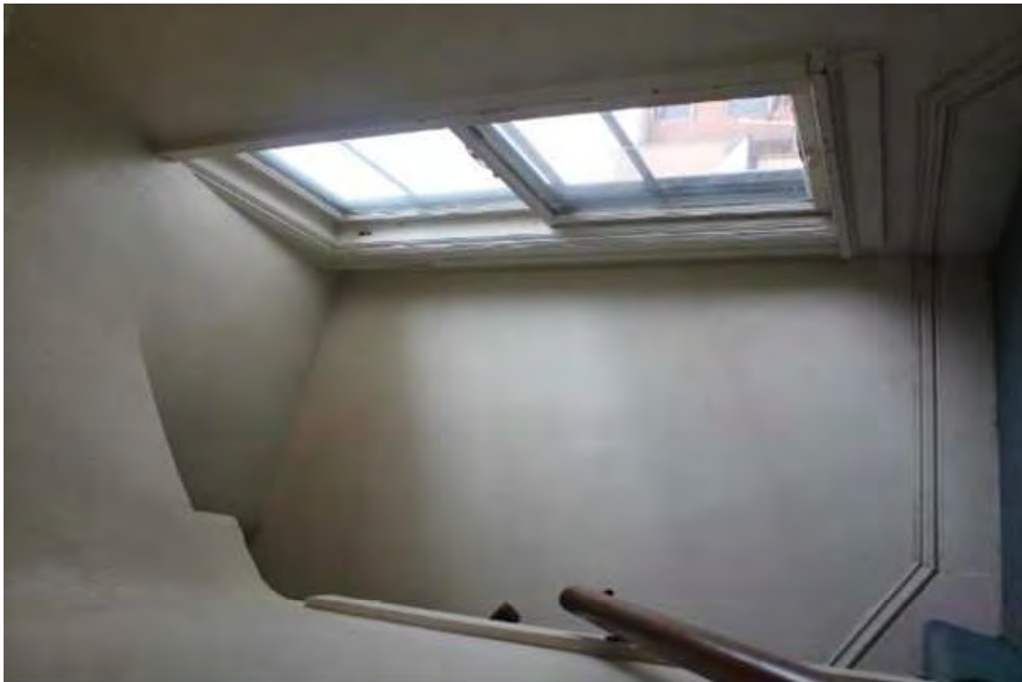
Photo 78: 8-10 North Franklin Street, Interior, second floor stairs
