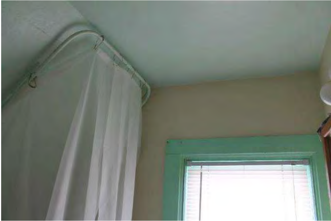
Photo 94: 8-10 North Franklin Street, Interior, third floor unit 3
