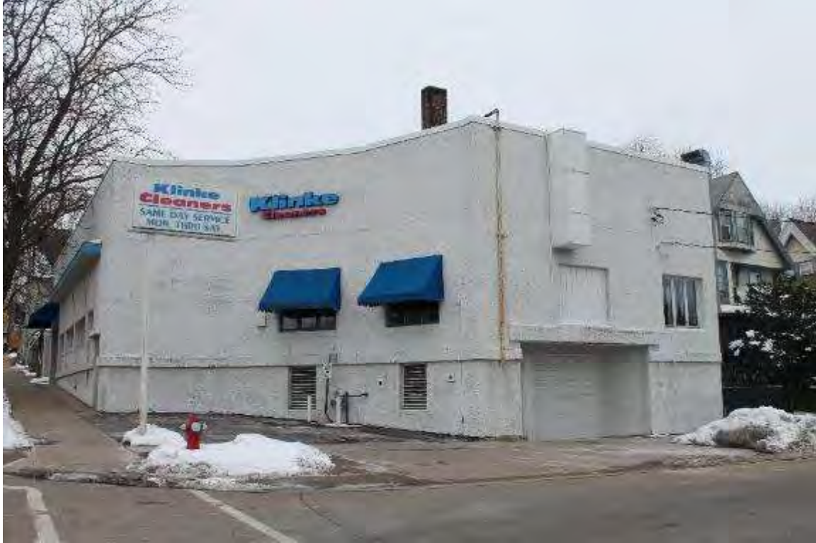
Photo 327: 412-414 East Washington Avenue, Exterior, facing west
