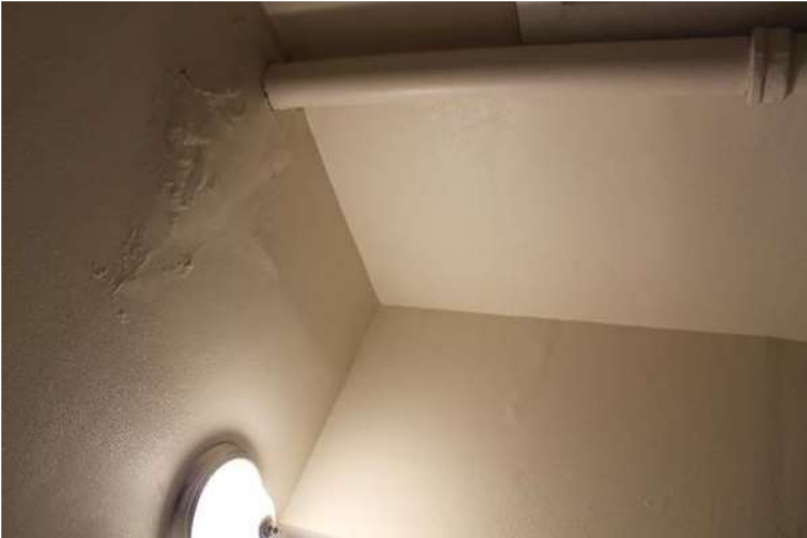
Photo 198: 402-408 East Washington Avenue, Interior, second floor unit 3
