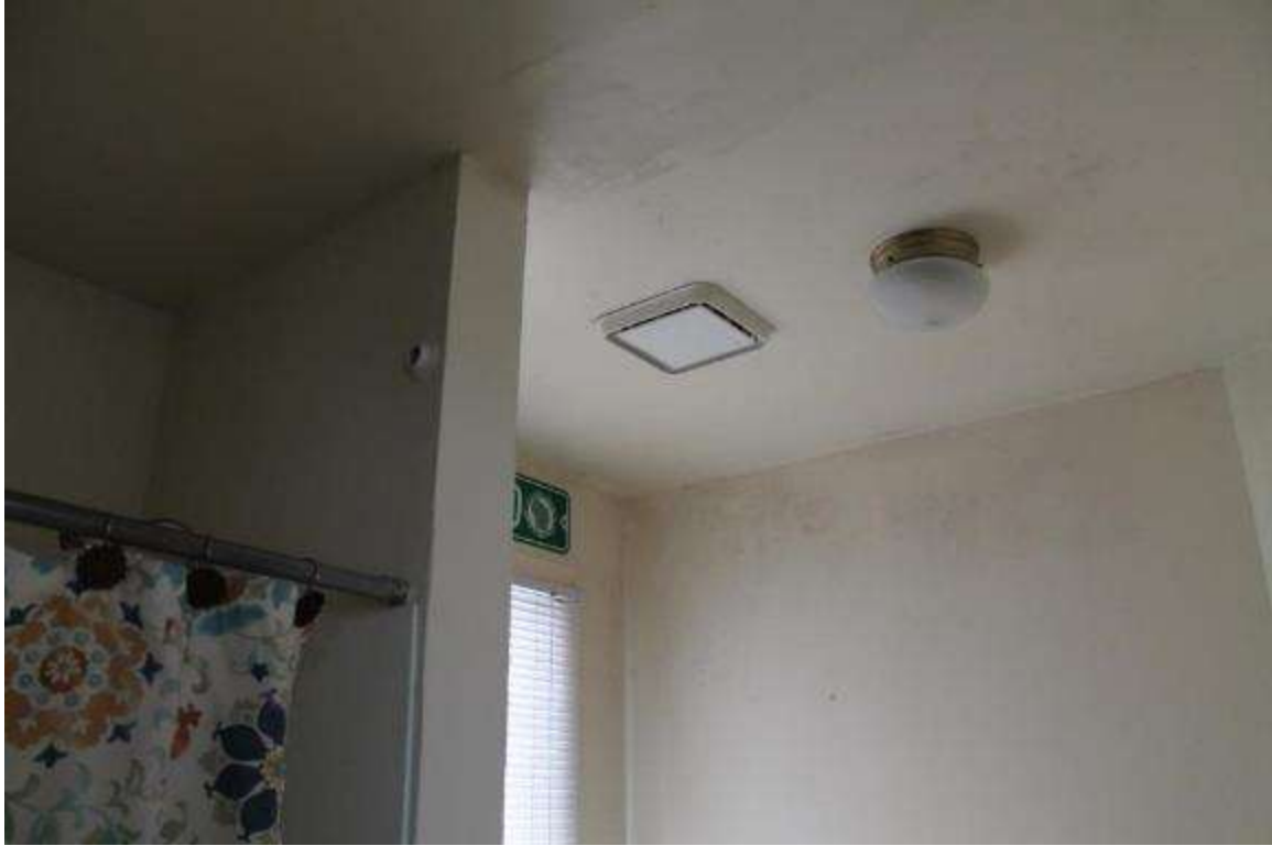
Photo 83: 8-10 North Franklin Street, Interior, second floor unit 2
