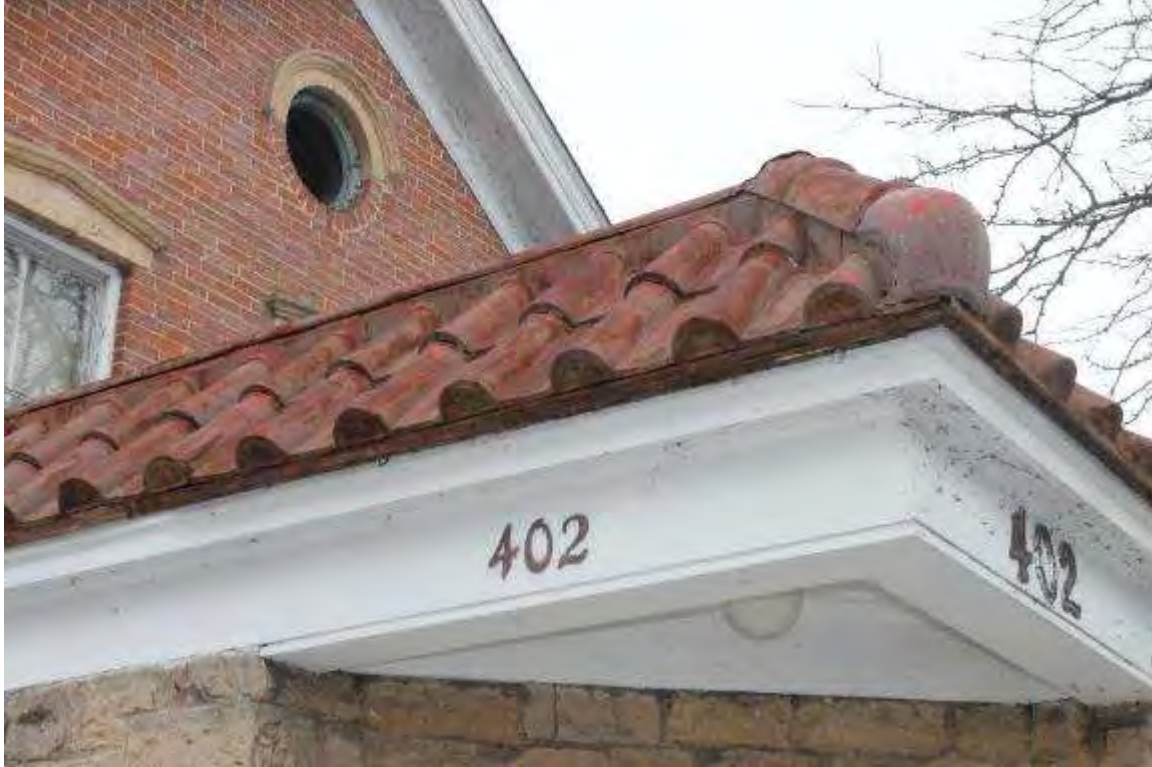
Photo 139: 402-408 East Washington Avenue, Exterior, facing north
