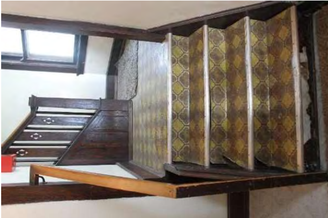
Photo 252: 410 East Washington Avenue, Interior, first floor stairwell
