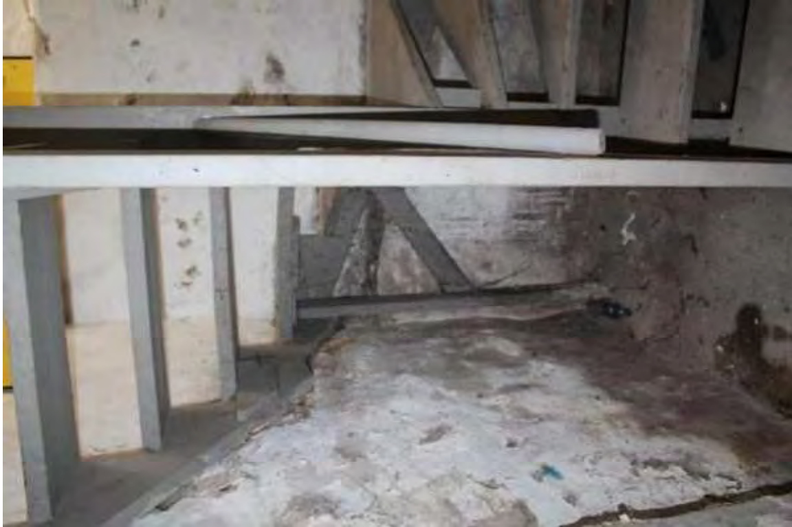
Photo 97: 8-10 North Franklin Street, Interior, basement
