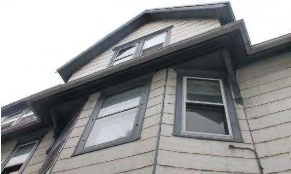
Photo 57: 8-10 North Franklin Street, Exterior, facing northwest
