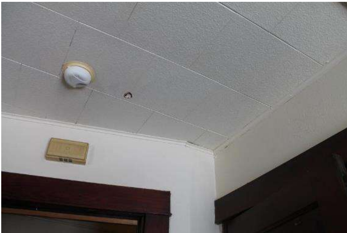
Photo 268: 410 East Washington Avenue, Interior, second floor unit 4
