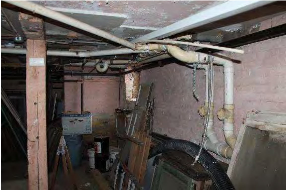
Photo 48: 9 North Hancock Street, Interior, basement
