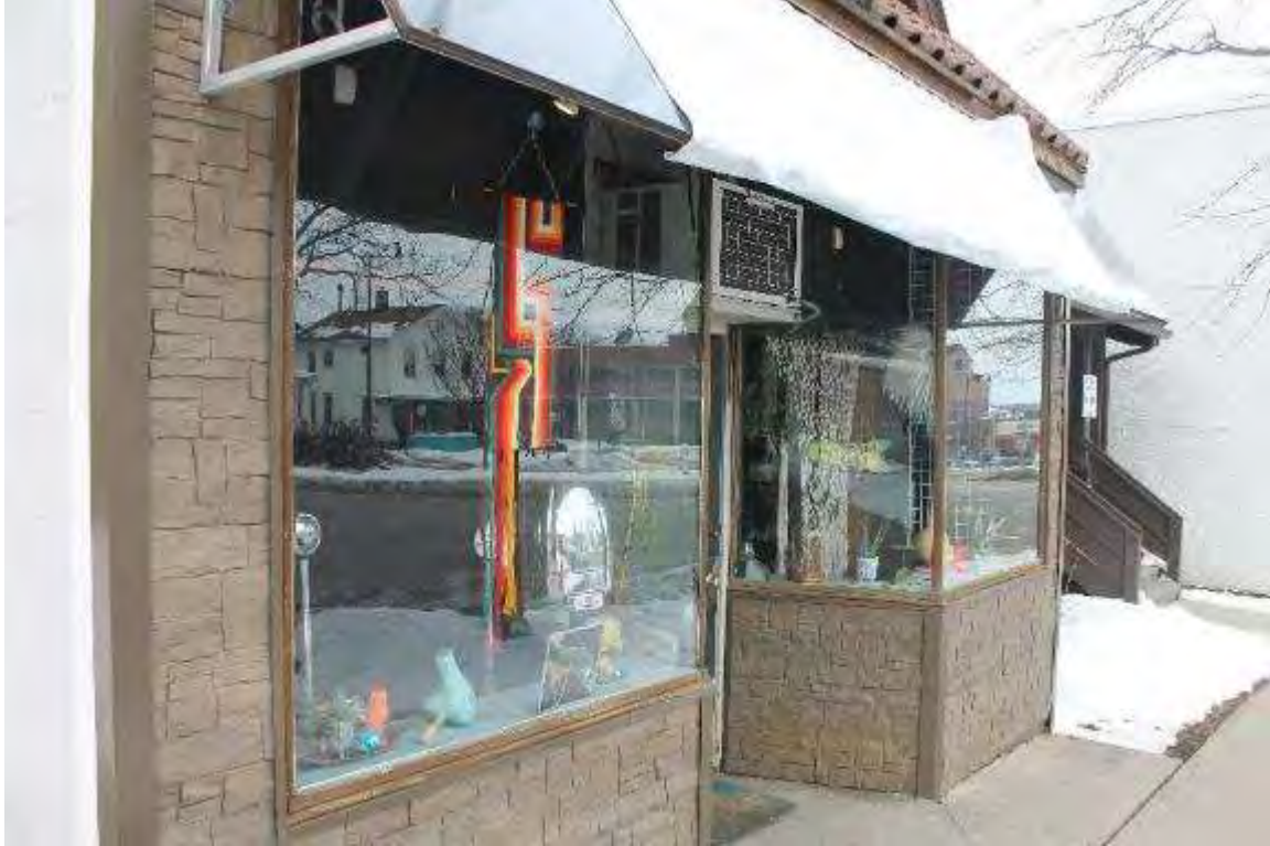
Photo 161: 402-408 East Washington Avenue, Exterior, facing north
