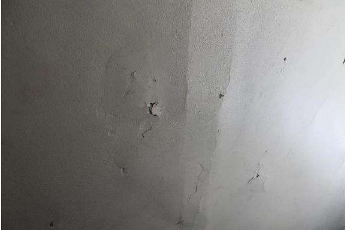
Photo 127: 12 North Franklin Street, Interior, second floor unit 2
