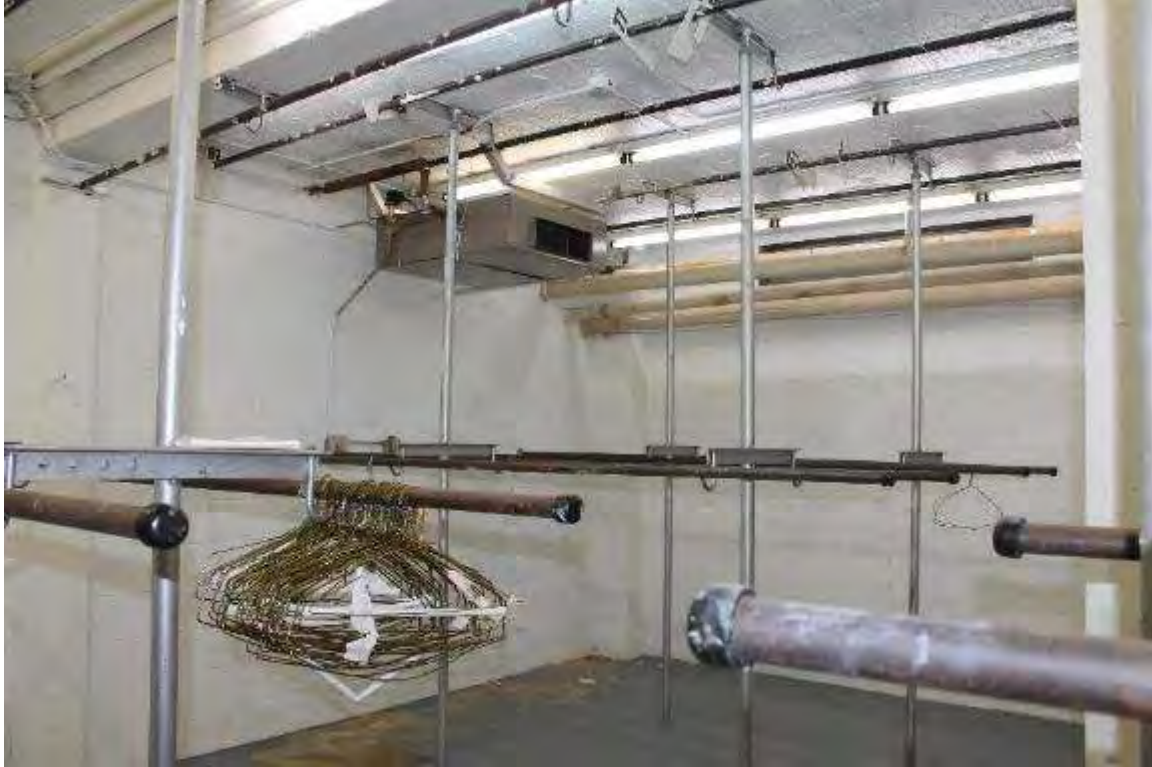
Photo 367: 412-414 East Washington Avenue, Interior, lower level storage space
