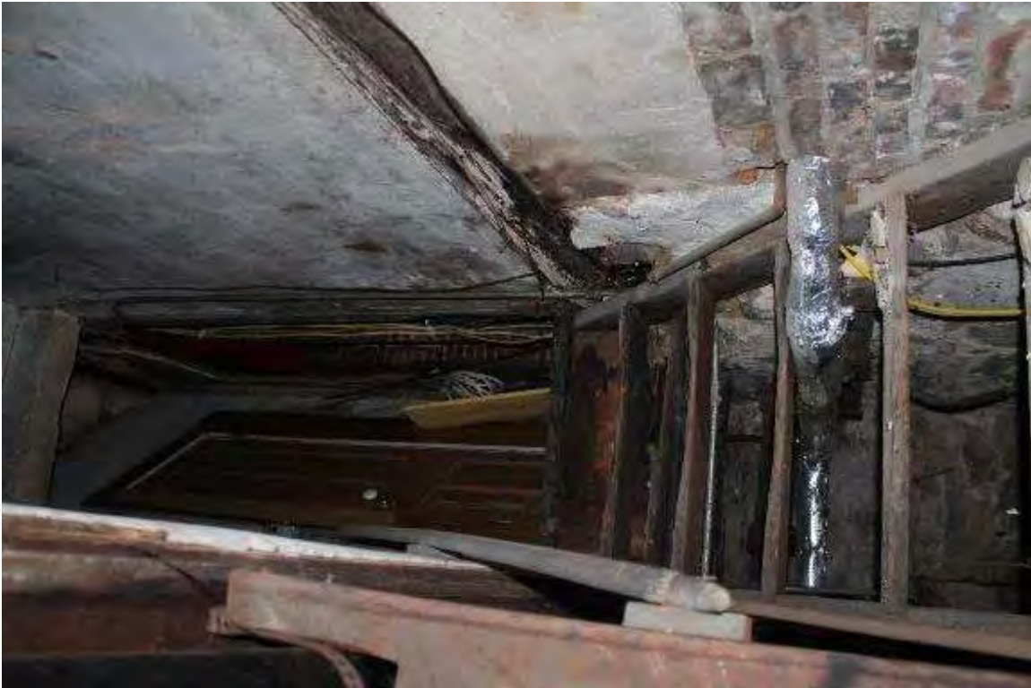
Photo 224: 402-408 East Washington Avenue, Interior, basement
