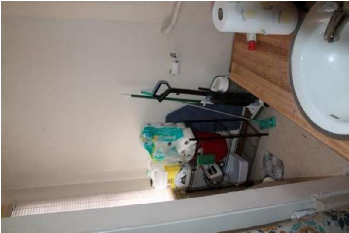
Photo 82: 8-10 North Franklin Street, Interior, second floor unit 2
