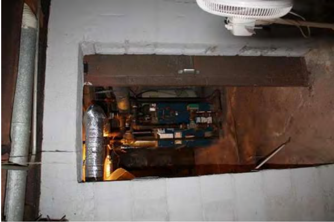
Photo 219: 402-408 East Washington Avenue, Interior, basement
