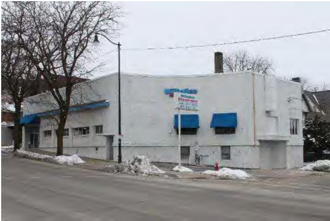
Photo 326: 412-414 East Washington Avenue, Exterior, facing west
