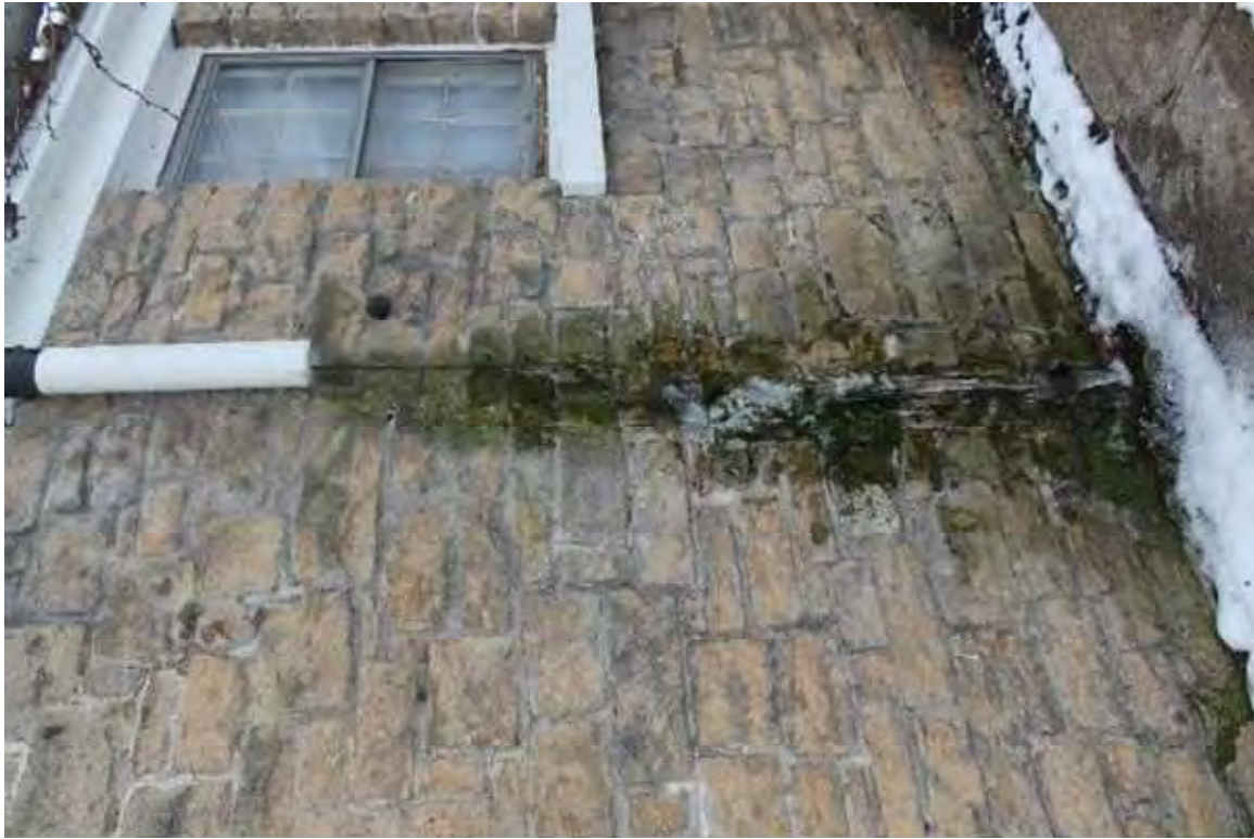
Photo 152: 402-408 East Washington Avenue, Exterior, facing west
