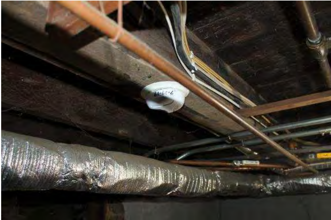
Photo 218: 402-408 East Washington Avenue, Interior, basement
