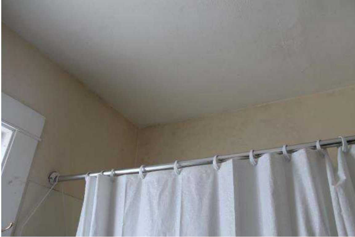
Photo 255: 410 East Washington Avenue, Interior, second floor toilet
