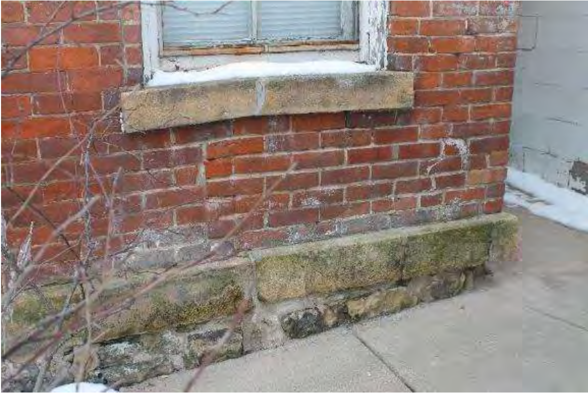
Photo 156: 402-408 East Washington Avenue, Exterior, facing north
