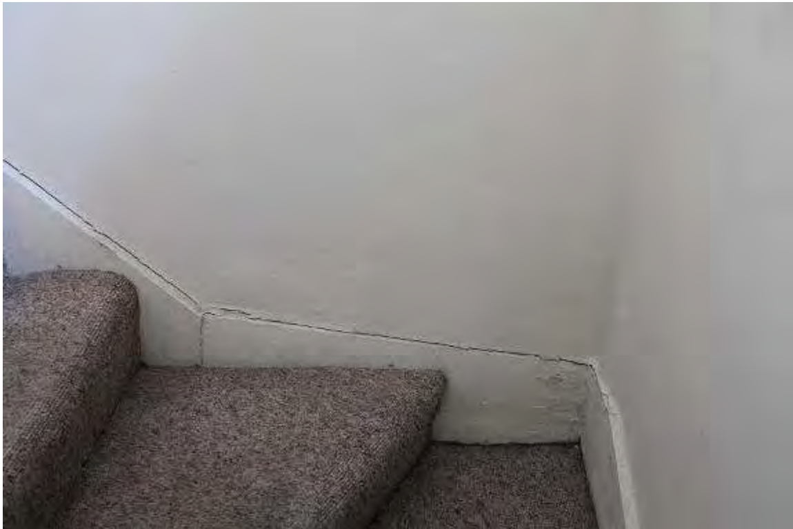
Photo 274: 410 East Washington Avenue, Interior, third floor stairwell
