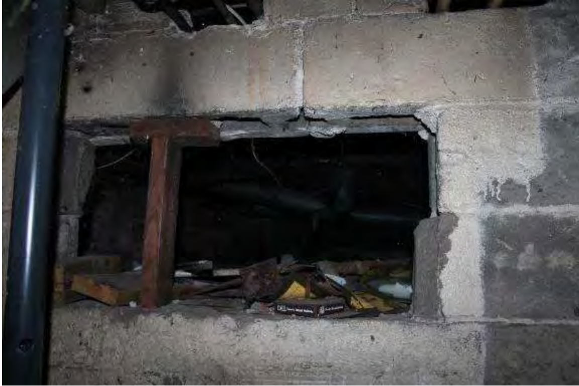
Photo 325: 410 1/2 East Washington Avenue, Interior, basement
