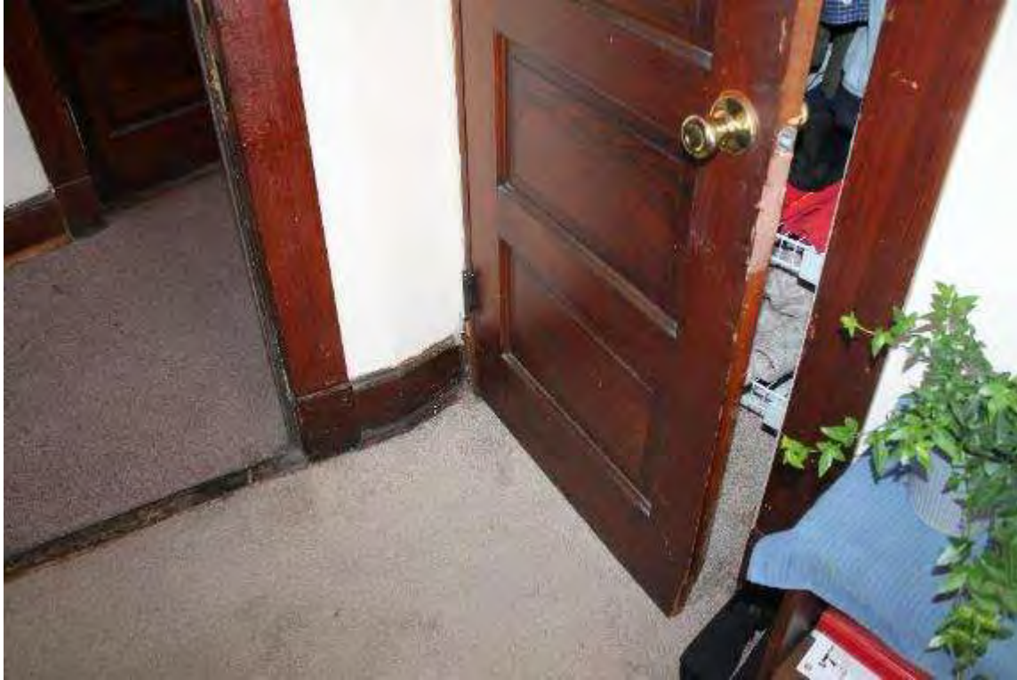
Photo 267: 410 East Washington Avenue, Interior, second floor unit 4
