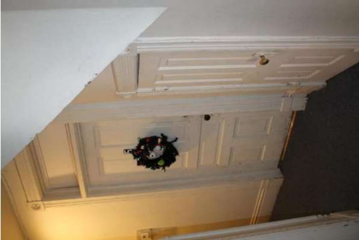
Photo 33: 9 North Hancock Street, Interior, second floor hallway
