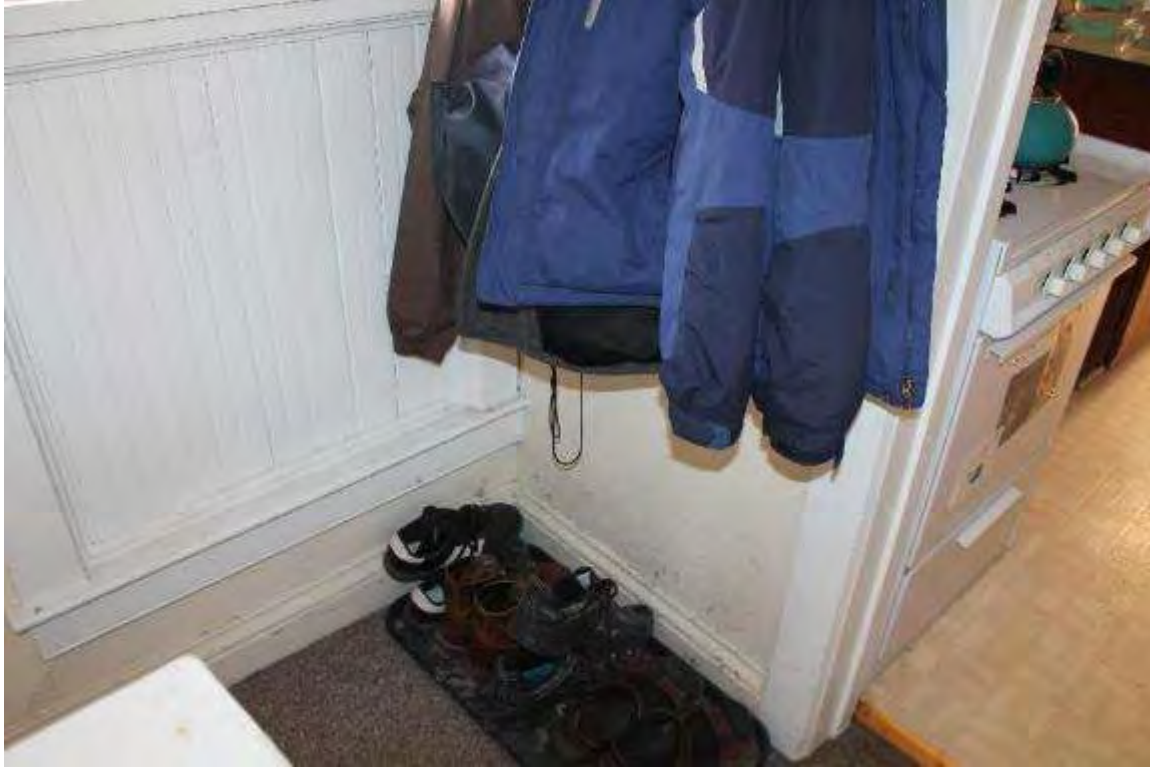
Photo 323: 410 1/2 East Washington Avenue, Interior, second floor unit 2
