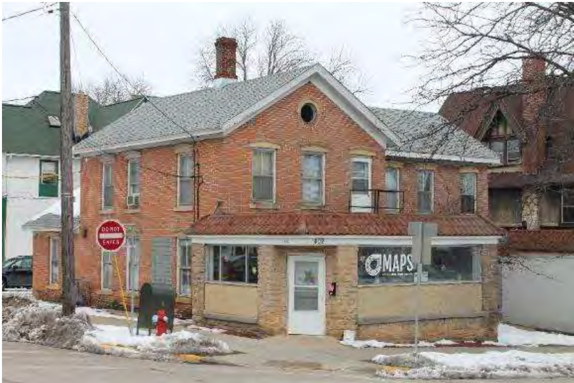
Photo 132: 402-408 East Washington Avenue, Exterior, facing north
