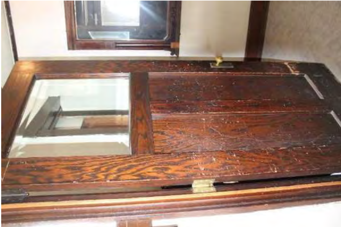
Photo 250: 410 East Washington Avenue, Interior, first floor front entry
