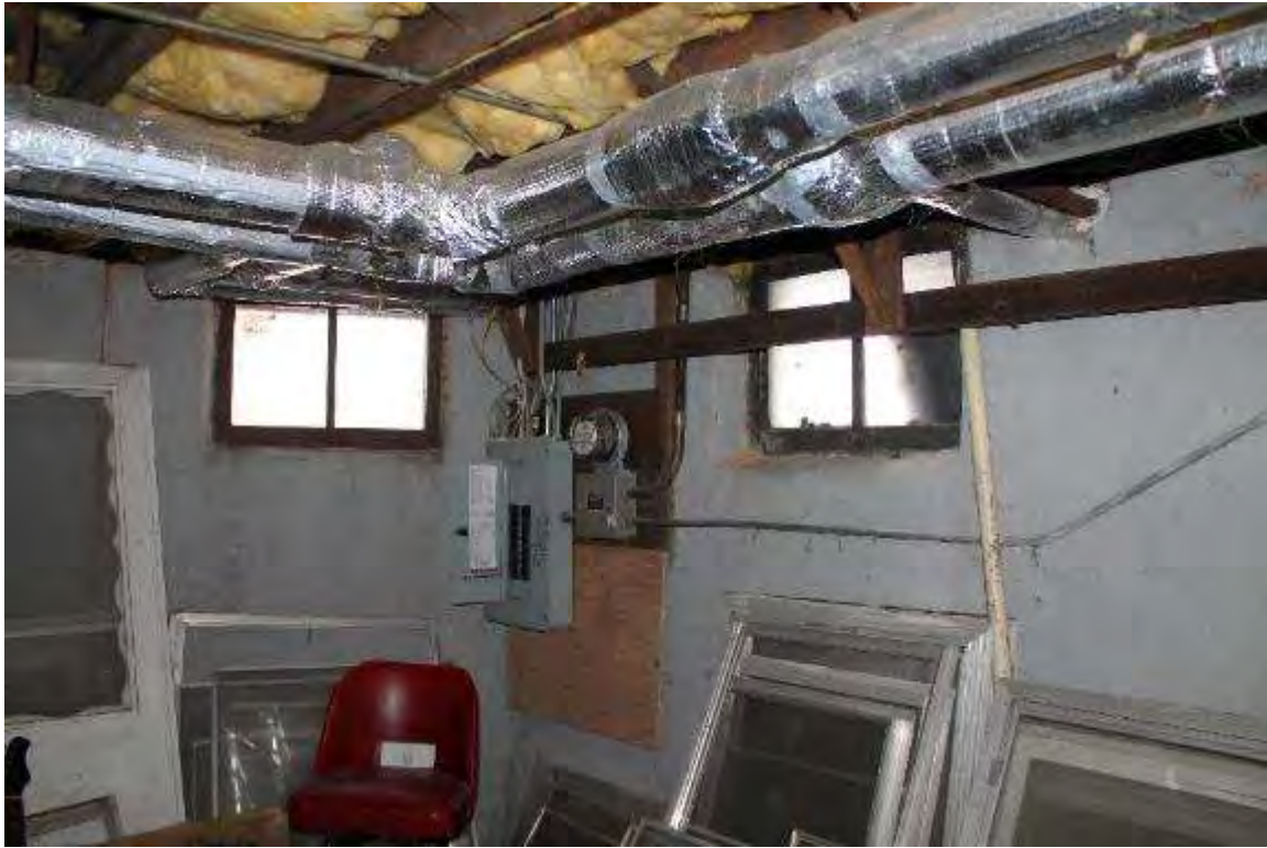
Photo 290: 410 East Washington Avenue, Interior, basement
