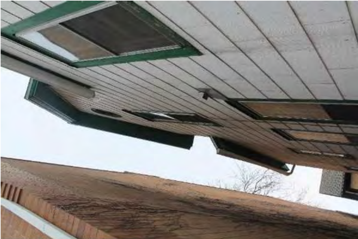
Photo 12: 9 North Hancock Street, Exterior, facing east
