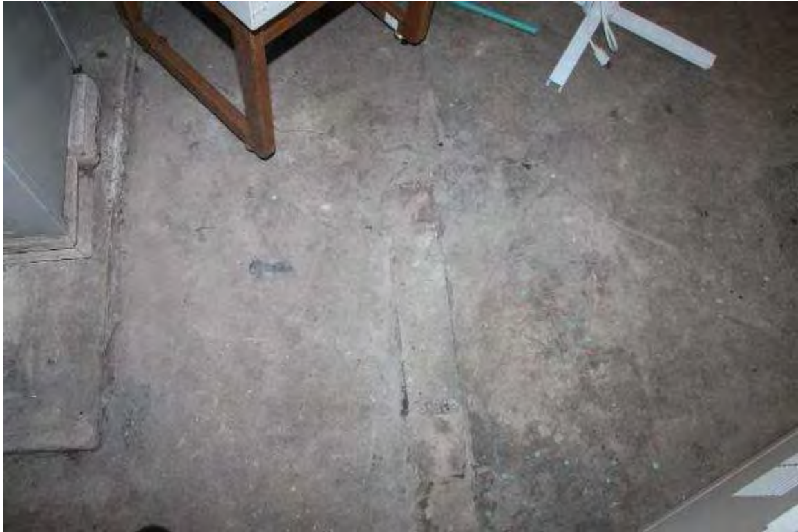
Photo 100: 8-10 North Franklin Street, Interior, basement
