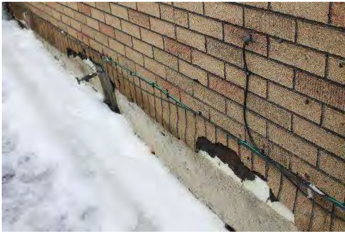
Photo 106: 12 North Franklin Street, Exterior, facing west
