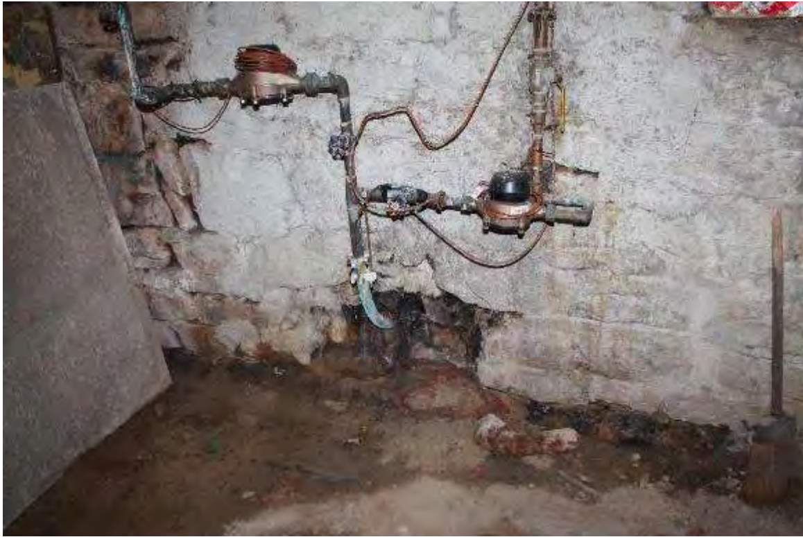
Photo 222: 402-408 East Washington Avenue, Interior, basement
