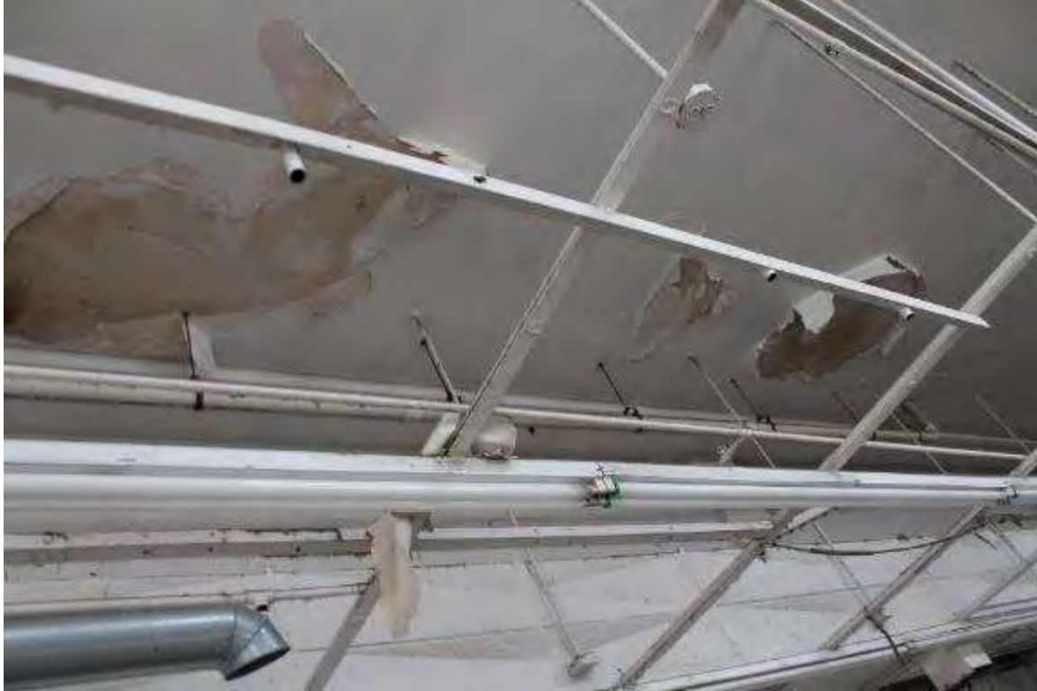
Photo 355: 412-414 East Washington Avenue, Interior, first floor processing space
