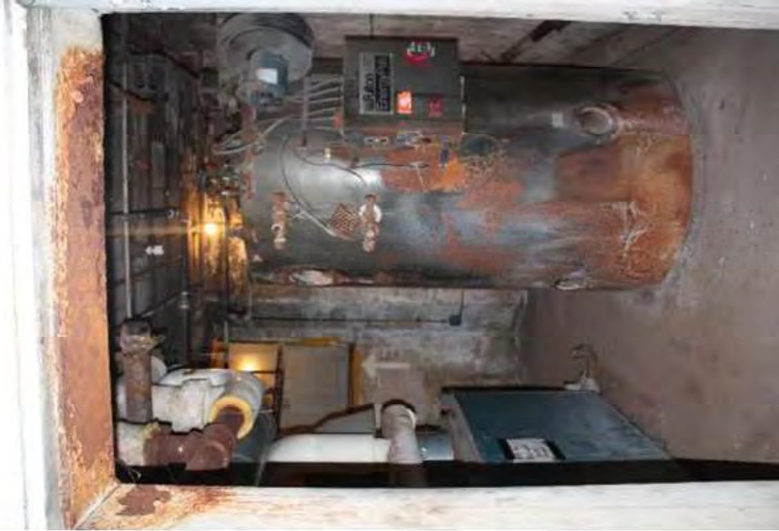
Photo 369: 412-414 East Washington Avenue, Interior, lower level storage space
