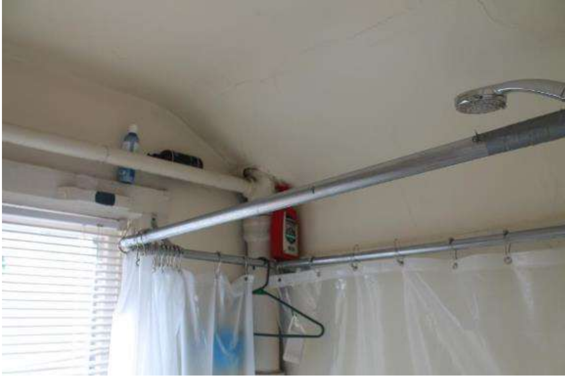
Photo 319: 410 1/2 East Washington Avenue, Interior, second floor unit 2
