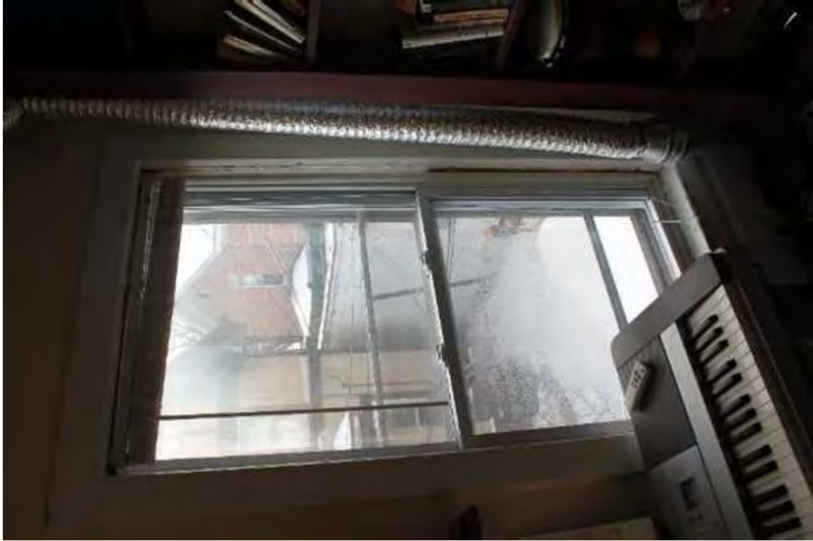
Photo 321: 410 1/2 East Washington Avenue, Interior, second floor unit 2
