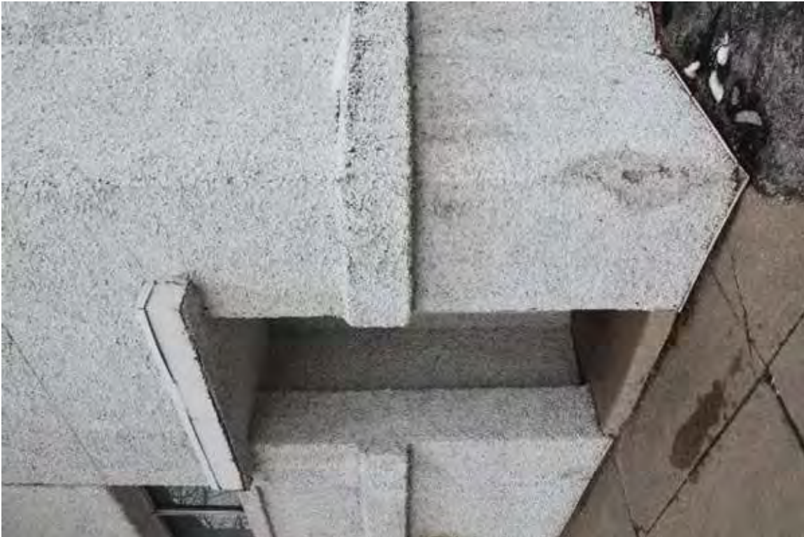
Photo 336: 412-414 East Washington Avenue, Exterior, facing west
