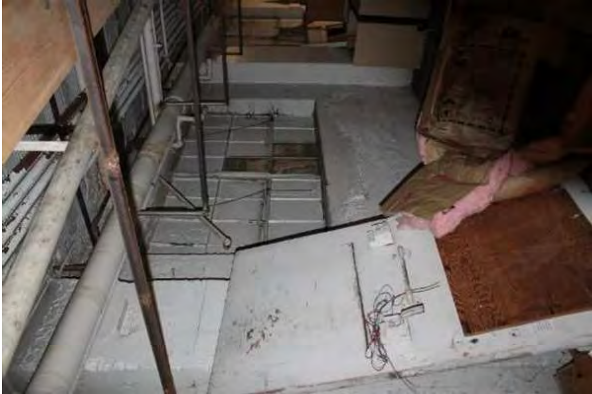
Photo 363: 412-414 East Washington Avenue, Interior, lower level storage space
