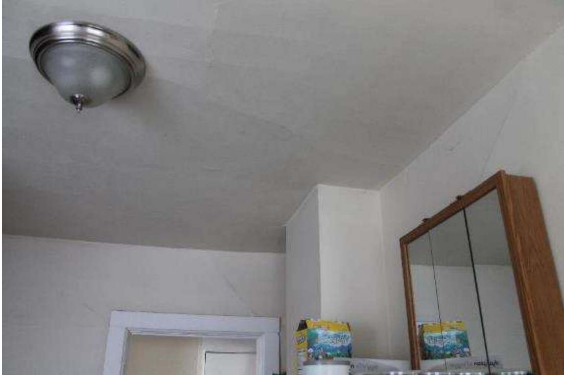
Photo 203: 402-408 East Washington Avenue, Interior, second floor unit 3
