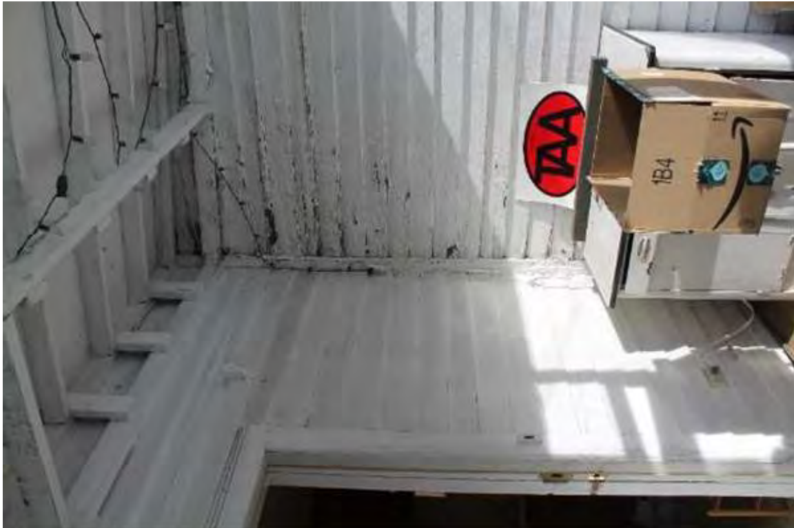
Photo 306: 410 1/2 East Washington Avenue, Exterior, facing northeast
