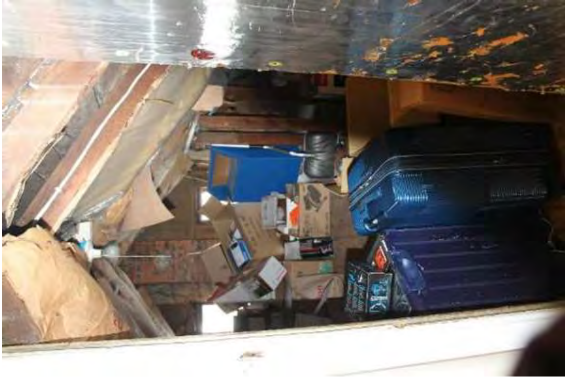
Photo 201: 402-408 East Washington Avenue, Interior, second floor unit 3
