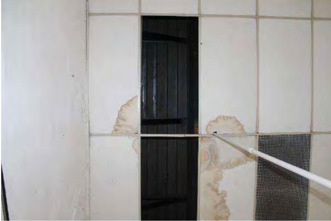
Photo 349: 412-414 East Washington Avenue, Interior, first floor commercial space
