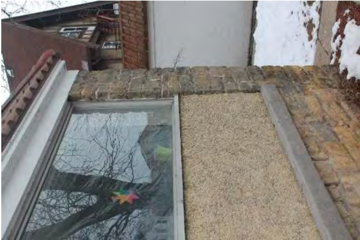
Photo 138: 402-408 East Washington Avenue, Exterior, facing north
