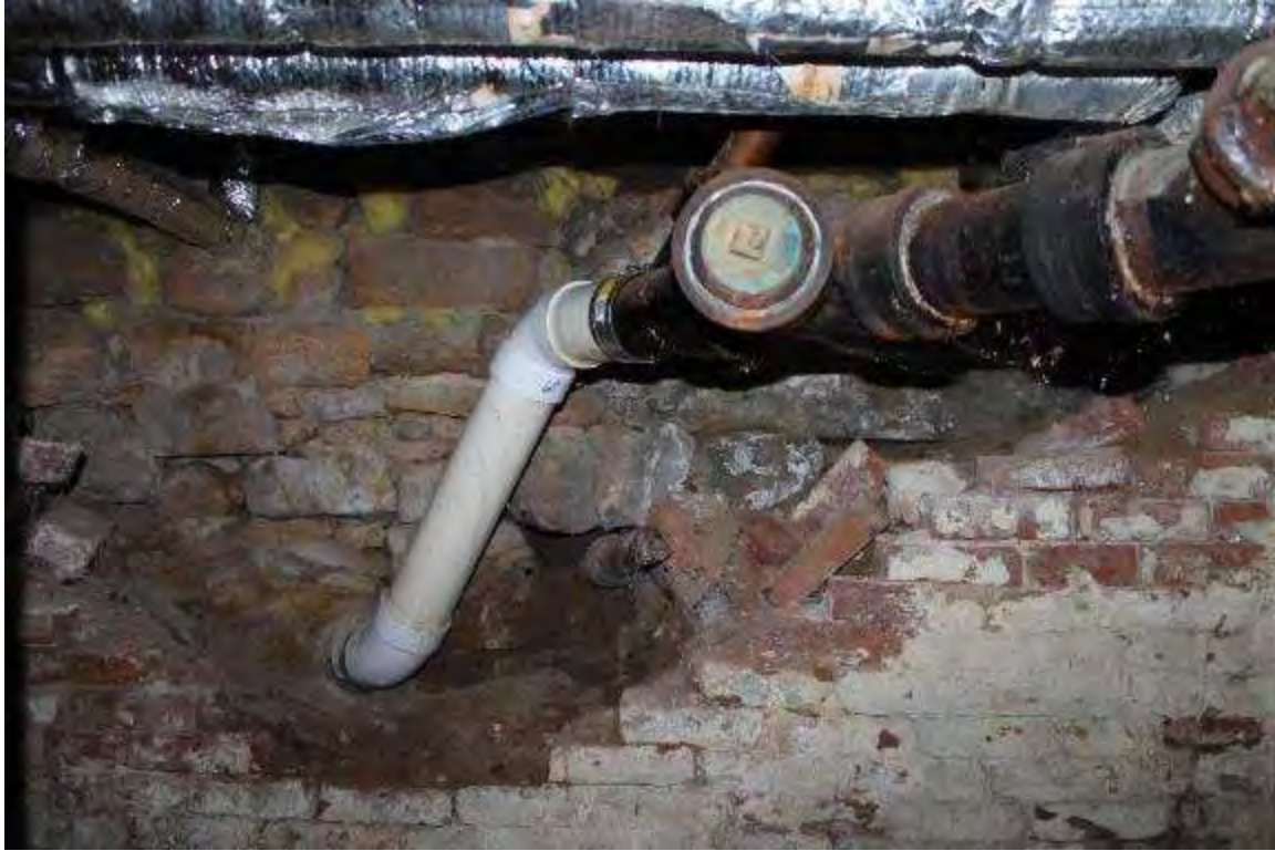
Photo 129: 12 North Franklin Street, Interior, basement
