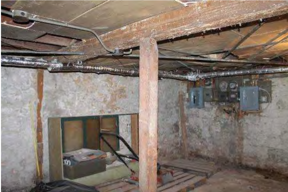
Photo 221: 402-408 East Washington Avenue, Interior, basement
