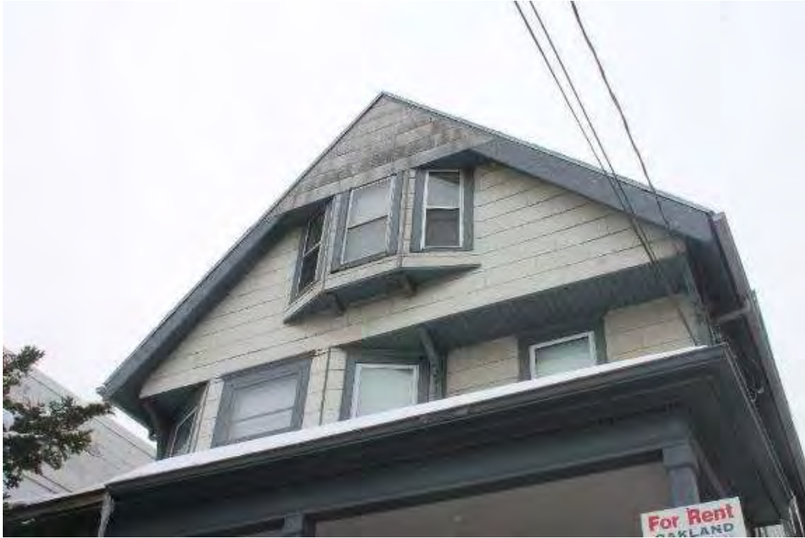
Photo 53: 8-10 North Franklin Street, Exterior, facing south
