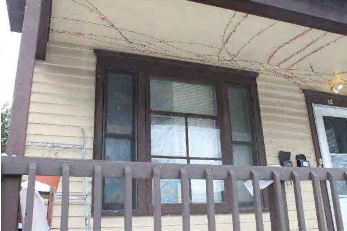
Photo 104: 12 North Franklin Street, Exterior, facing southwest
