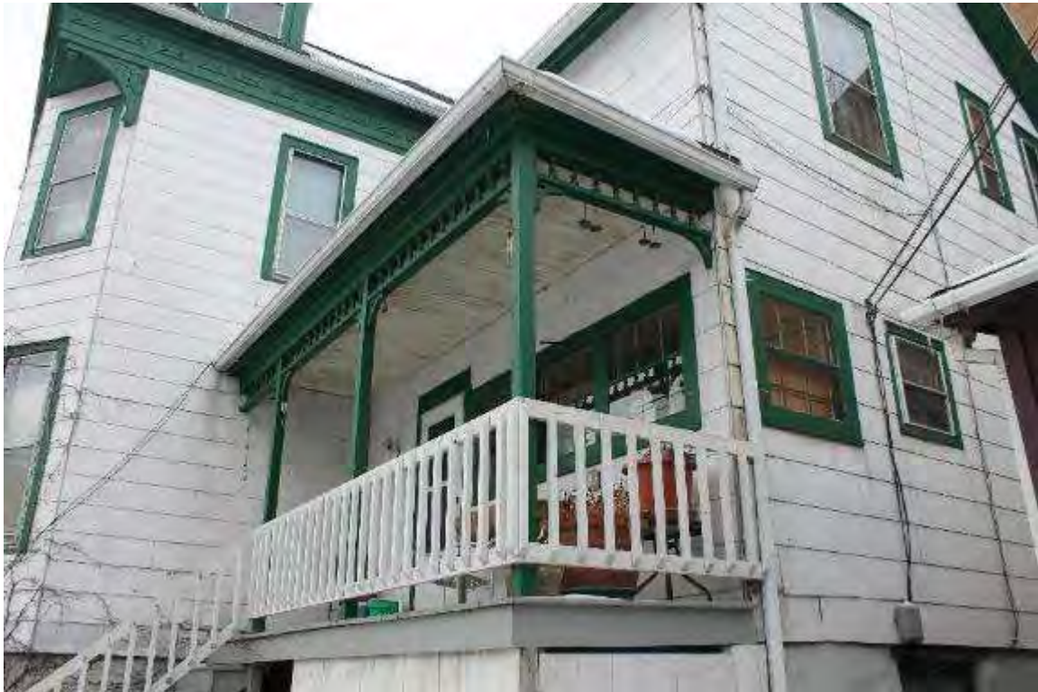
Photo 6: 9 North Hancock Street, Exterior, facing west
