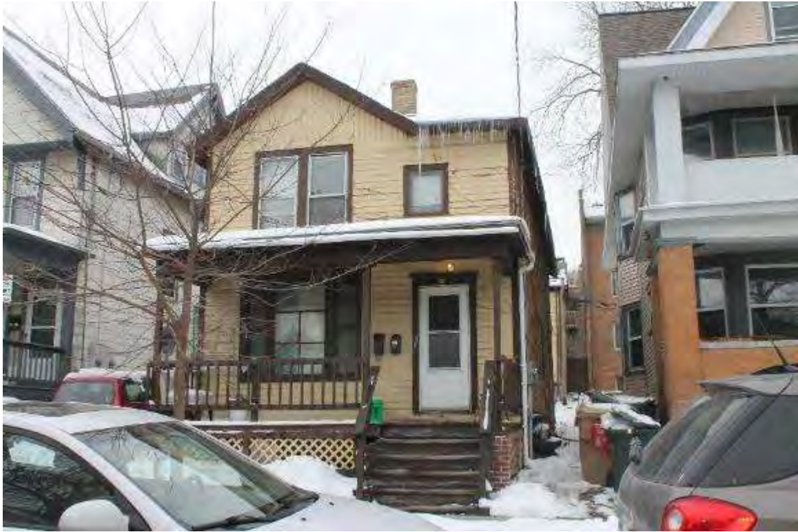
Photo 101: 12 North Franklin Street, Exterior, facing southwest
