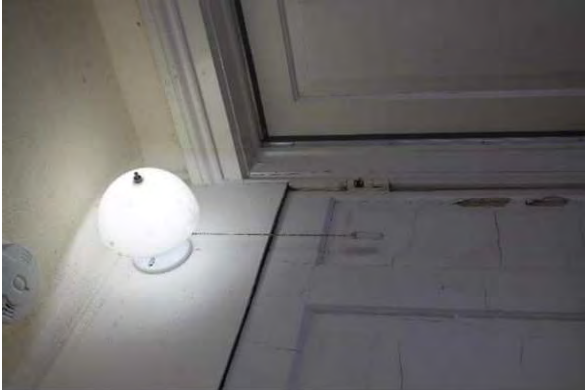
Photo 313: 410 1/2 East Washington Avenue, Interior, first floor entryway
