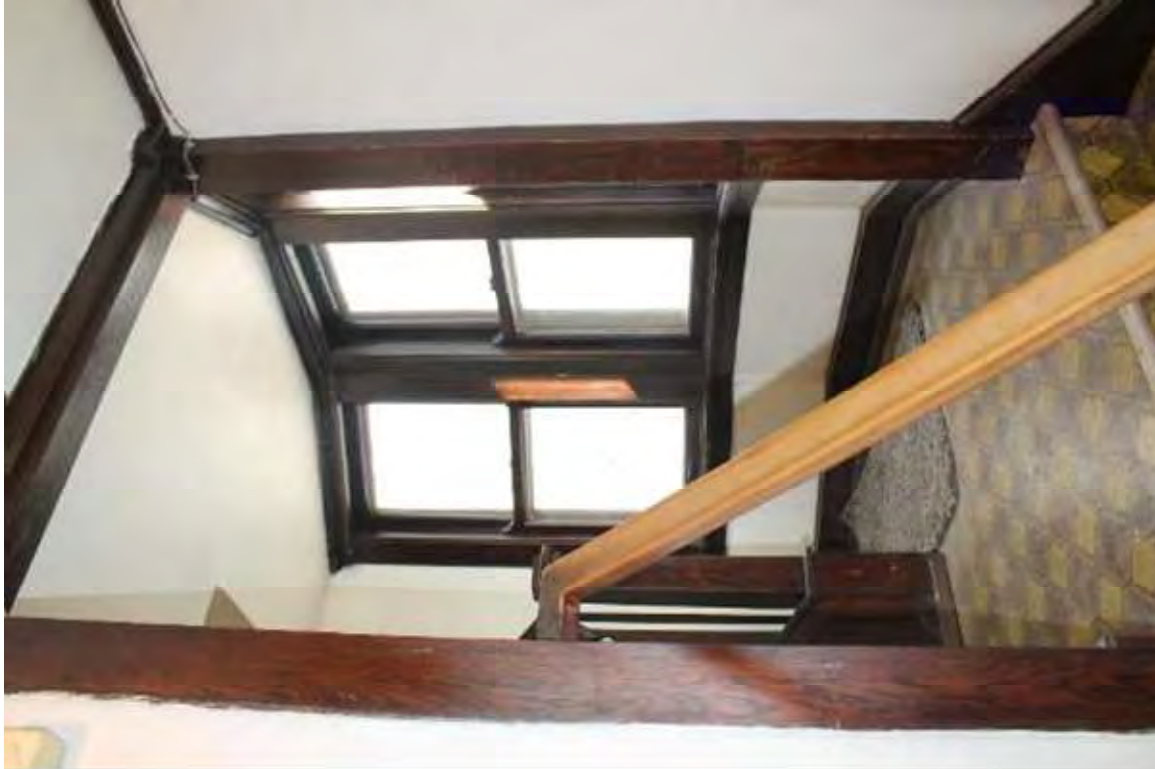
Photo 253: 410 East Washington Avenue, Interior, first floor stairwell
