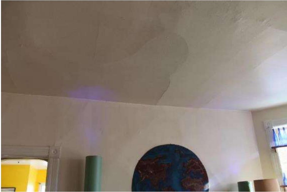
Photo 21: 9 North Hancock Street, Interior, first floor unit 1
