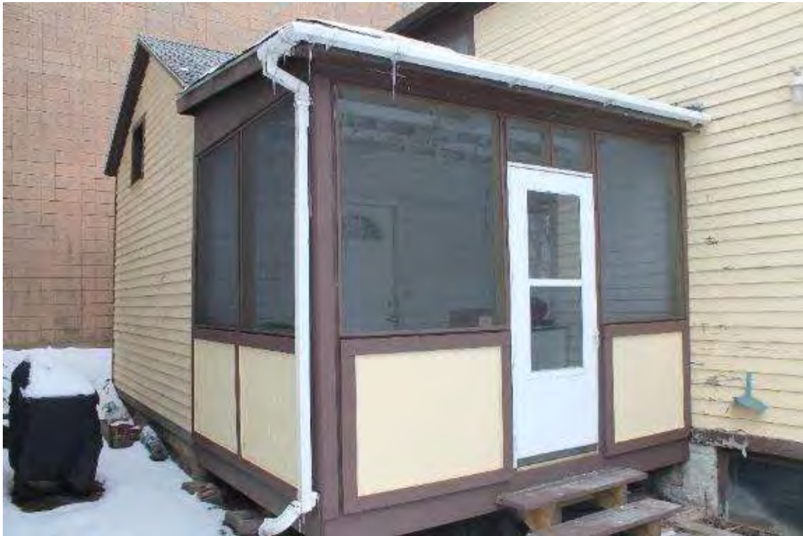
Photo 304: 410 1/2 East Washington Avenue, Exterior, facing north
