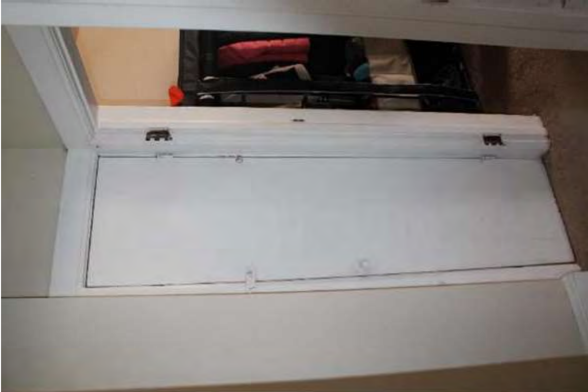
Photo 205: 402-408 East Washington Avenue, Interior, second floor unit 3
