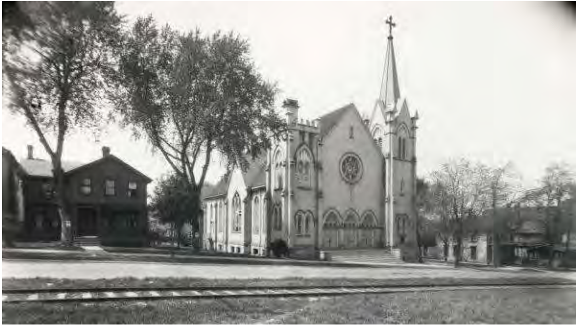
Photograph of St. John's Lutheran Church taken from the south, 1918. On file at the Wisconsin Historical Society Library and Archives. The house across Hancock Street on the left side of the photo are the subjects of this report.
