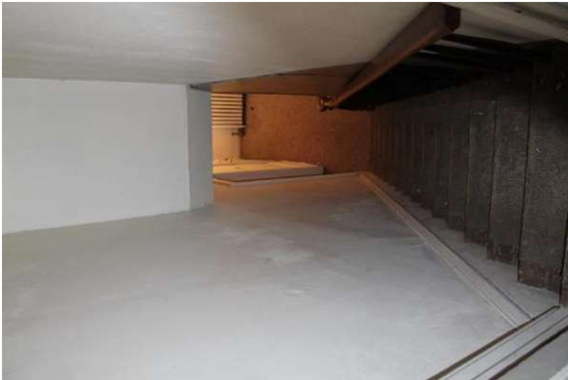
Photo 196: 402-408 East Washington Avenue, Interior, second floor stairs
