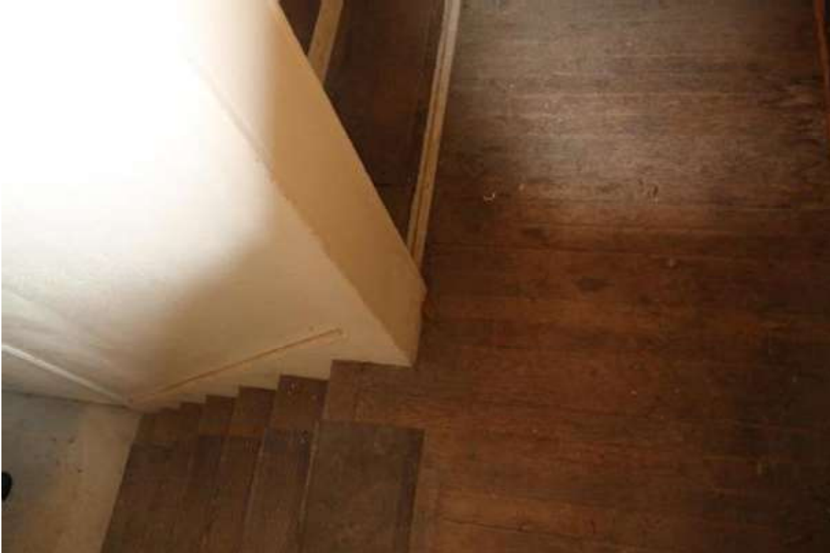
Photo 29: 9 North Hancock Street, Interior, first floor back stairs
