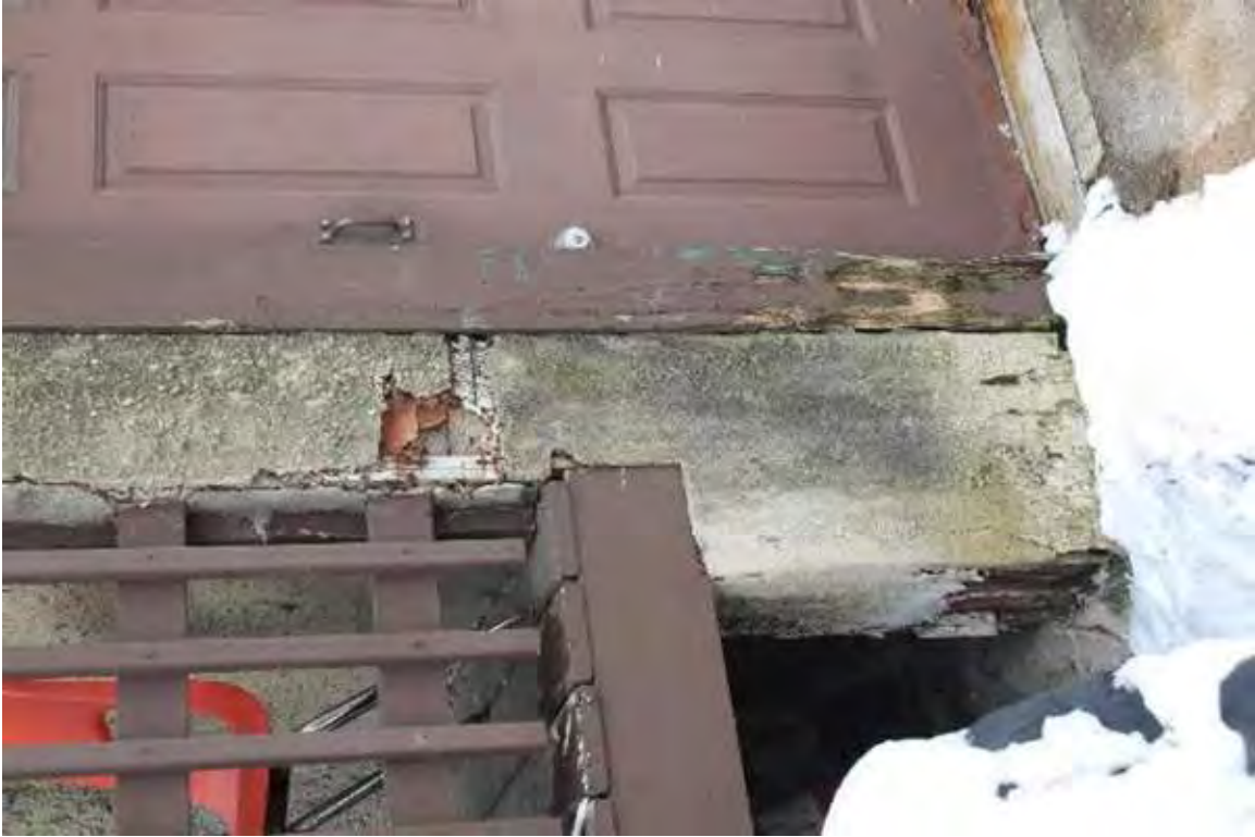
Photo 243: 410 East Washington Avenue, Exterior, facing south
