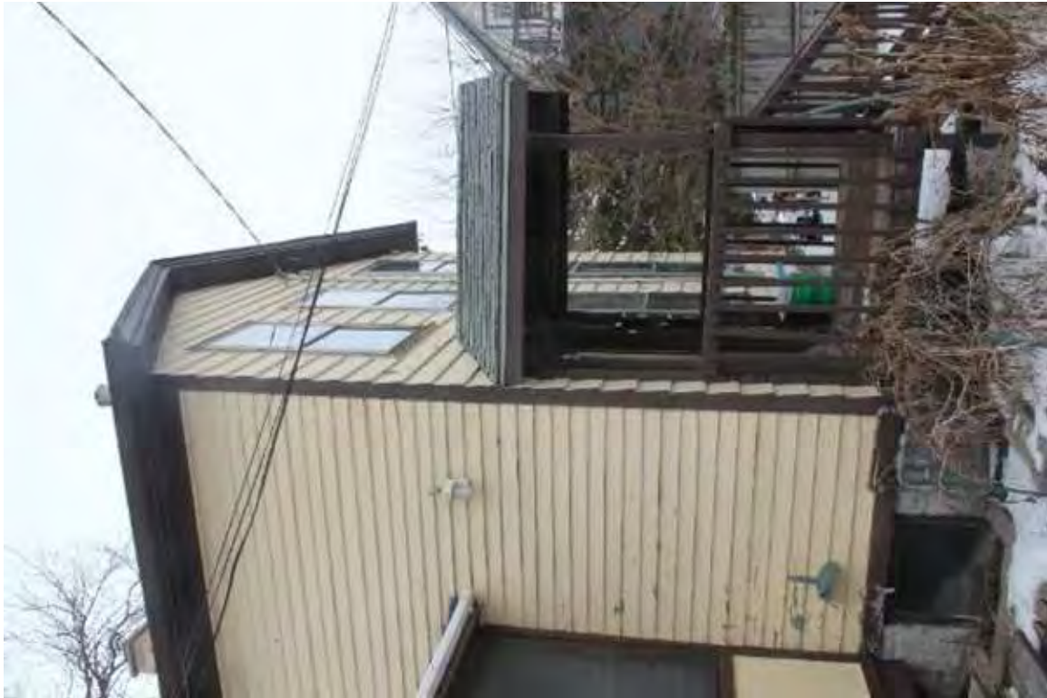
Photo 300: 410 1/2 East Washington Avenue, Exterior, facing northeast
