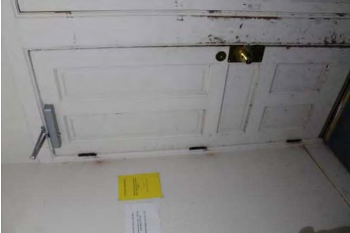
Photo 95: 8-10 North Franklin Street, Interior, third floor unit 3
