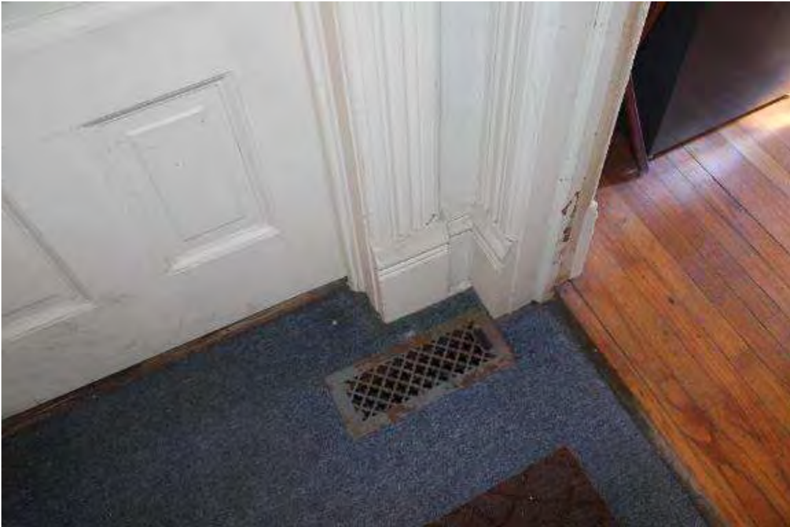
Photo 18: 9 North Hancock Street, Interior, first floor unit 1
