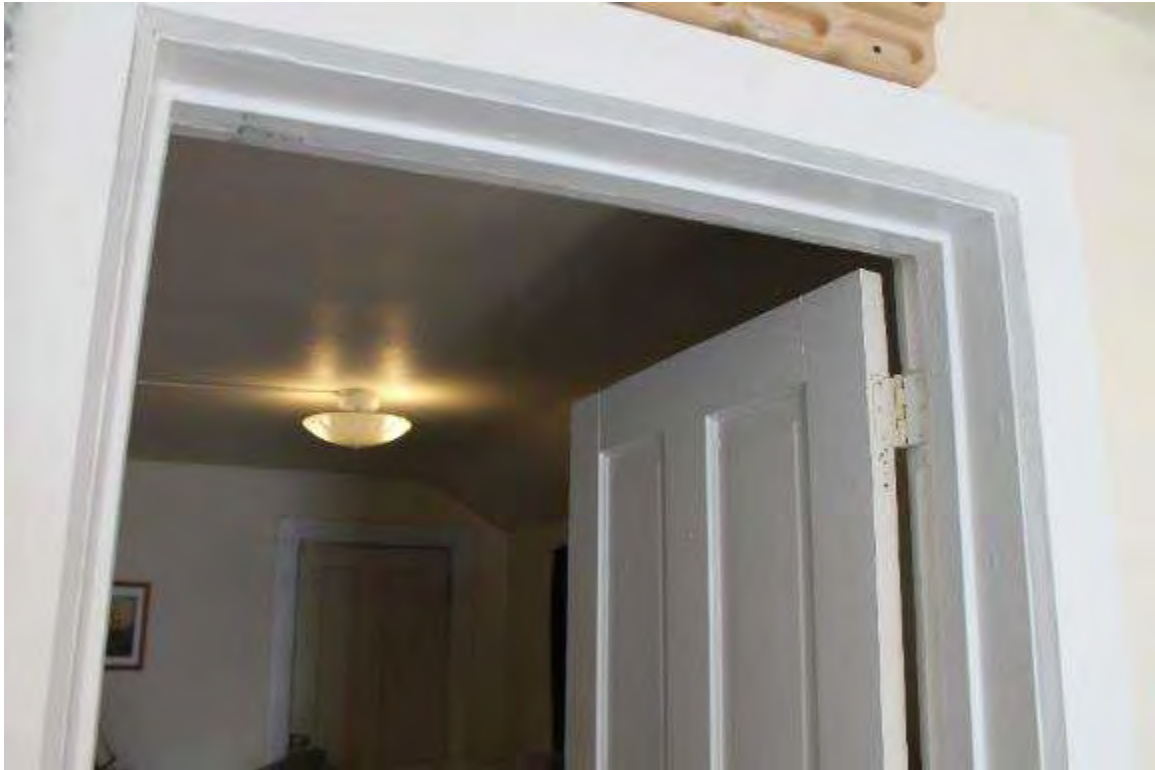
Photo 322: 410 1/2 East Washington Avenue, Interior, second floor unit 2
