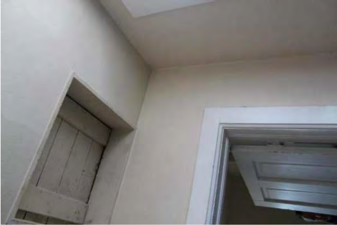
Photo 197: 402-408 East Washington Avenue, Interior, second floor unit 3
