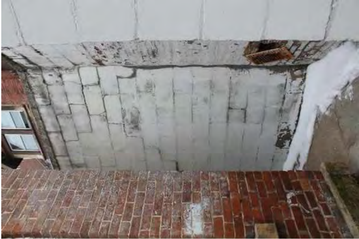
Photo 159: 402-408 East Washington Avenue, Exterior, facing northeast
