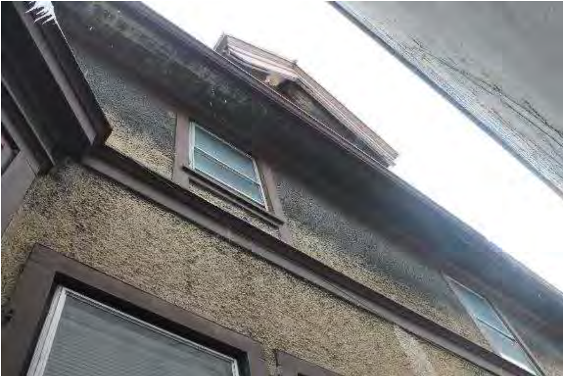
Photo 240: 410 East Washington Avenue, Exterior, facing west
