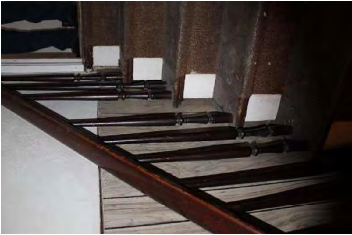
Photo 208: 402-408 East Washington Avenue, Interior, second floor stairs
