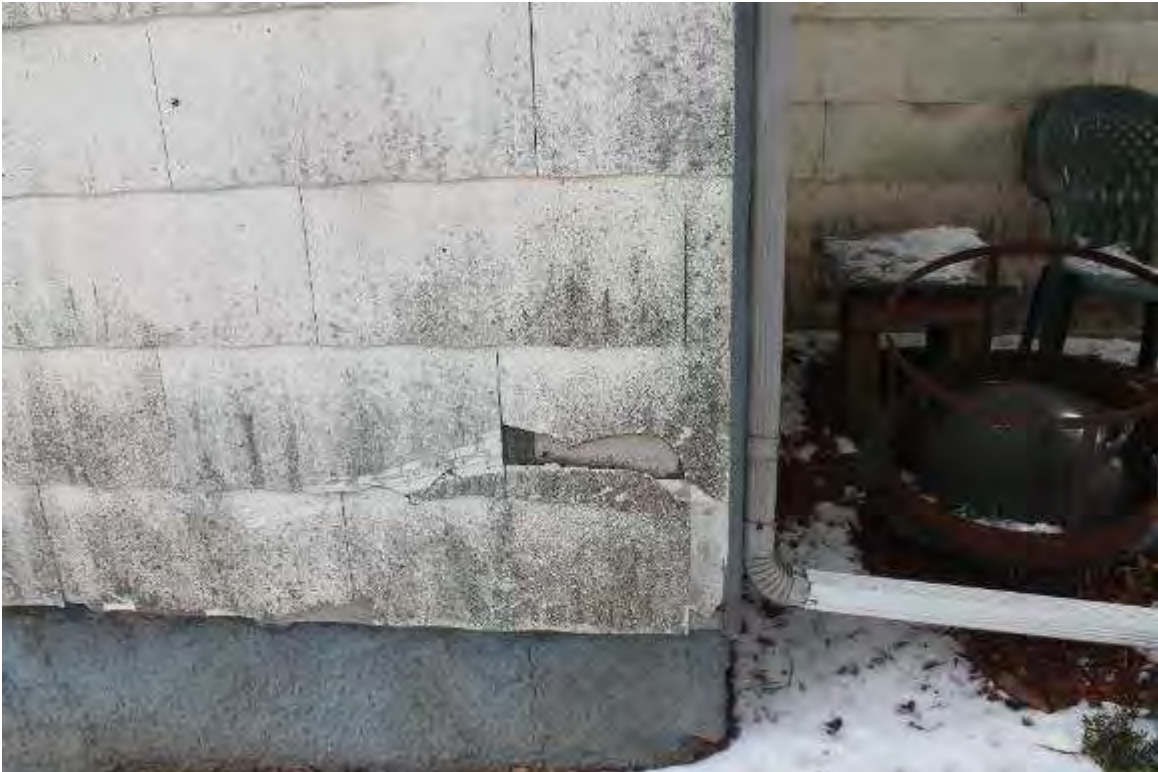
Photo 62: 8-10 North Franklin Street, Exterior, facing southeast
