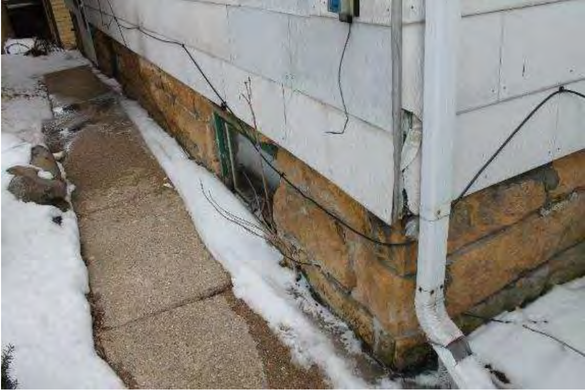
Photo 11: 9 North Hancock Street, Exterior, facing east
