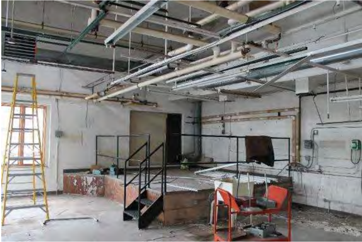
Photo 351: 412-414 East Washington Avenue, Interior, first floor processing space
