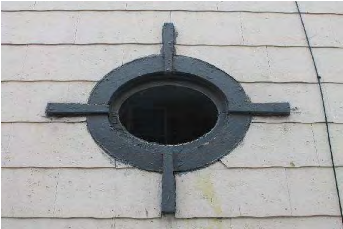
Photo 64: 8-10 North Franklin Street, Exterior, facing southeast
