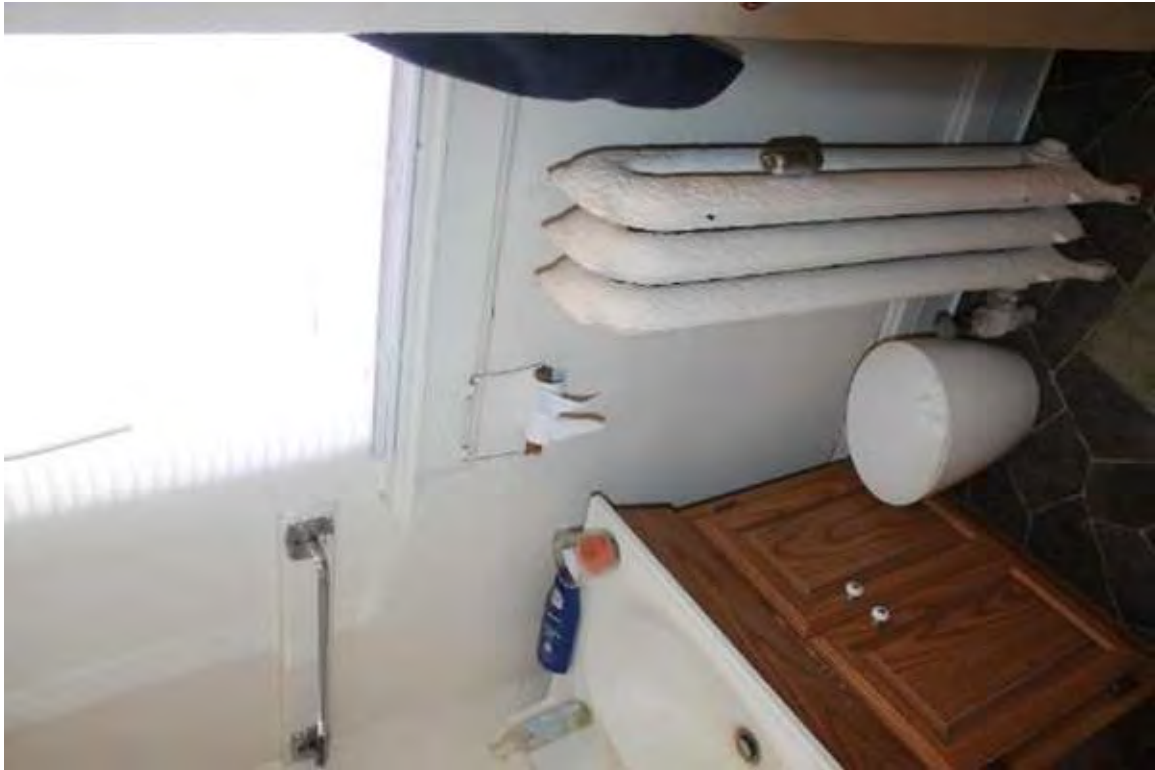
Photo 216: 402-408 East Washington Avenue, Interior, second floor unit 4
