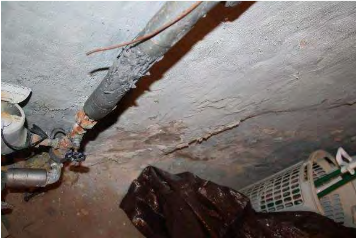
Photo 292: 410 East Washington Avenue, Interior, basement
