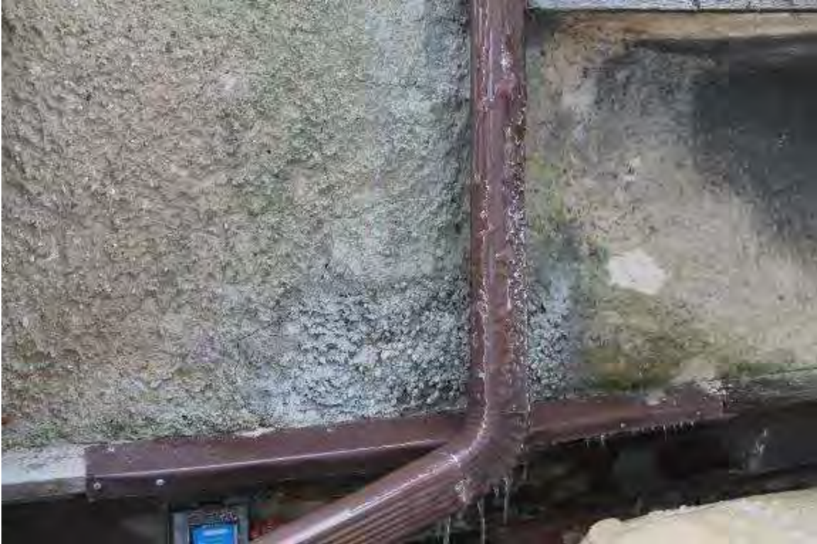
Photo 239: 410 East Washington Avenue, Exterior, facing west
