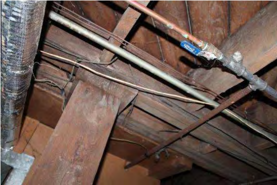
Photo 294: 410 East Washington Avenue, Interior, basement
