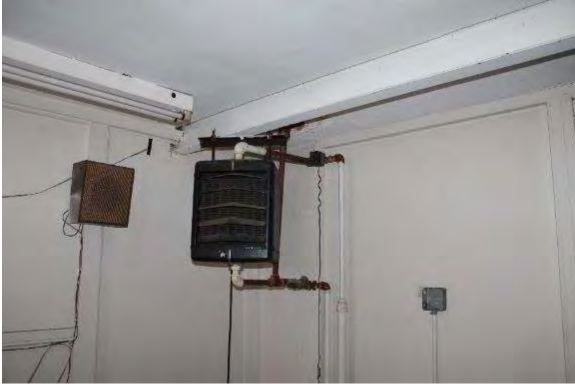
Photo 359: 412-414 East Washington Avenue, Interior, first floor mezzanine space
