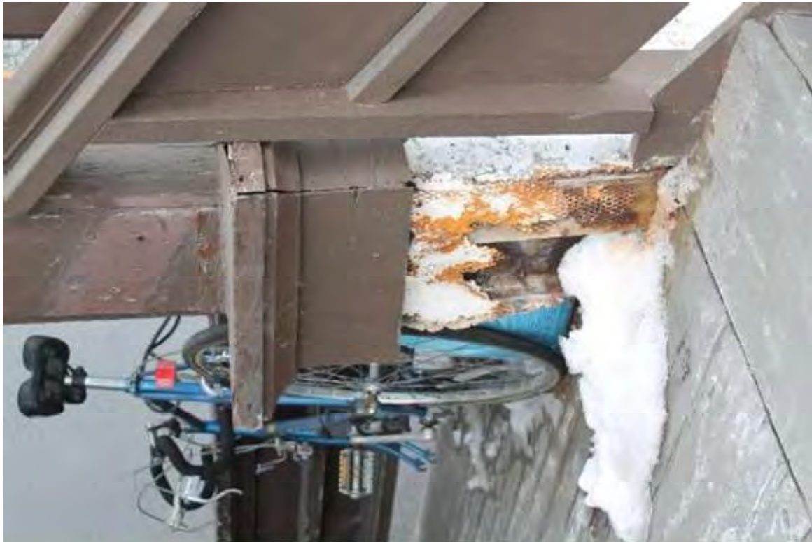
Photo 234: 410 East Washington Avenue, Exterior, facing north
