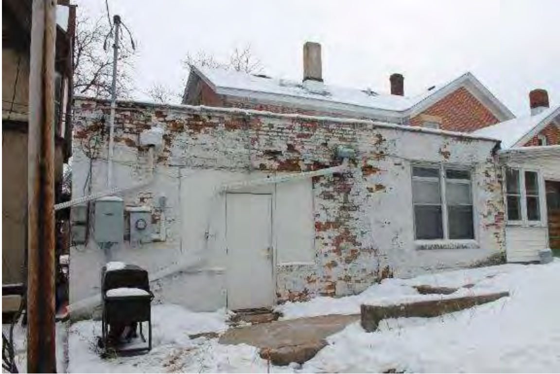
Photo 149: 402-408 East Washington Avenue, Exterior, facing south
