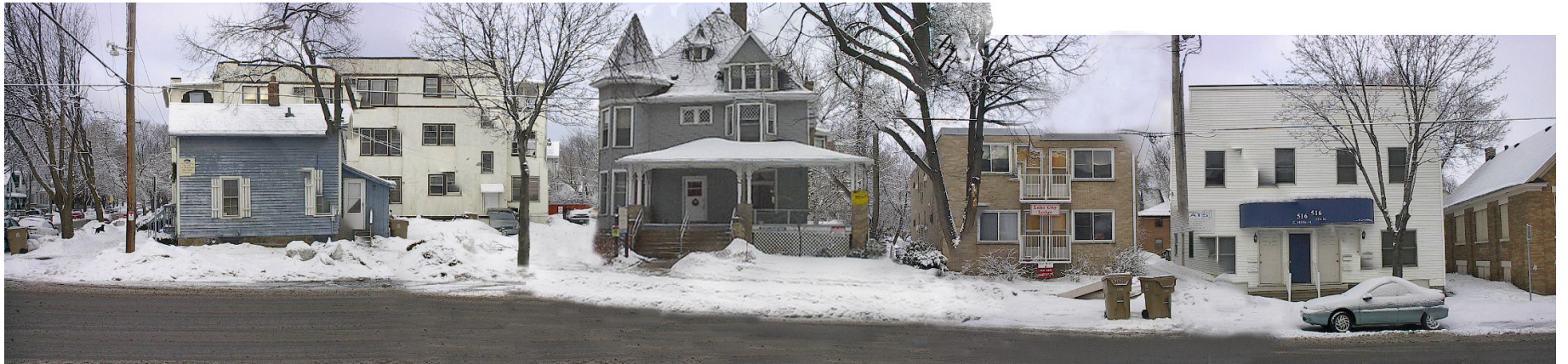
Conklin House at N. Franklin St. Site Elevation along E. Mifflin Street
