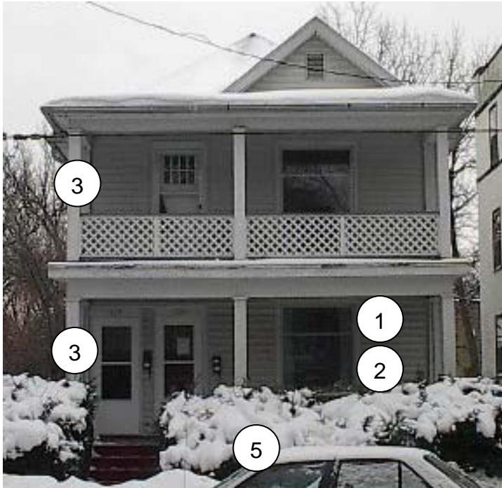
Southwest Elevation (Front)
