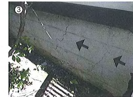
3 Repair cracked foundation
