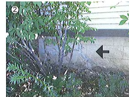
2 Repair cracked foundation
