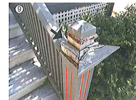
9 Repair/replace column trim
