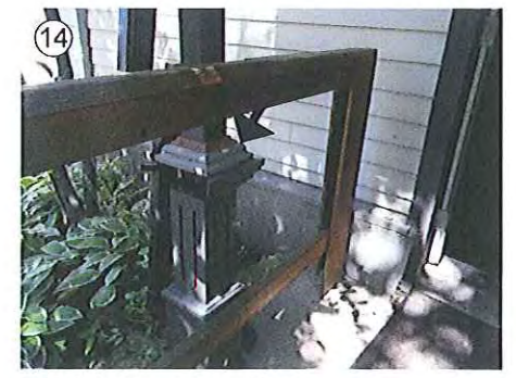
14 Repair/replace column trim
