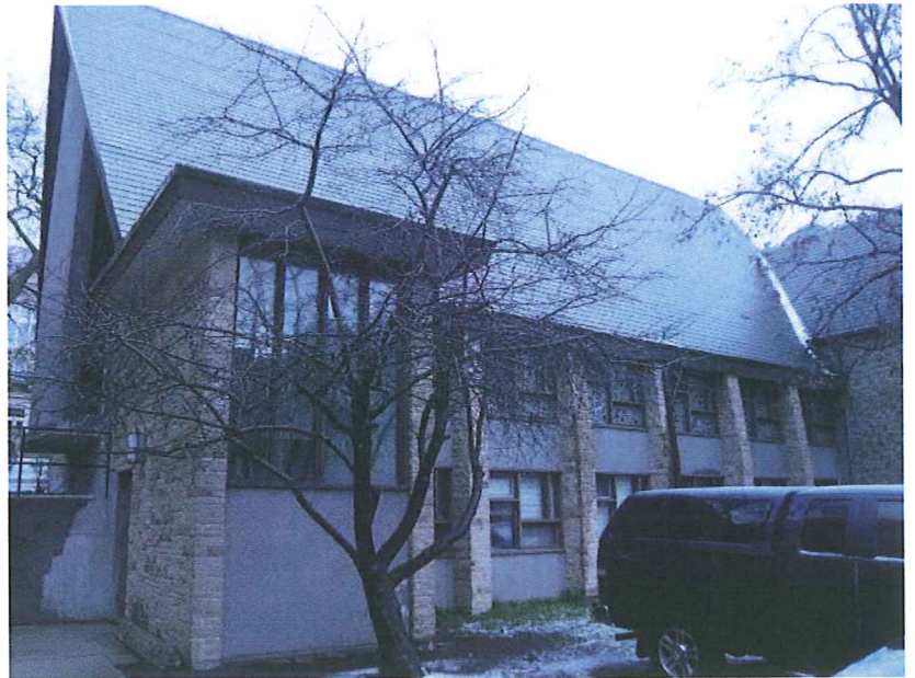
South Elevation-From Conklin Place
