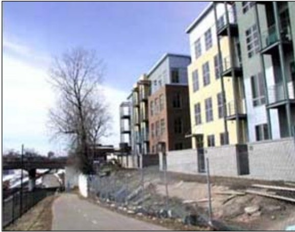
■ Balconies overlooking a path to increase safety.
