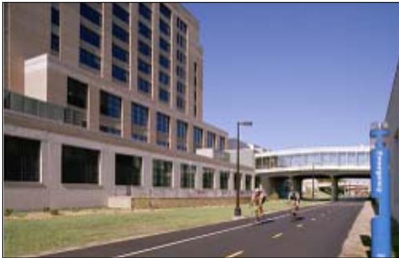
■ Building step-backs and emergency kiosks; Minneapolis Midtown Greenway.
