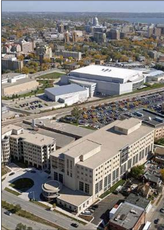
■ New UW Visitor's Center and parking structure at 21 N. Park Street.
