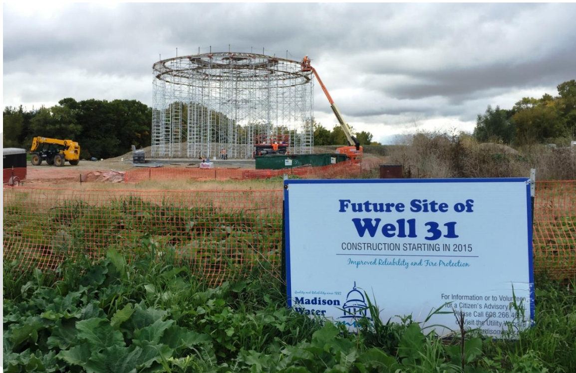
RESERVOIR CONSTRUCTION AT WELL 31 SITE, OCTOBER 2015
