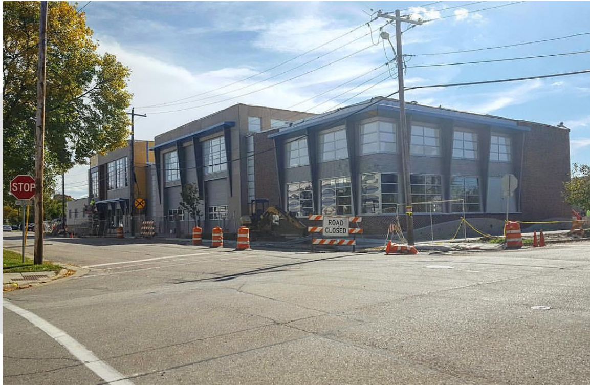
CONSTRUCTION OF NEW PATERSON STREET OPERATIONS CENTER, OCTOBER 2016
