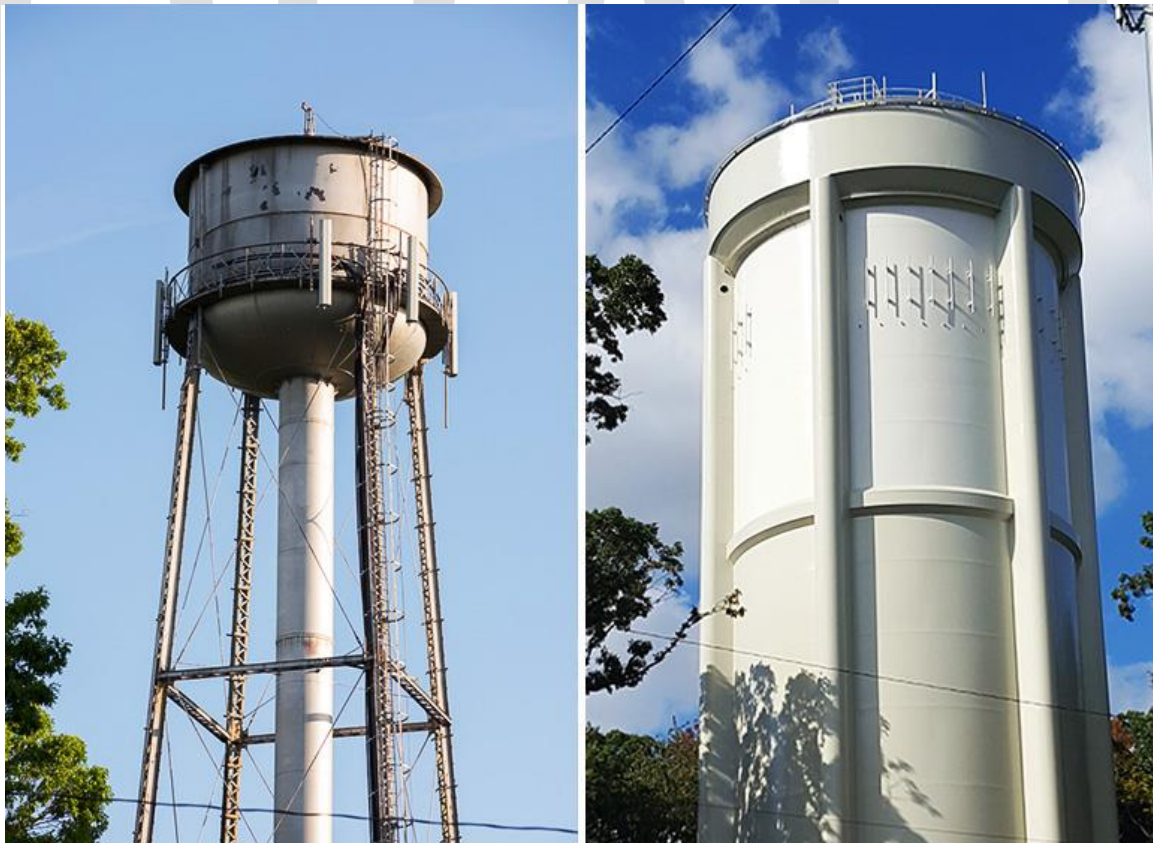
LAKEVIEW WATER RESERVOIR BEFORE AND AFTER
