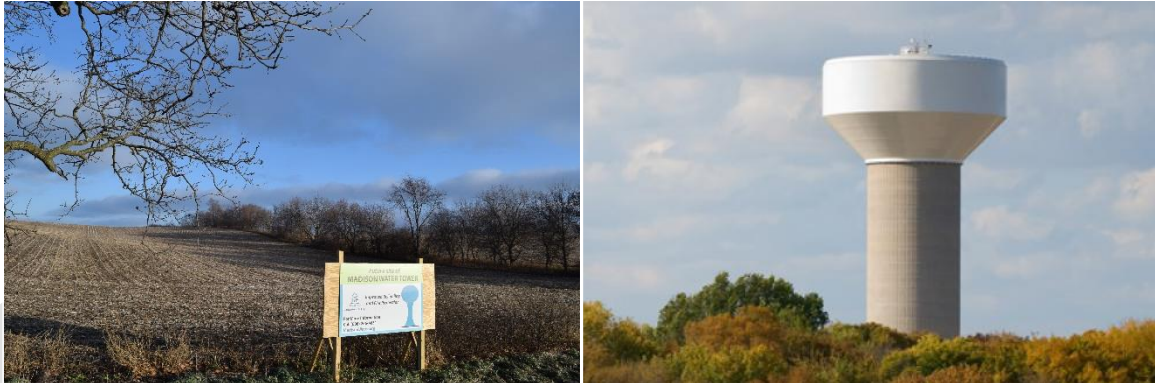
(LEFT TO RIGHT): BLACKHAWK WATER TOWER SITE, AND A SAMPLE PHOTO OF A COMPOSITE WATER TOWER
