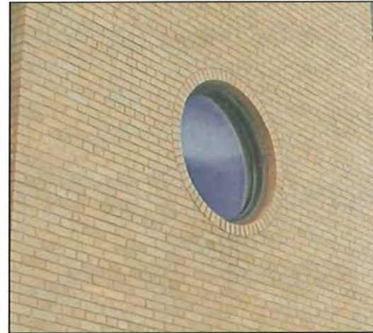
3 References to Architecture of 1940's Building NTS
