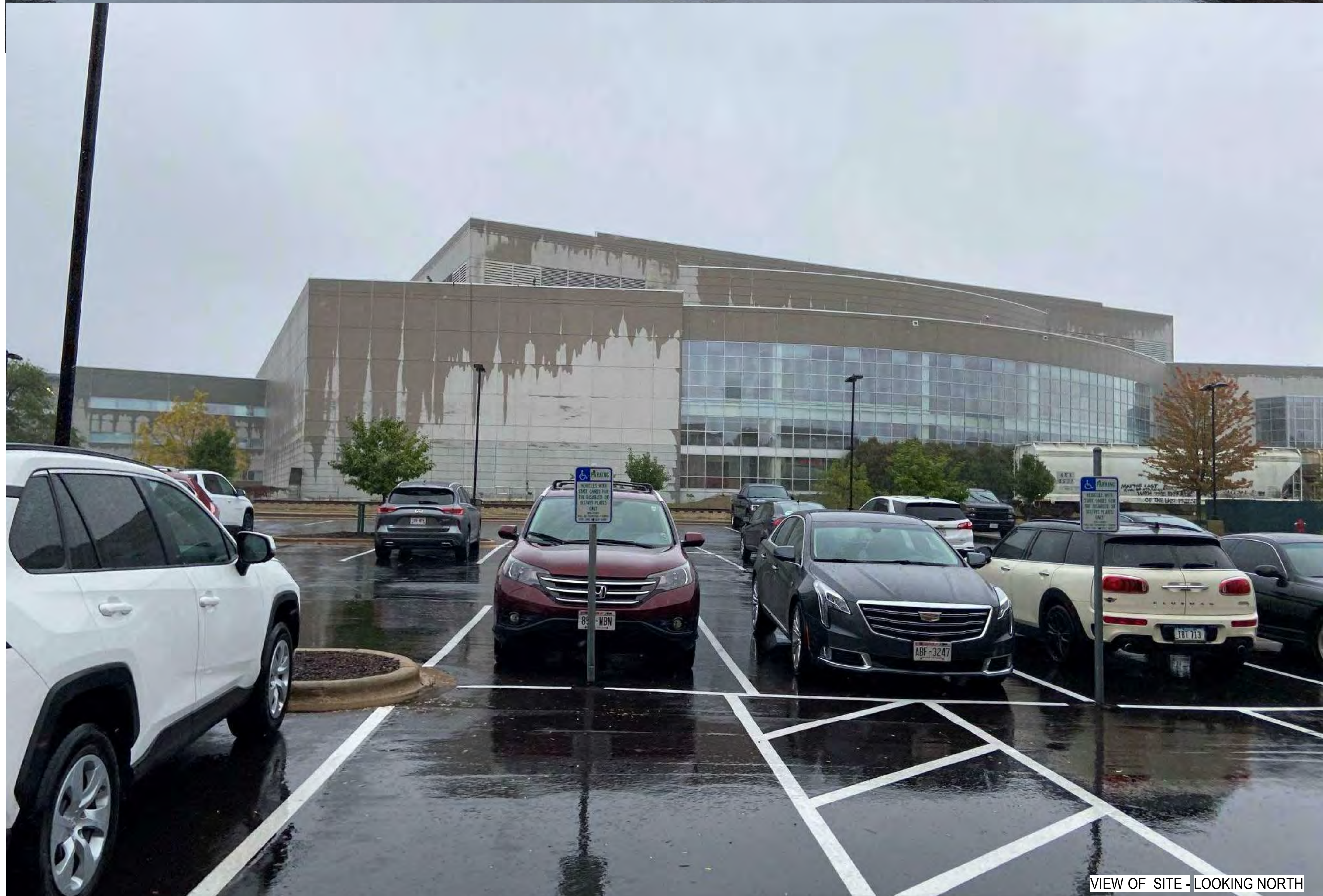
VIEW OF SITE - LOOKING EAST
