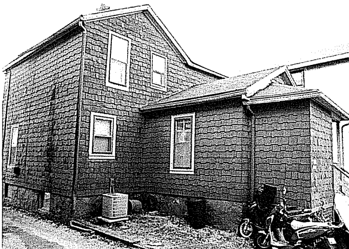
531 Mifflin existing building- from south
