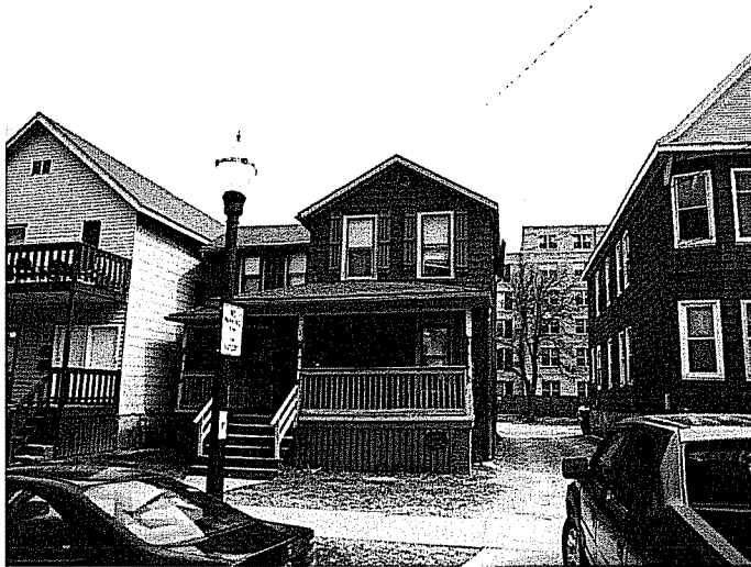
531 Mifflin existing building- street condition
