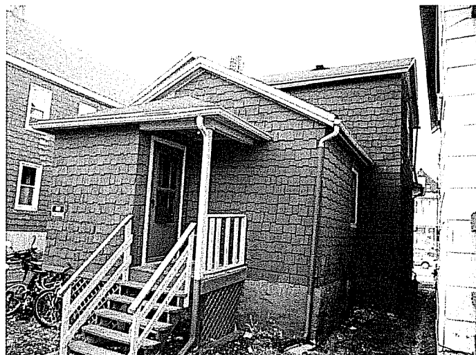
531 Mifflin existing building- from southeast
