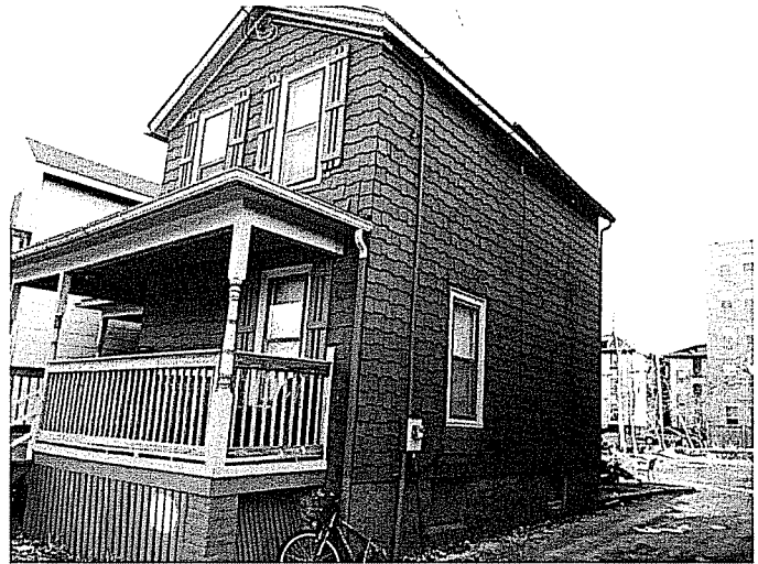
531 Mifflin existing building- from west
