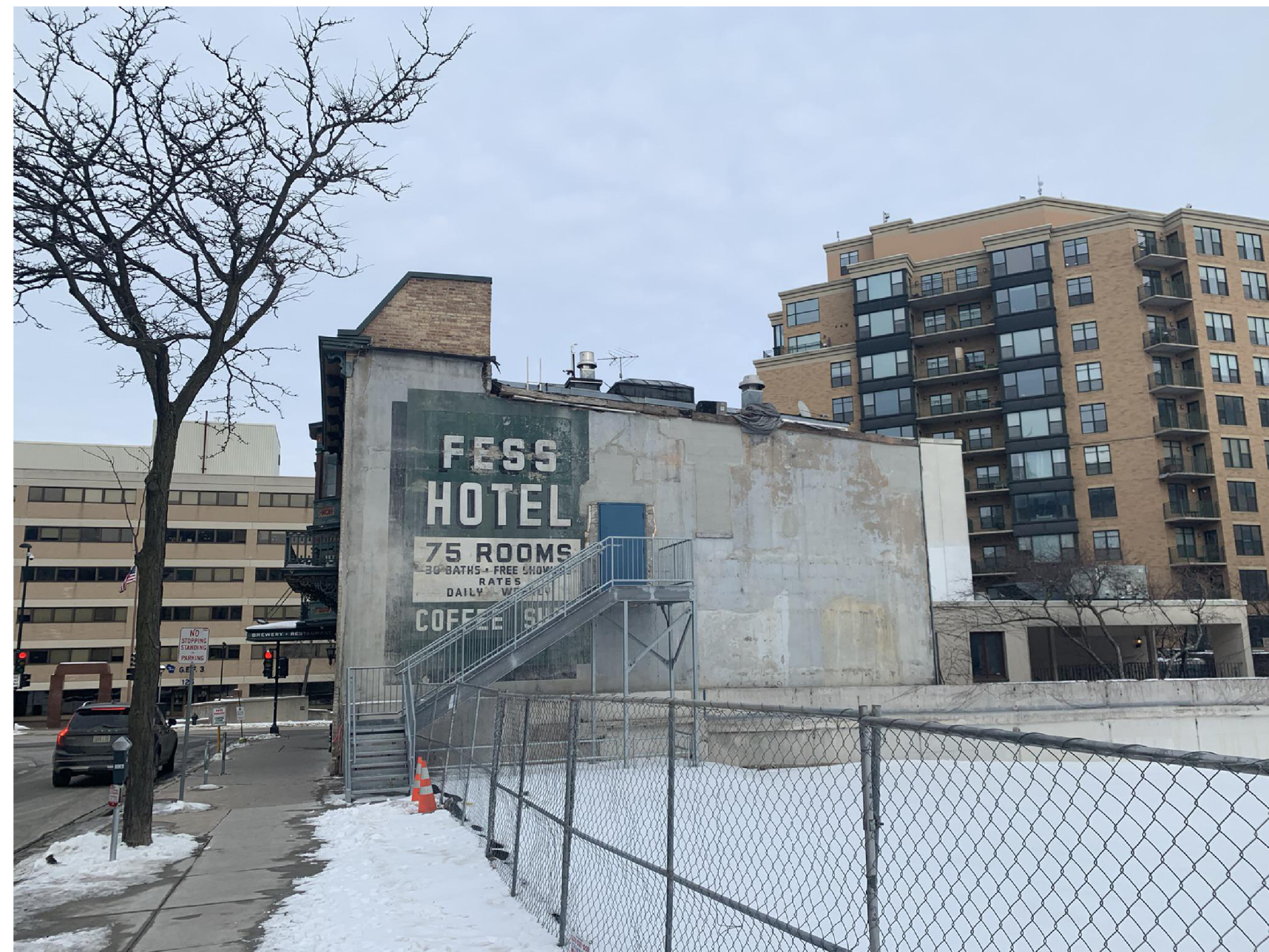
EXISTING CONDITIONS - SOUTHWEST WALL
