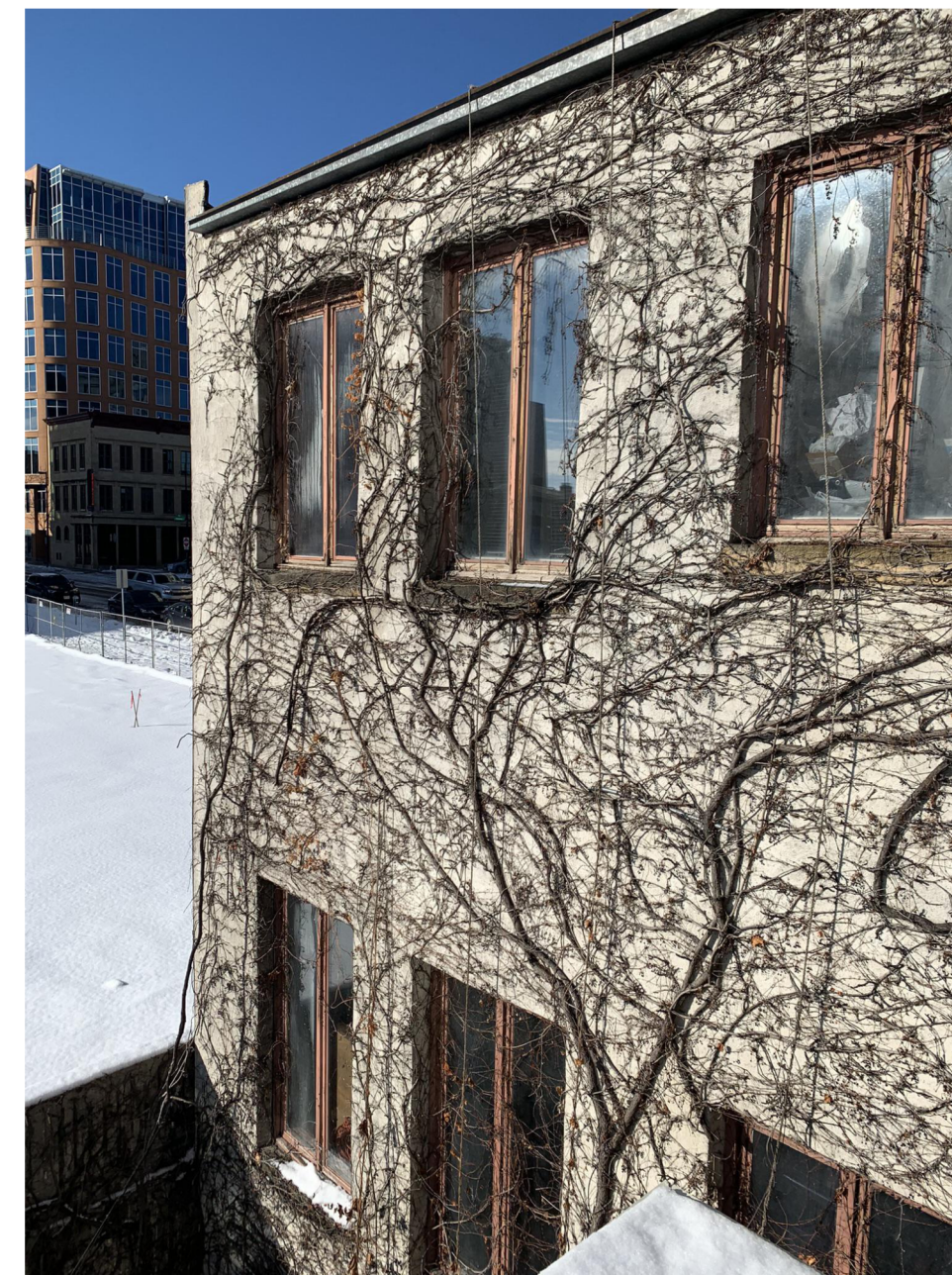
EXISTING CONDITIONS - SOUTHEAST WALL
