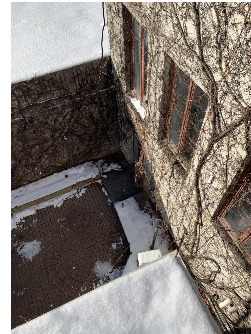
EXISTING CONDITIONS - SOUTHEAST WALL
