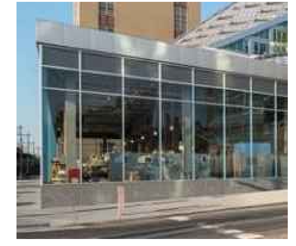
1" - INSULATED, LOW-E GLAZING & BIRD GLAZING ELEVATION KEYNOTES 5 & 6
