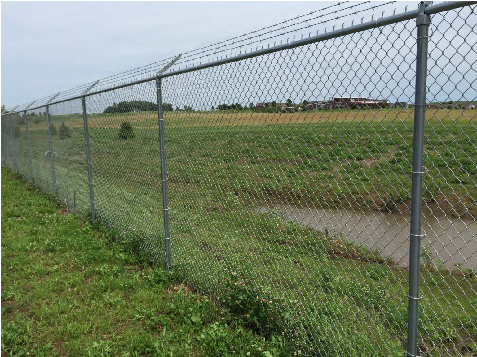
South Point Yard M-2 : East Stormwater Treatment
