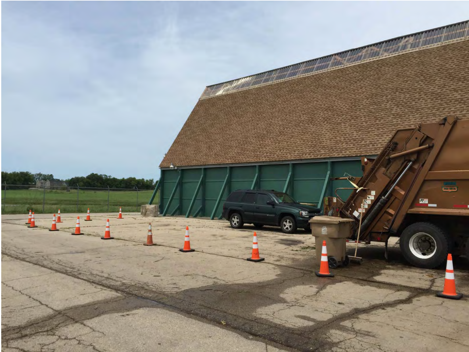
South Point Yard M-1 : Vehicle Storage Building
