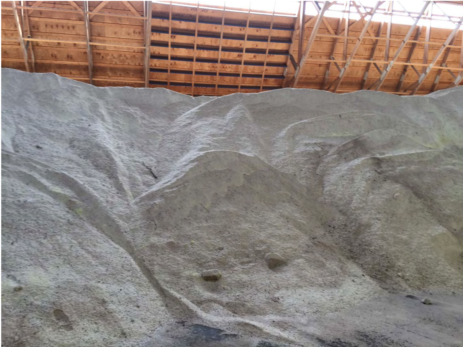
South Point Yard B2-1 : Salt Storage
